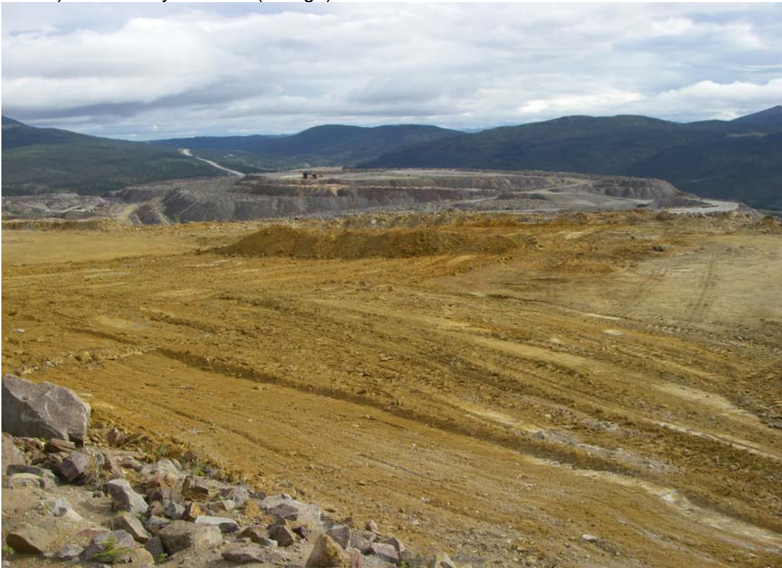
Photo 8: Footprint of S/P2 after leveling with the dozer, after all the above grade material was removed. The pile visible in the photo contains contaminated subgrade material waiting to be hauled away.
