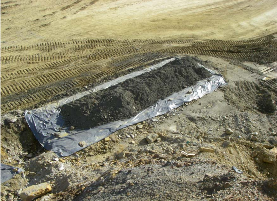
Photo 17: Grey waste placed on the liner of Test Pad 2.
