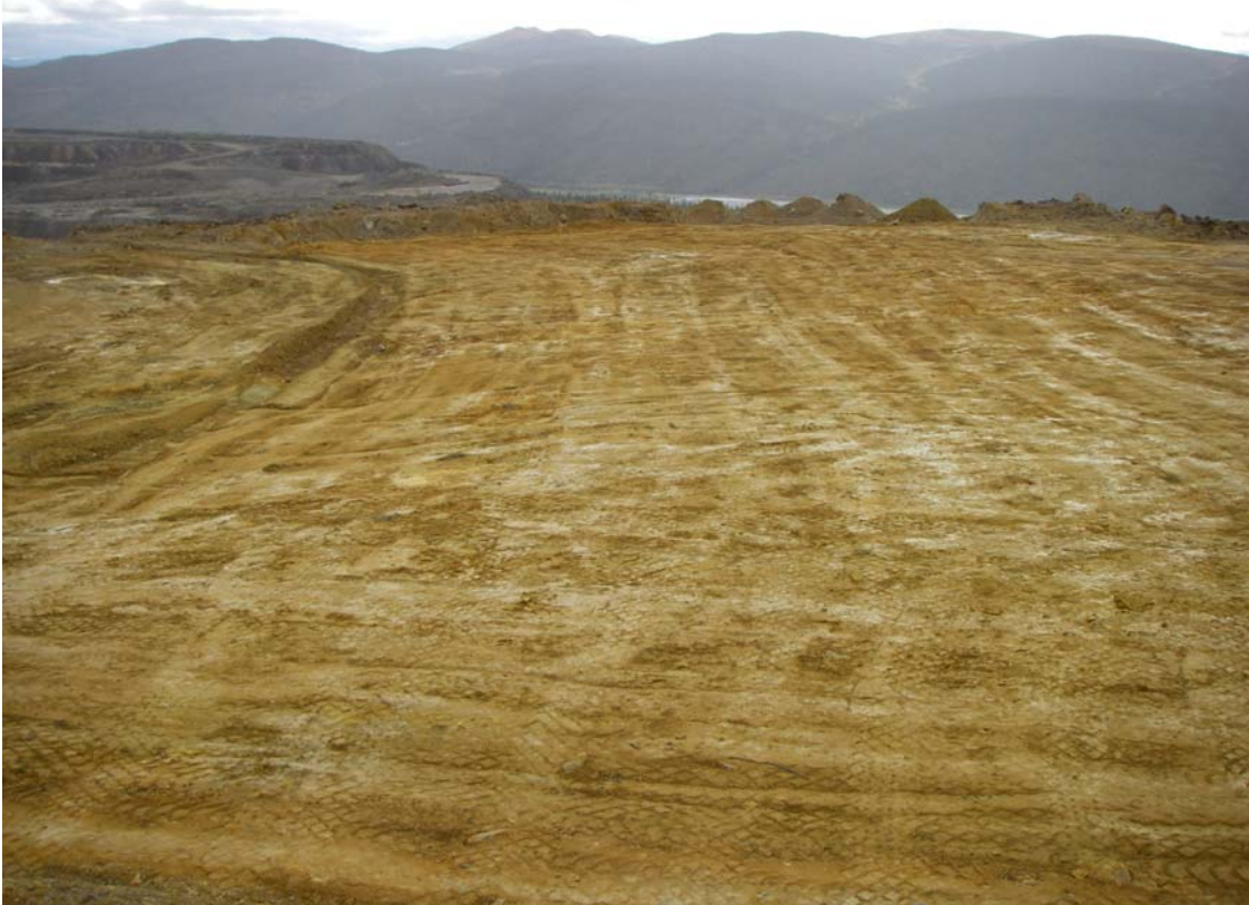
Photo 9: Footprint of S/P2 after grading and compaction. Drainage ditch noticeable in the upper left corner of picture.
