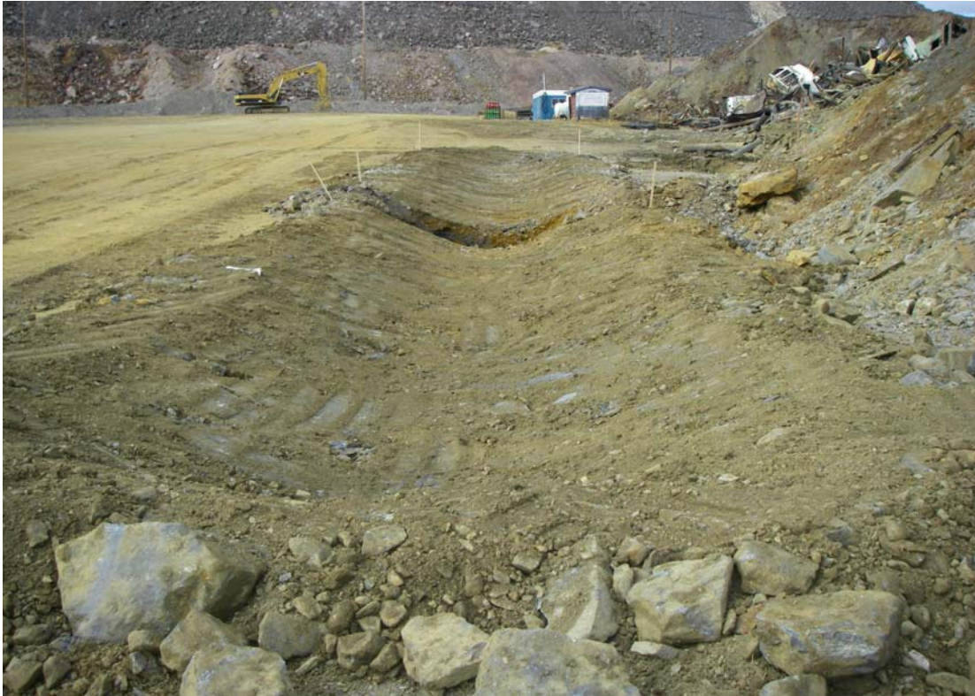
Photo 15: Test Pad 2 (in background) and 3 in foreground after excavation, prepared for the placing of the PVC liner. Collection point between the two test pads.
