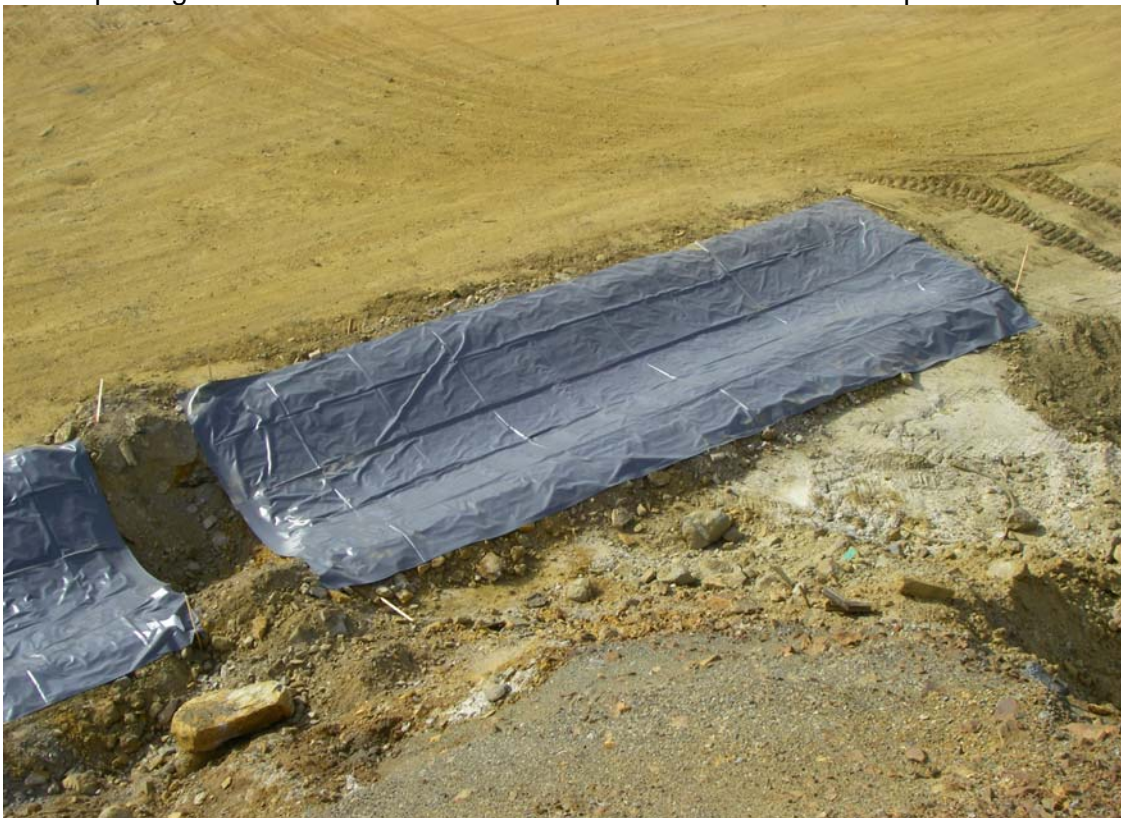
Photo 16: PVC liner placed on Test Pads 2 (right side) and 3 (left side).
