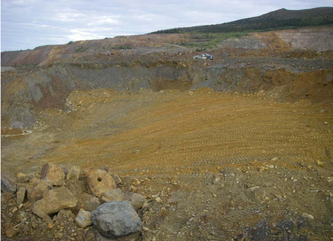
Photo 5: Finished waste repository at LGSP'C'. Drainage ditch and test pad 3 visible at the left side of the photo.
