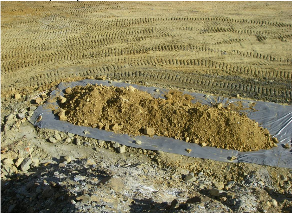
Photo 18: Orange waste placed on the liner of Test Pad 3.
