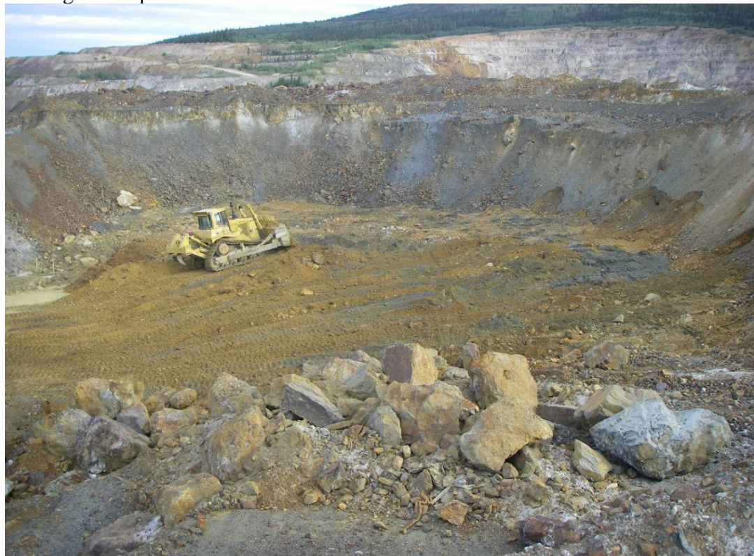
Photo 4: Dozer pushing up and levelling the hauled waste at LGSP‘C’ on day 6.
