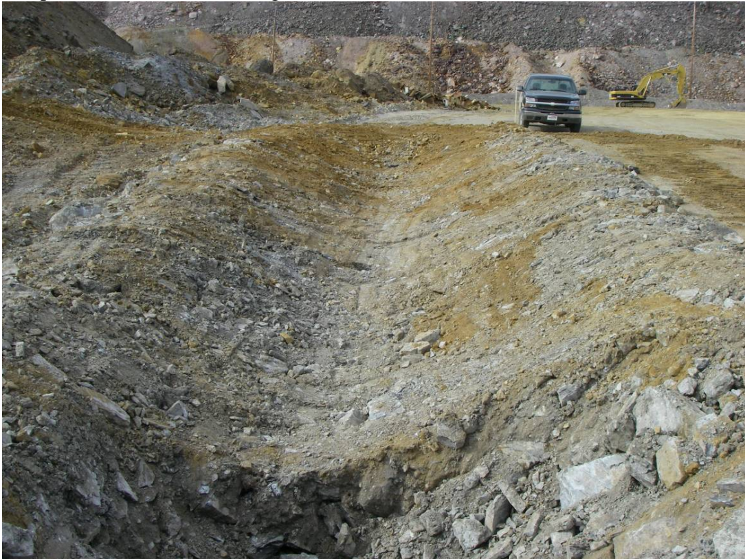
Photo 12: Test Pad 1 with the collection point in the foreground.
