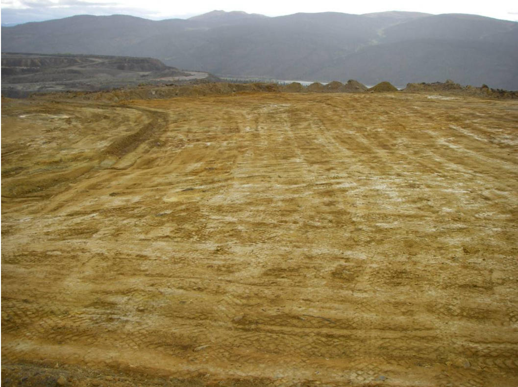
Photo 9: Footprint of S/P2 after grading and compaction. Drainage ditch noticeable in the upper left corner of picture.
