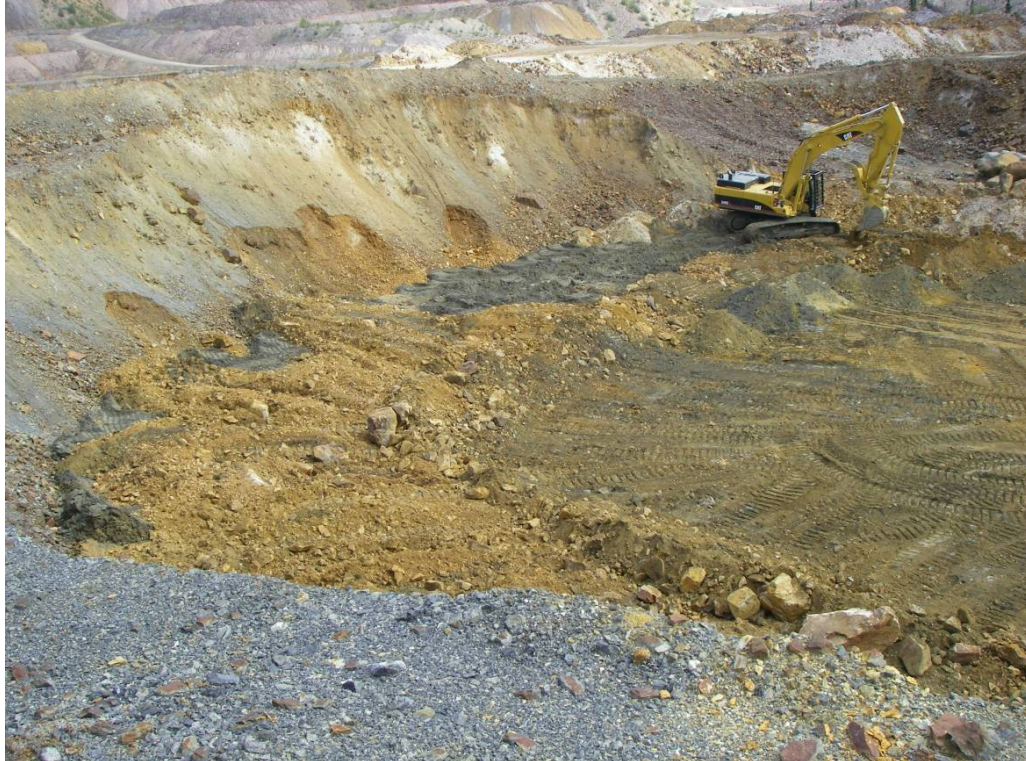
Photo 2: Waste repository at LGSP 'C' – the soft fines from S/P2 on the far side of the photo (grey colour) placed against the original topography of LGSP 'C' and the dry, rocky material from S/P3 placed downstream (orange colour) at the end of day 3 of the program.
