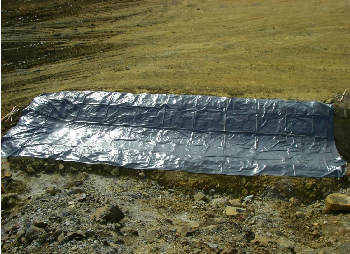
Photo 13: PVC liner placed on Test Pad 1. The drainage point is located in the right side of the photo.
