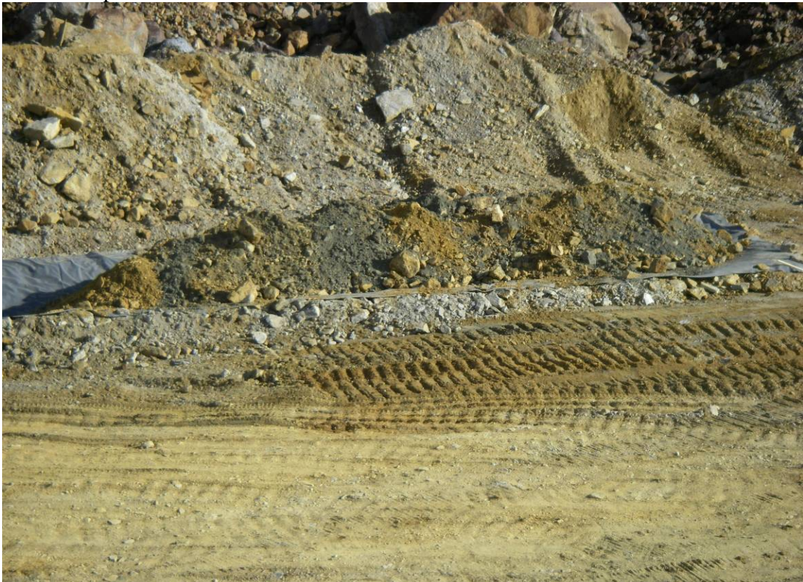
Photo 14: Mixed waste (gray and orange) placed on the liner of Test Pad 1.
