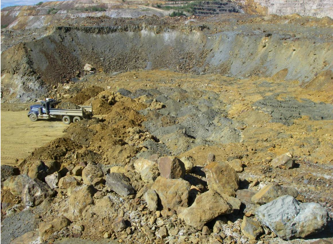
Photo 3: Relocated waste rock from S/P2 “bubble dumped” at the repository site on day 5. Material hauled on previous days pushed up and levelled in a bench against the original slope of LGSP‘C’.
