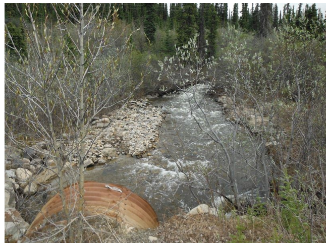
Photo 12. South Fork Rose Creek downstream of Haul Road but upstream of Mine Access Road ( GCULV ), looking upstream from culvert.
