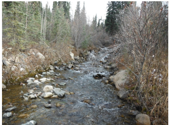
Photo 20. Reservoir Creek upstream of Mine Access Road ( K8 ), view looking upstream of culvert from sampling location.
