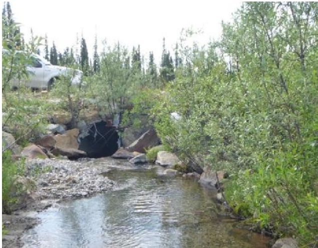
Photo 9. West Fork Vangorda Creek downstream of AEX Creek (VW3), looking downstream to auxiliary road culvert, July 22, 2015.
