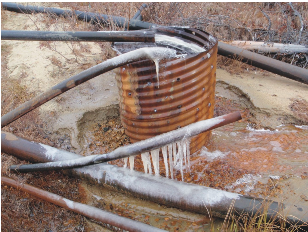
Photo 5: Outlet from seepage pond.
