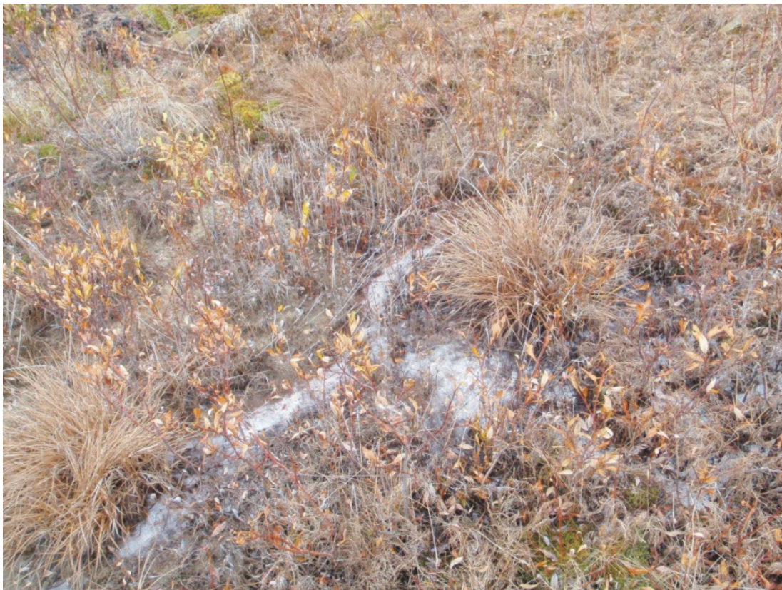
Photo 3: Frozen seep at base of seepage pond dam (See Figure 1).
