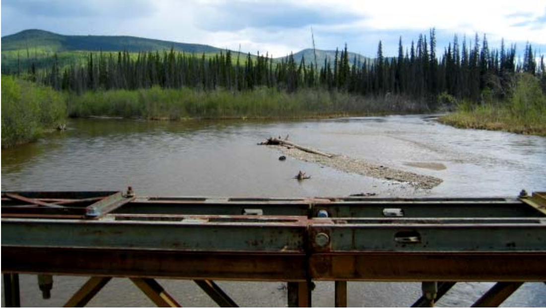
Photo 13: the confluence of the South McQuesten River (right) and Haggart Creek as seen from the Haggart Creek bridge in June, 2006.
