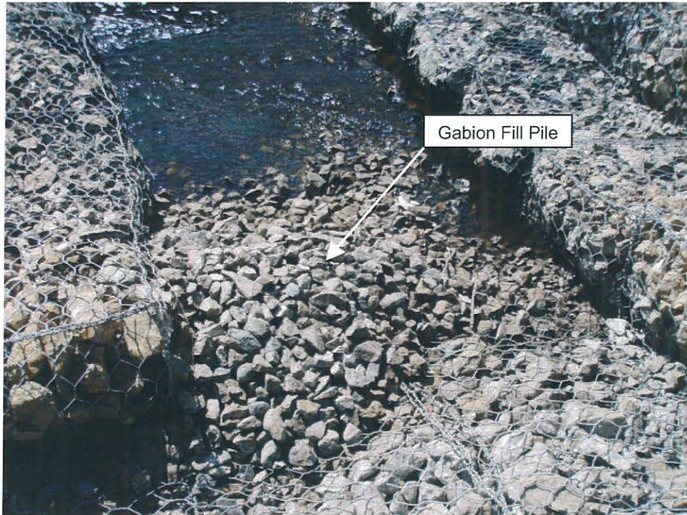
Figure 01: Remove deposit of gabion fill at outside corners of end sills.
