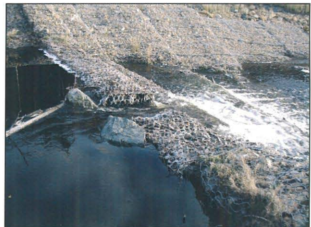
Figure 5.2 DS#1 – Compartment Removed from Drawdown Weir in 2007
