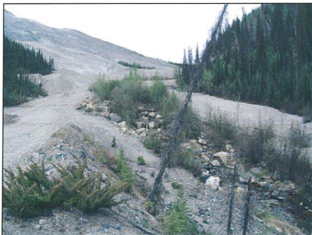
Figure 3.1 Vegetation Along Rock-Lined Channel
