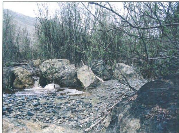
Figure 3.2 Sedimentation and Shifted Boulders In Rock-Lined Channel
