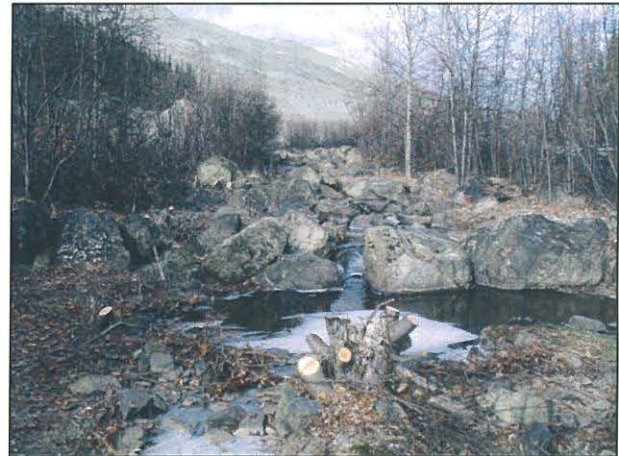
Figure 5.5 Trees Removed From Rock-lined Channel
