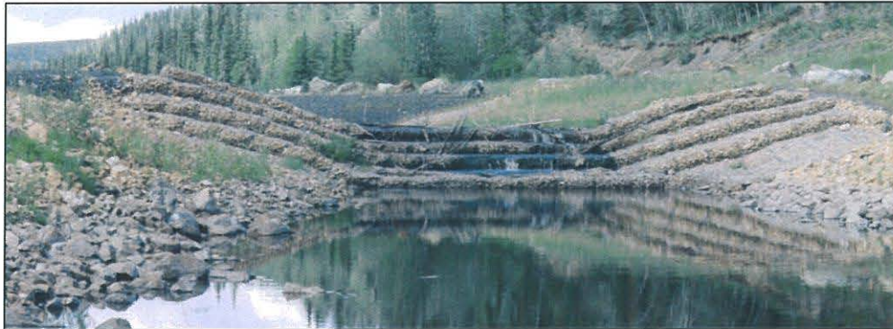
Figure 2.2 General Condition of Drop Structure #1
