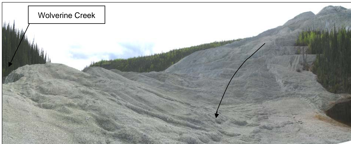
Figure 2-1) Mounding at Toe of South Lobe Near Monitor 2005-01 (view facing south)
