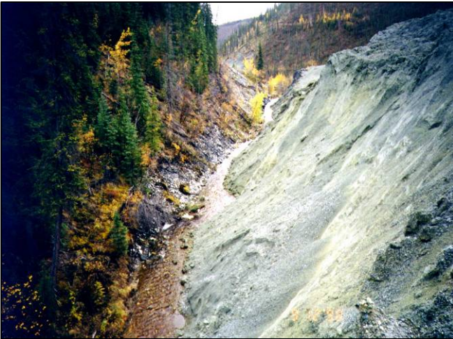
Figure 41 Toe of Tailings in 1998 (view D/S)
