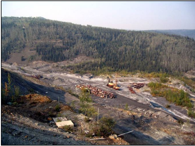
Figure 14 Crusher Building Demolition (2004)
