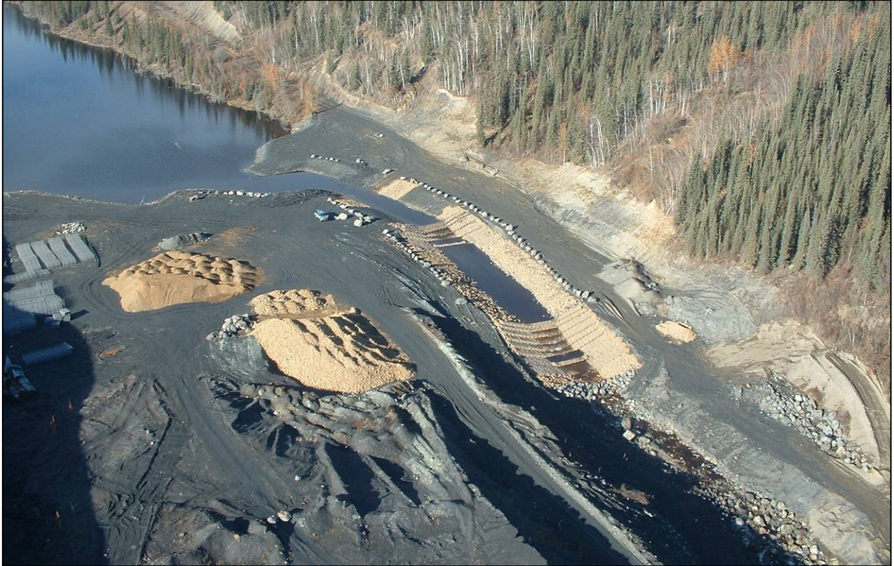
Figure 11 Completed Stage I and II Channel Stabilization Works (2003)
