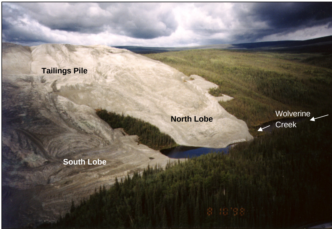
Figure 05 Wolverine Creek Tailings Pile (1998)
