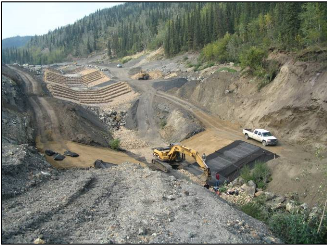
Figure 12 Construction of DS #4 (2004)
