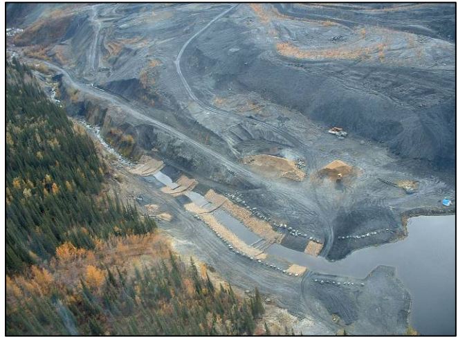
Figure 13 Completed Stabilization Works (2004)
