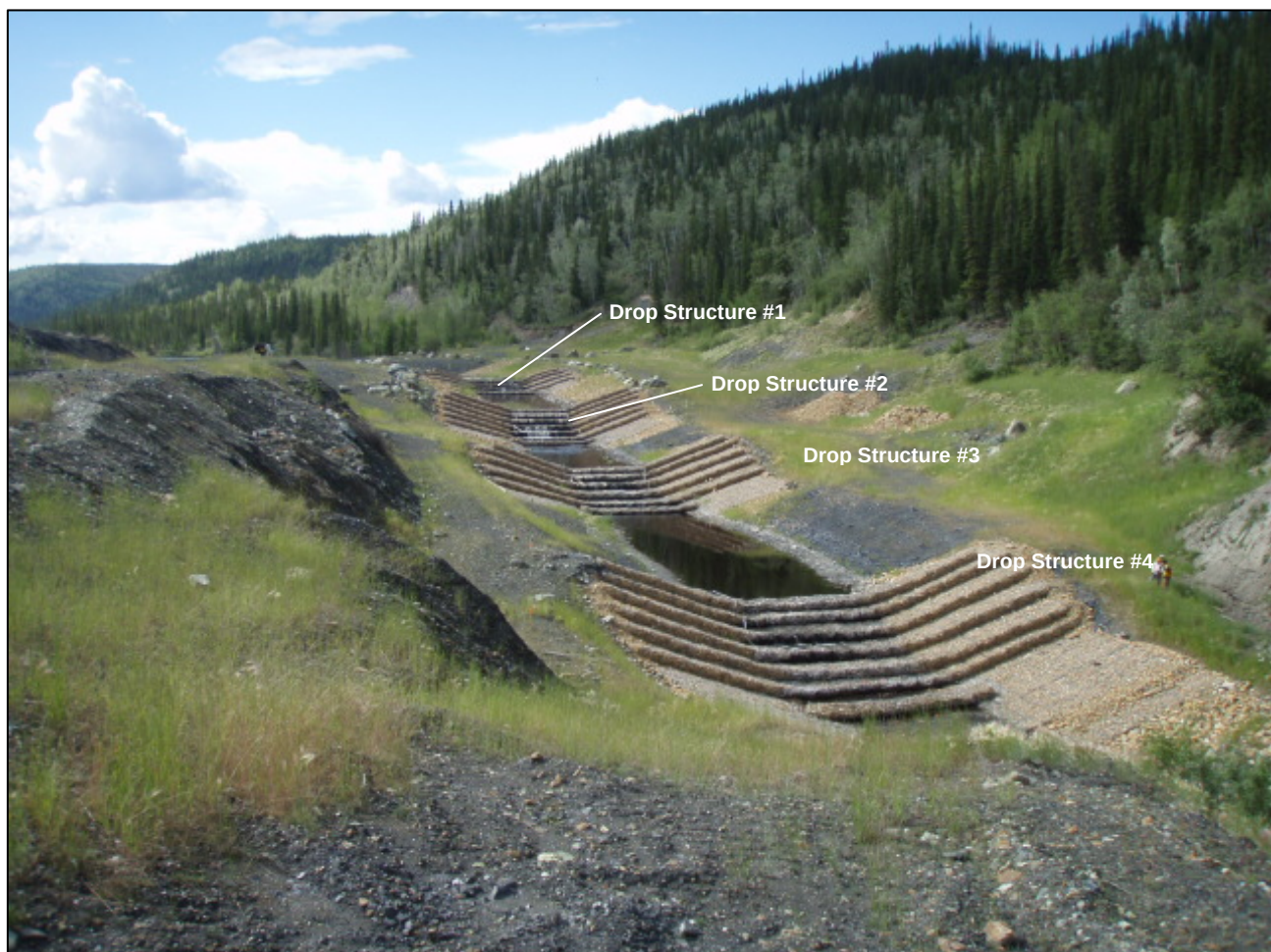
Figure 17 Stabilized Channel Section at Hudgeon Lake Outlet (2007)
