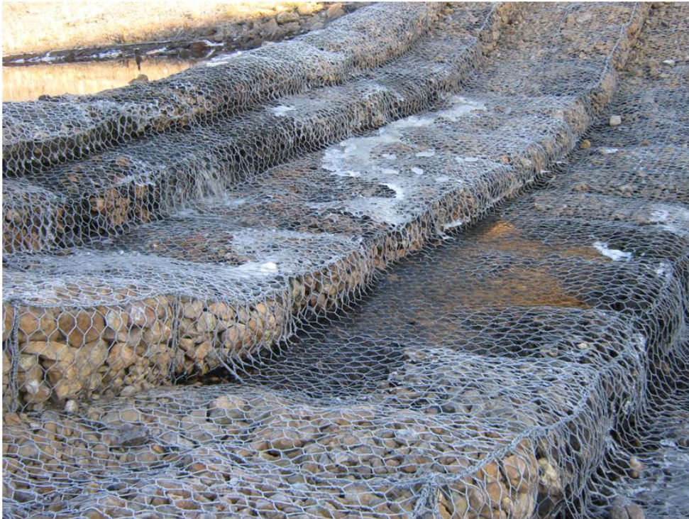
Photo 20: Drop Structure #4. Wire mesh placed overtop of existing gabions.
