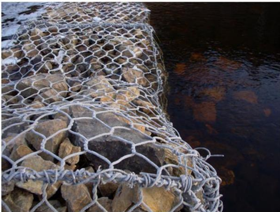
Photo 9: Drop Structure #2. Top of new 0.3 m end sill hand stitched closed.
