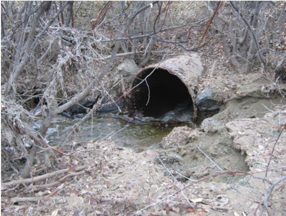
Photo 23: Wolverine Creek Road Crossing. Existing west culvert inlet cleared of debris.
