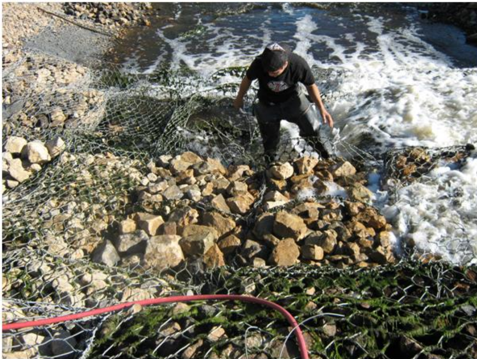
Photo 16: Drop Structure #4. Baskets being filled with large rock.
