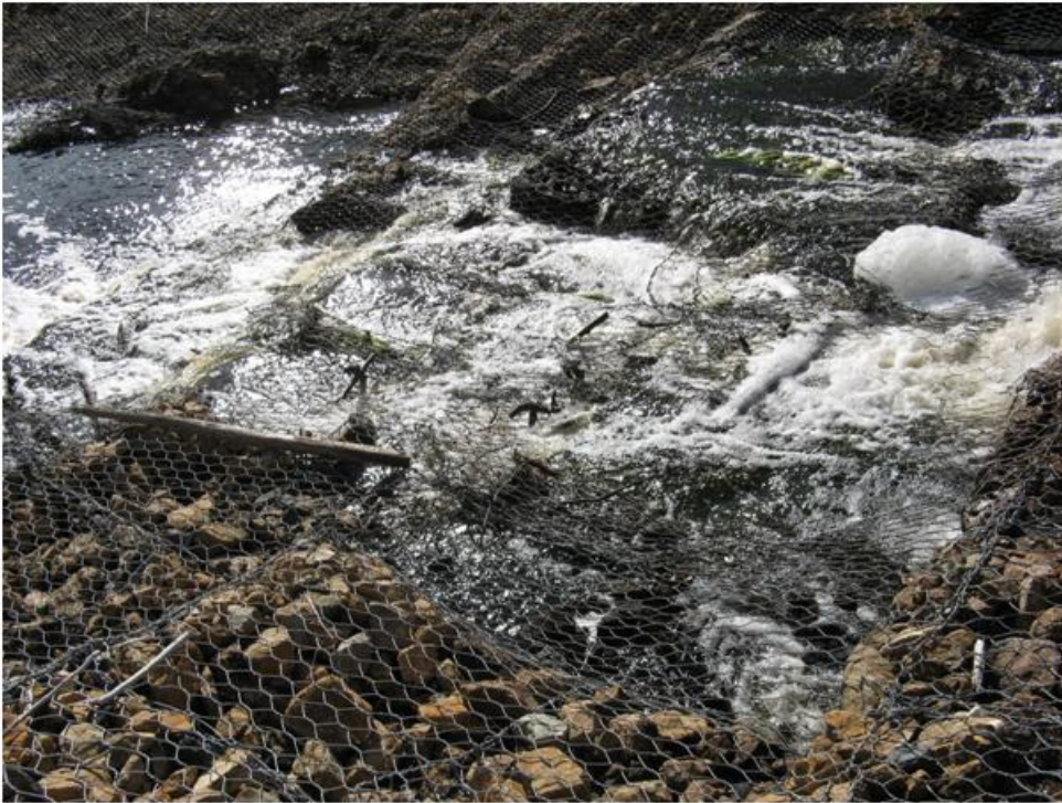
Photo 13: Drop Structure #4 prior to construction. Empty baskets along the bottom width.
