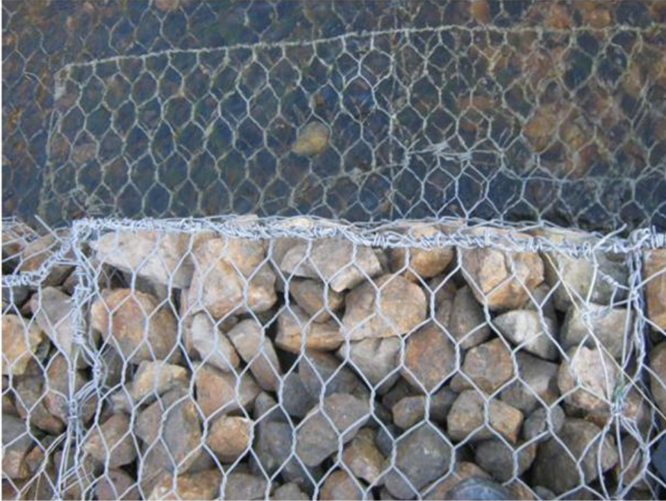
Photo 19: Drop Structure #4. Hand stitching at the downstream end of the structure.
