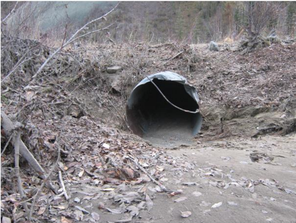
Photo 24: Wolverine Creek Road Crossing. Existing east culvert inlet cleared of debris.
