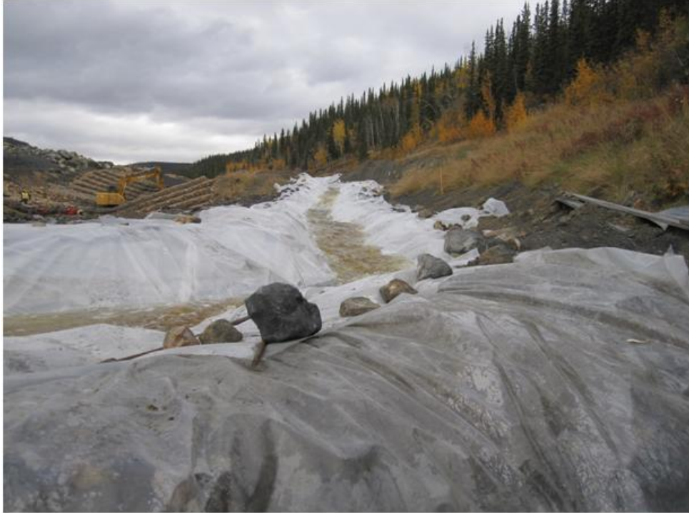
Photo 7. Diversion channel adjacent Drop Structure #4 looking upstream
