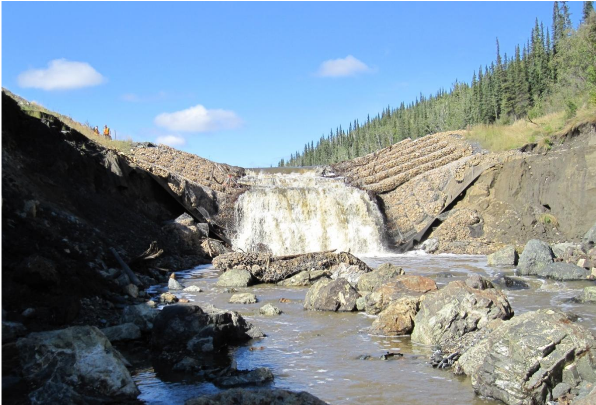
Figure 3: Looking Upstream at Drop Structure #4, August 19th, 2010
