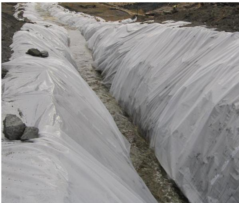
Photo 6. Diversion channel adjacent Drop Structure #2 looking downstream.
