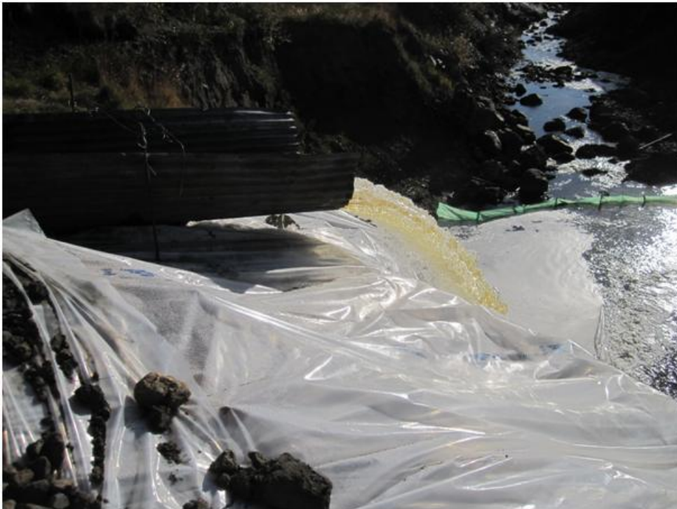
Photo 8. Outlet of the diversion channel at Drop Structure #4
