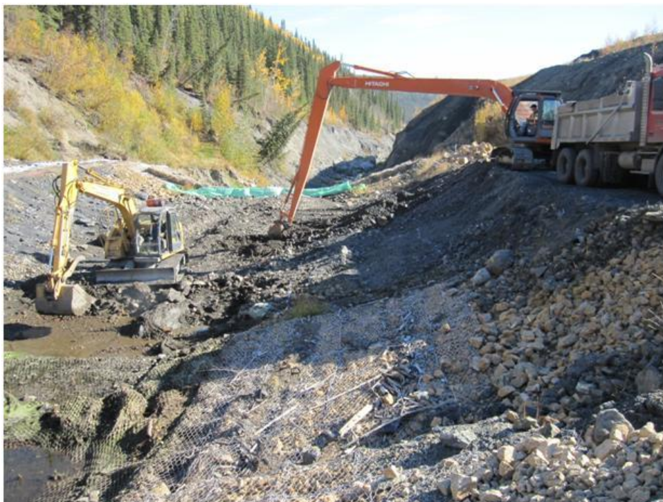
Photo 12. 135 Deere and 200 Hitachi excavators reshaping the channel downstream of Drop Structure #4.
