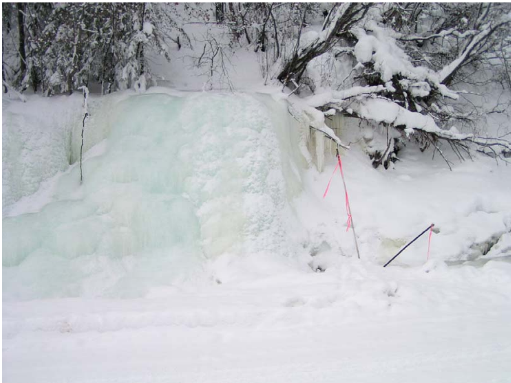
Culvert #5, Glacier. No Q through Hwy.
