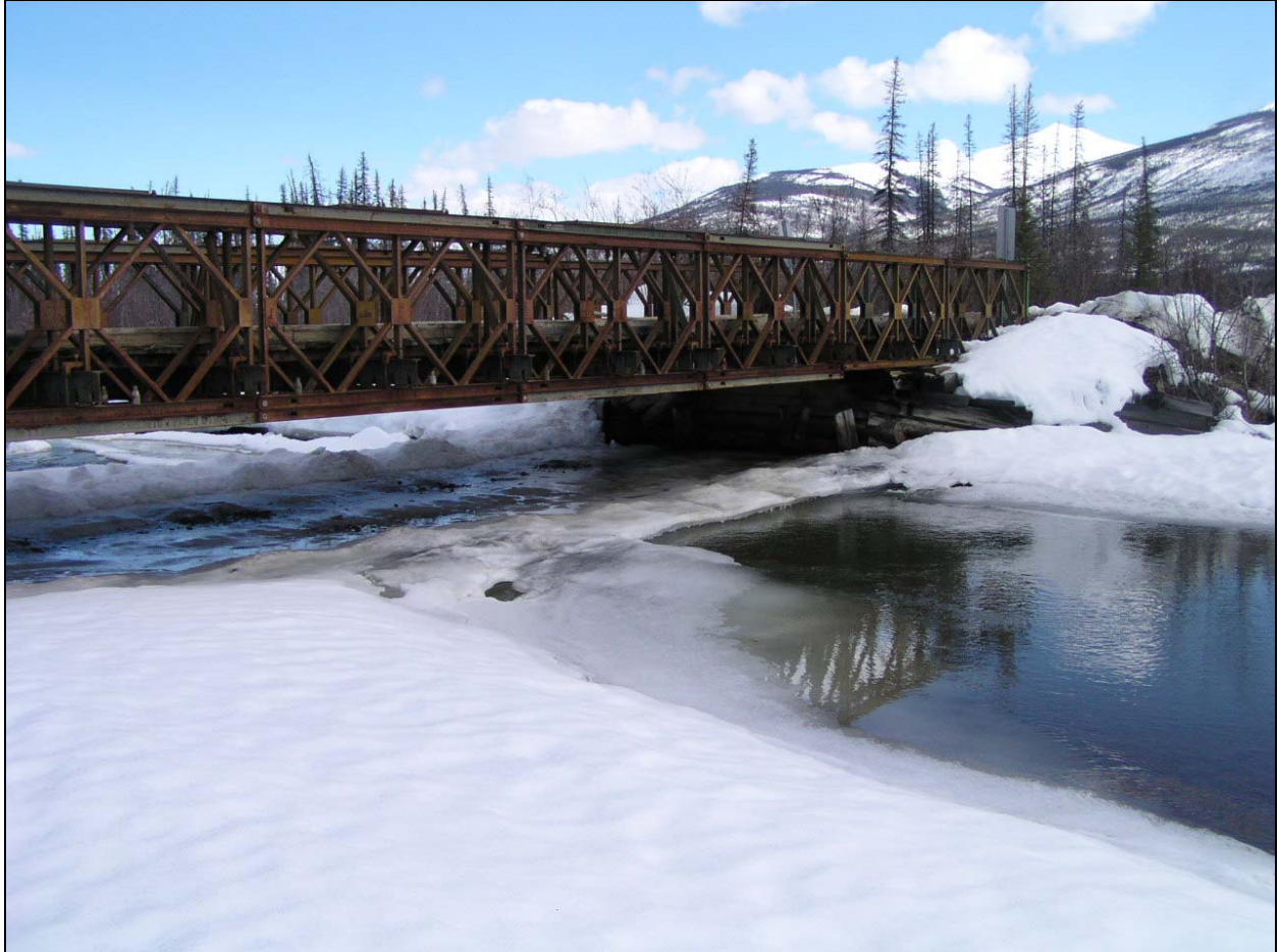
South McQuesten River at Haggart Creek Bridge.
