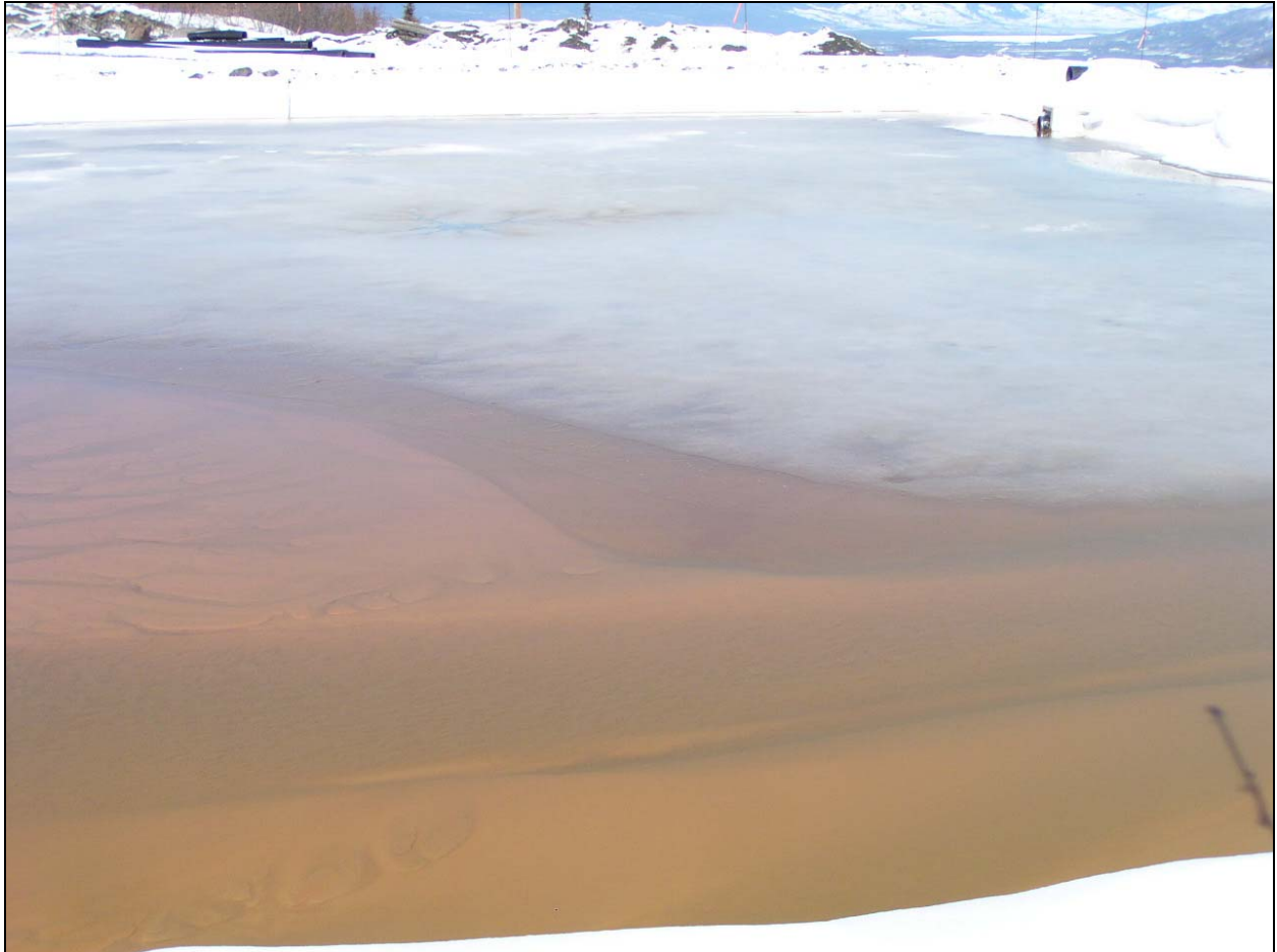
Galkeno 300 treatment pond. Note short circuiting and floating loose floc.
