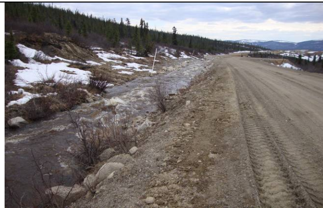
Photo 1: Upper portion of FCDC looking downstream.
