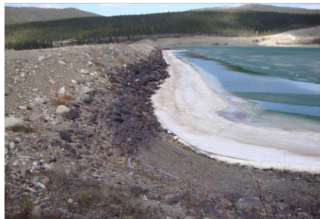
Photo 15: CVD upstream slope conditions.
