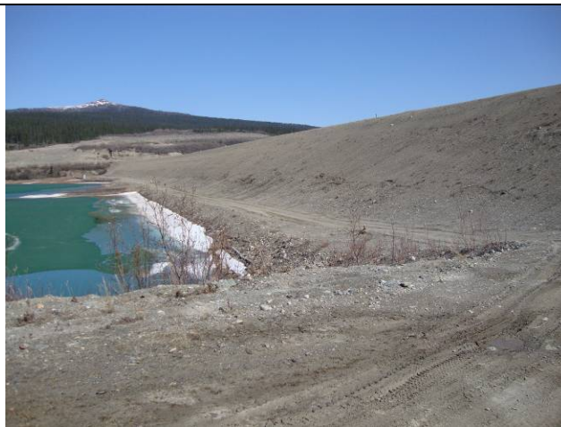
Photo 14: ID downstream stream slope conditions.
