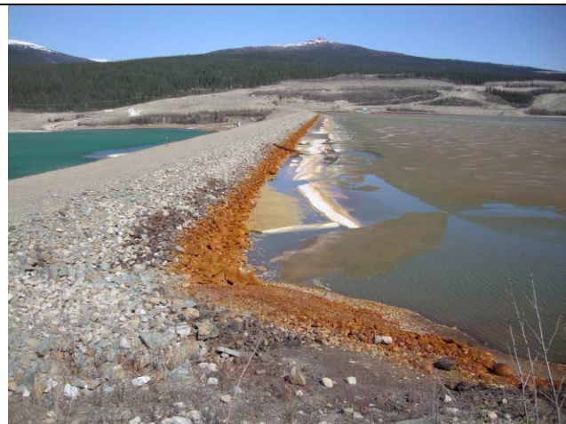
Photo 13: ID upstream slope conditions.
