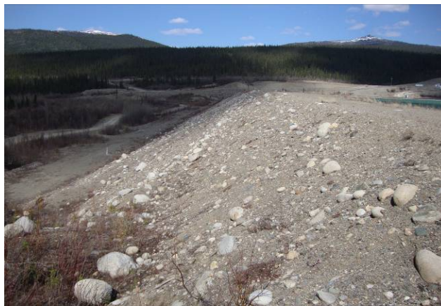
Photo 16: CVD downstream stream slope conditions.
