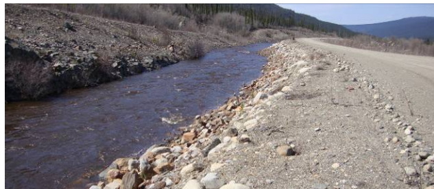
Photo 11: Channel condition looking downstream RCDC.
