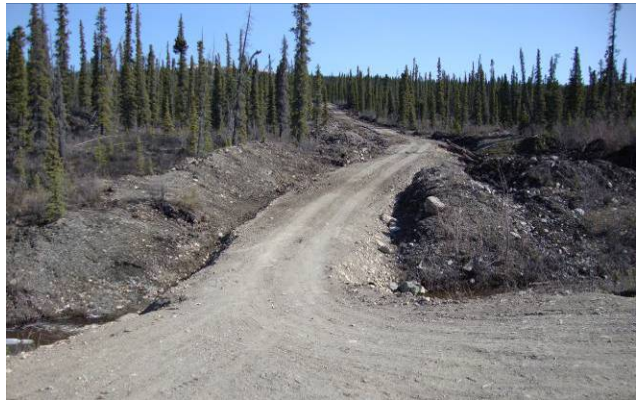
Photo 8: Service road crossing conditions looking north from NWID towards fresh water supply well.
