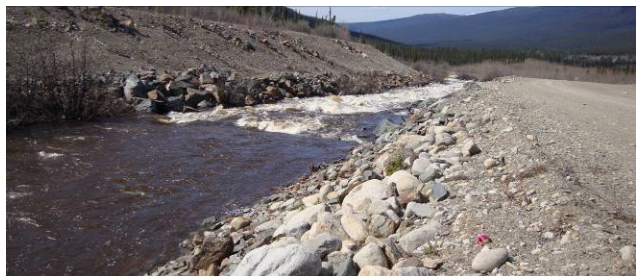
Photo 12: Channel condition looking downstream RCDC.
