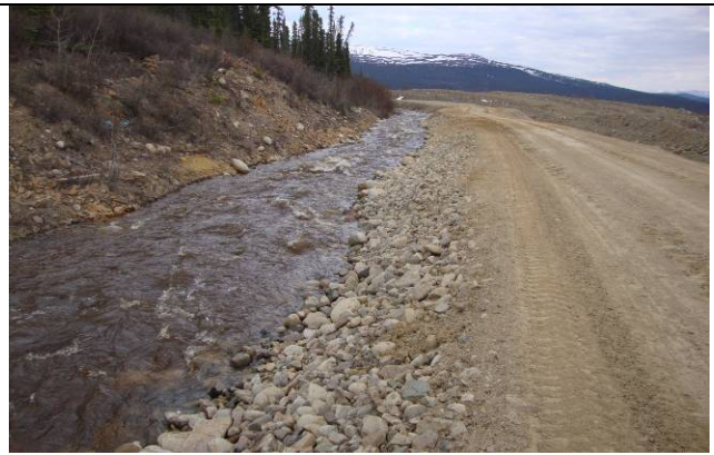
Photo 2: Lower portion of FCDC looking downstream.
