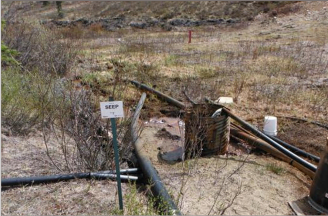
Photo 33: Seepage Discharge Point. Note MW09-08 in Background. June 3, 2012
