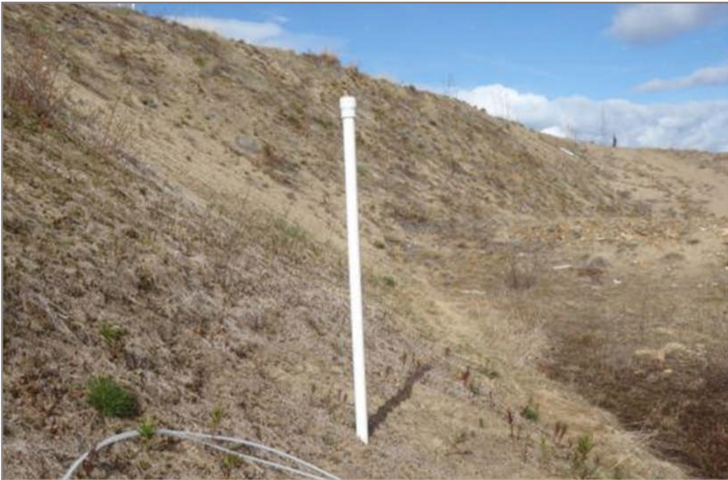
Photo 20: MP09-04 Located North of the Seepage Pond. June 3, 2012
