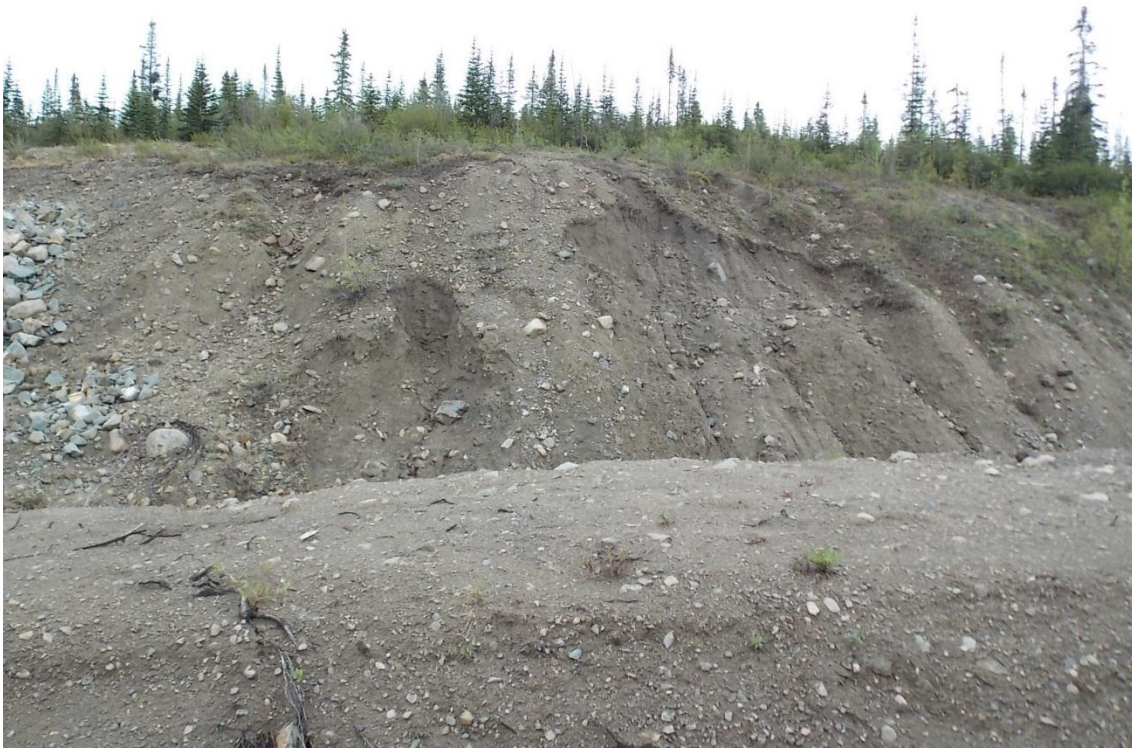
Photo 3-1. Sloughs located on the backslope at the Faro Creek Diversion Channel (June 13, 2013).
