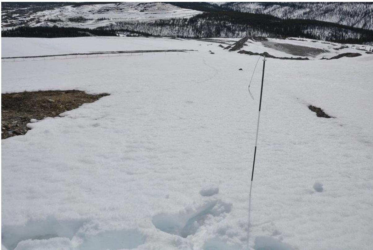
Photo 3-3. View looking down the perimeter ditch along the southwest side of the GSC cover; 1 m of snow indicated by probe (May 10, 2013).
