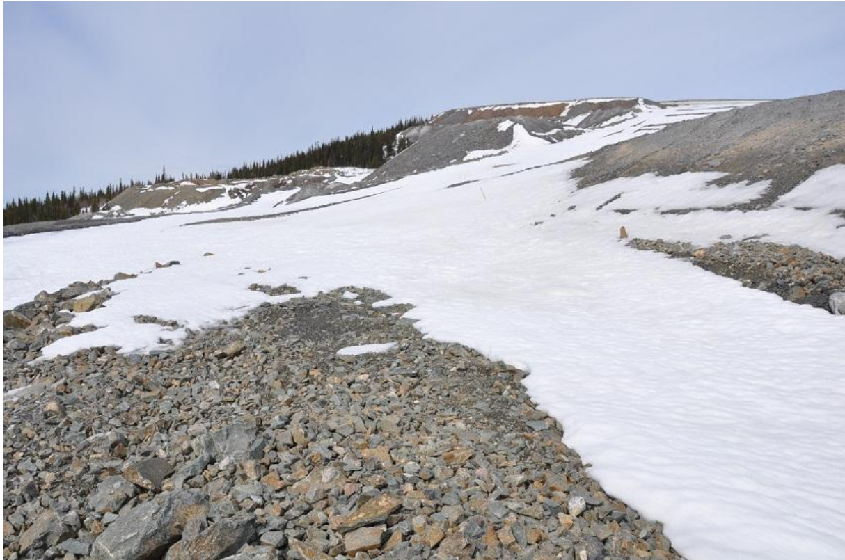
Photo 3-2. View looking south onto West Dissipation Pond (mid-ground) and perimeter ditch heading uphill to the right background (May 10, 2013).
