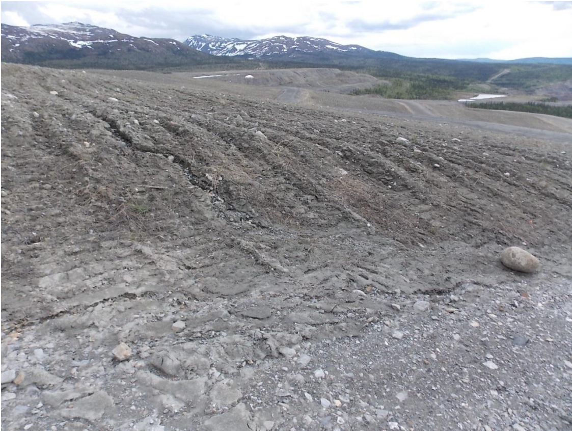
Photo 3-4. Longitudinal gully on cover surface near south perimeter ditch (June 13, 2013).
