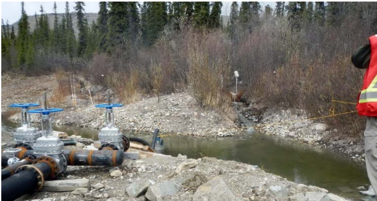
Photo 2-2. View of water collection and pumping elements at Pumping Station V15 at the confluence of V15 seep and Grum Creek seep (May 21, 2014). V15 water comes in from the southwest portion of the dump from the left channel. Grum Creek emerges from under the northeast corner of dump and flows over monitoring location GC Weir (white container marking channel at right-center of photo).
