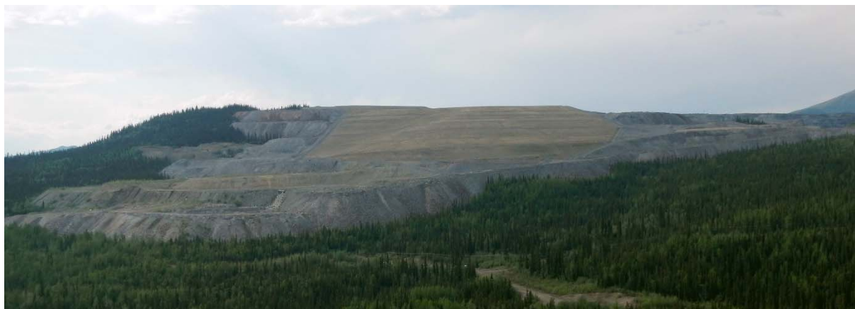
Photo 3-2. View of the GSC cover, taken from the Vangorda Waste Dump. Note the light gray original waste rock surface around the reclaimed olive brown GSC cover (May 26, 2015).
