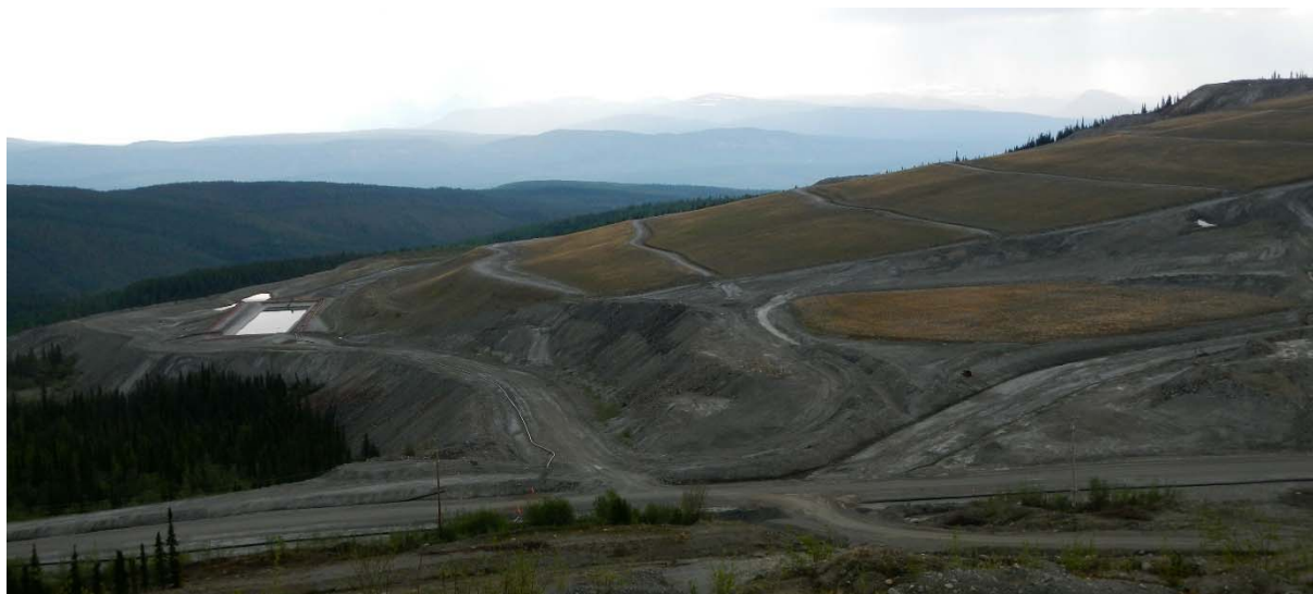
Photo 3-1. View of the lower portion of the GSC cover, with the Vangorda Access Road in the foreground. Vegetation cover now pronounced. Note the water retained in both the Lined and Unlined Ponds located at the toe of the cover (May 26, 2015).
