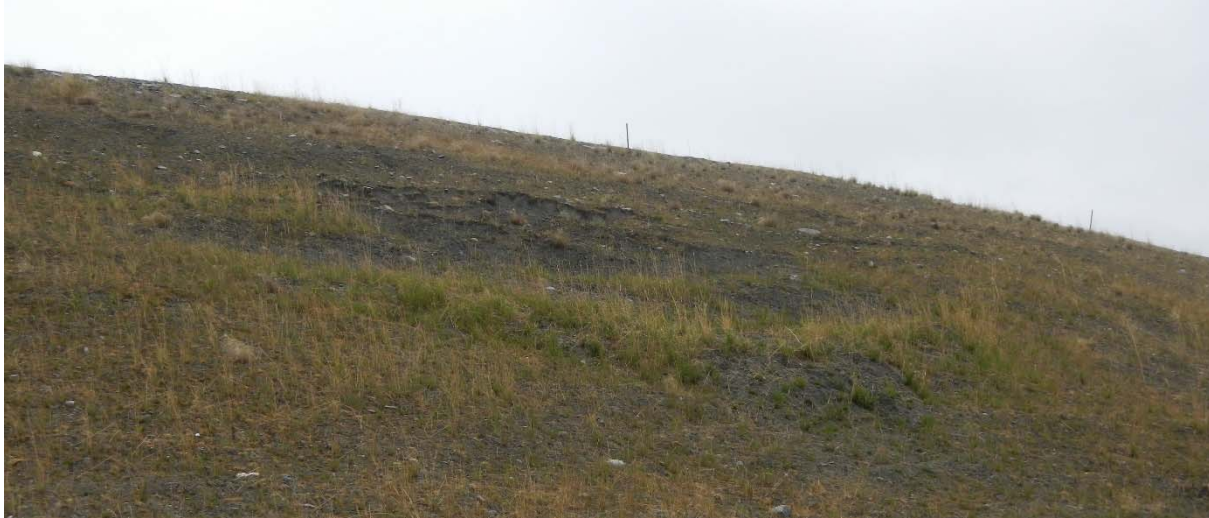
Photo 3-9. View of the small slough (one of three) on slope above diversion ditch (May 27, 2015).
