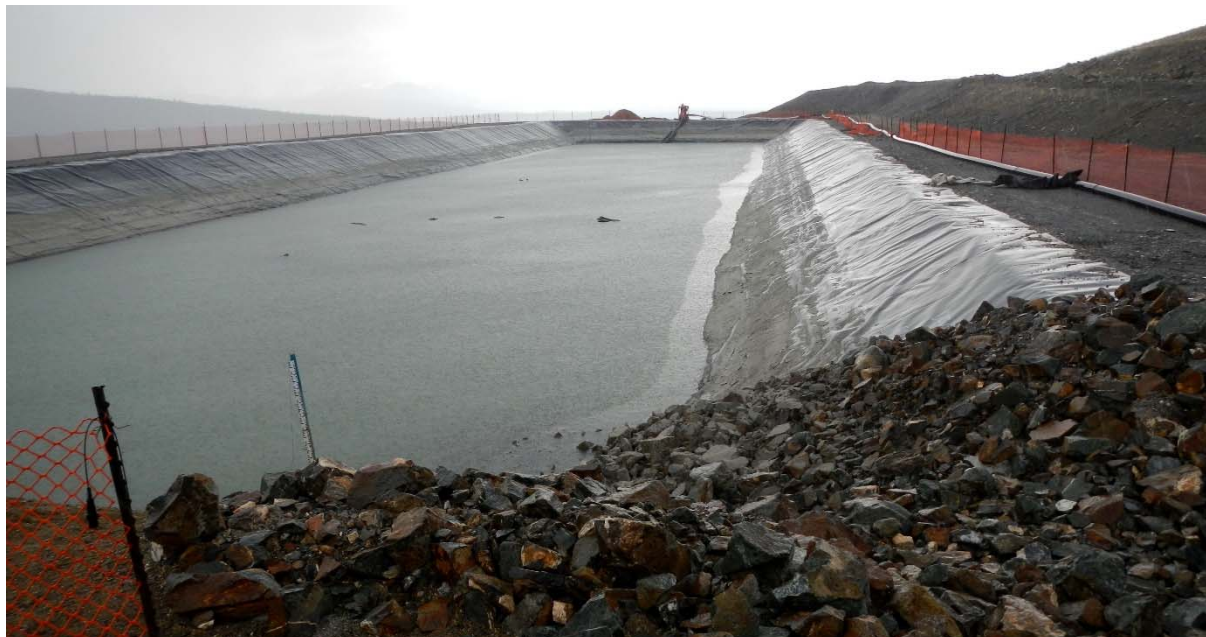
Photo 3-3. View of the Lined Pond and staff gauge (May 26, 2016).
