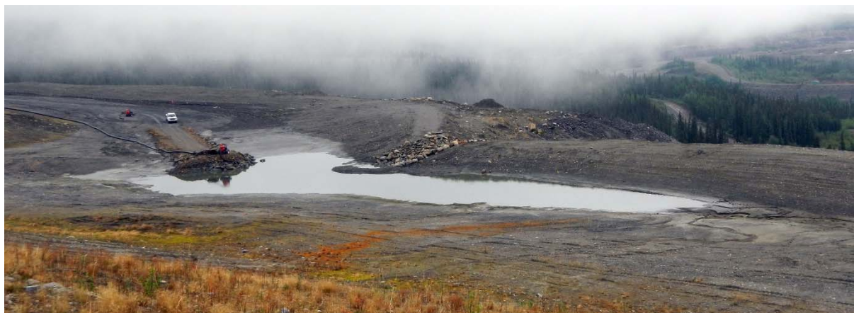
Photo 3-4. View of the Unlined Pond and associated pump arrangement up to Lined Pond (May 27, 2015).
