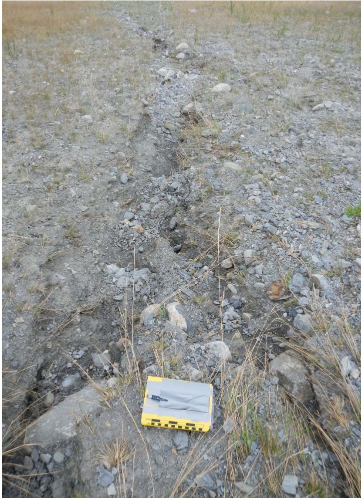
Photo 3-8. View of erosional gully from fourth bench (May 27, 2015).
