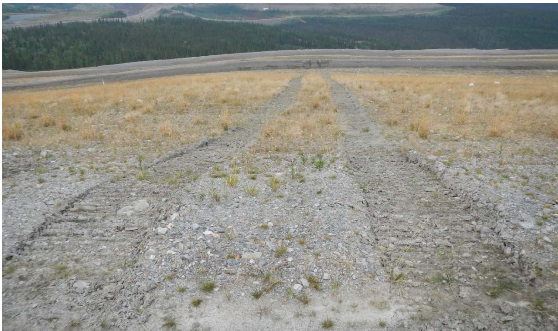
Photo 3-6. View of the excavator tracks from third bench looking down onto fourth bench. Note grass cover has been trampled under tracks, along with minor depressions have been formed (May 27, 2015).
