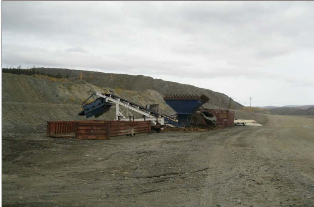
Photo 35: Machinery located to the north of the Warehouse
