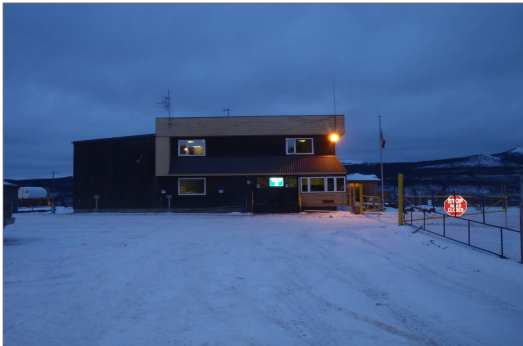
Photo 8: Guard house looking south
