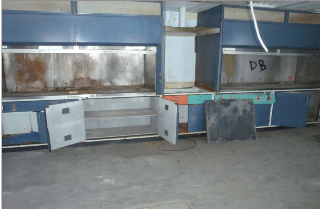
Photo 13: Asbestos containing transite cement board associated with the cupboards and fume hood in the 2 nd floor lab of the warehouse
