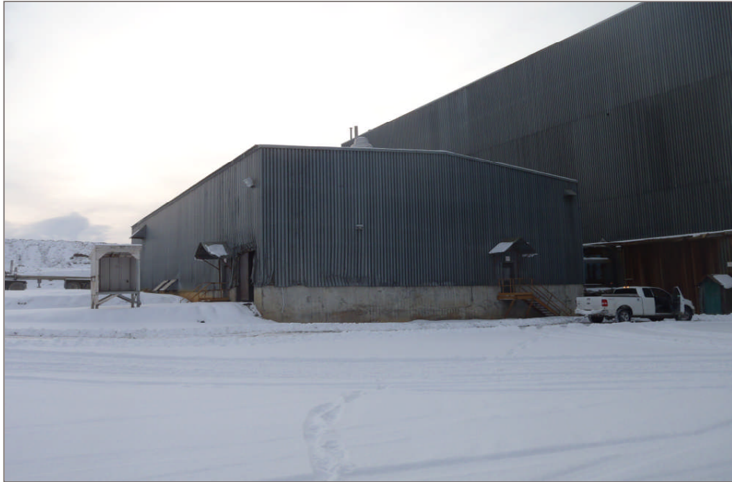
Photo 5: Reagents building looking east
