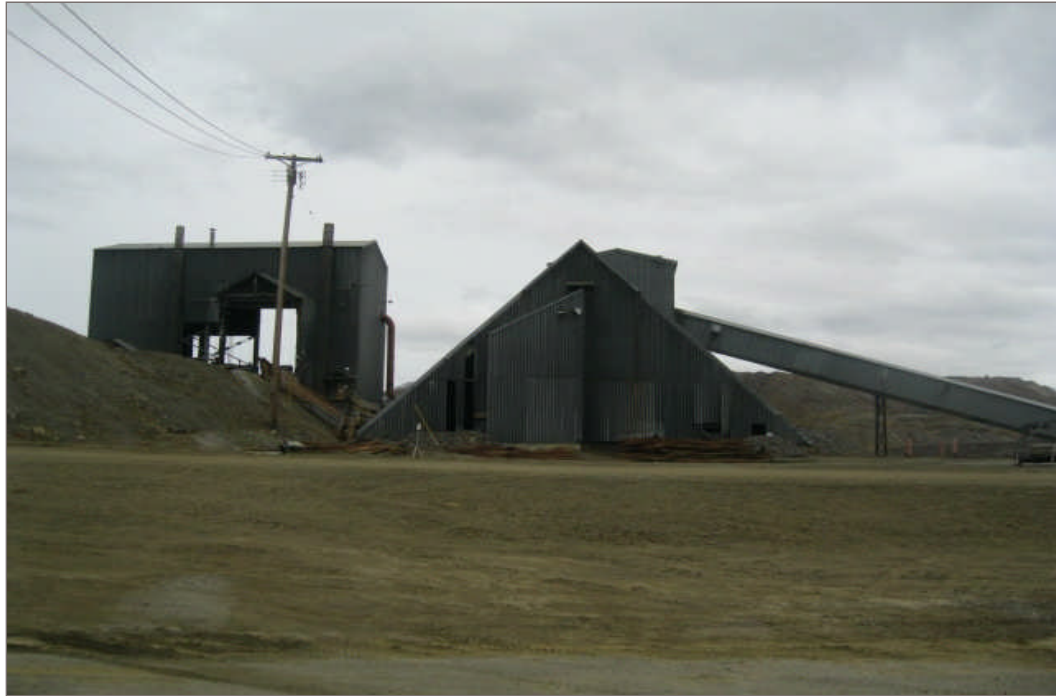
Photo 7: Fine ore building looking east
