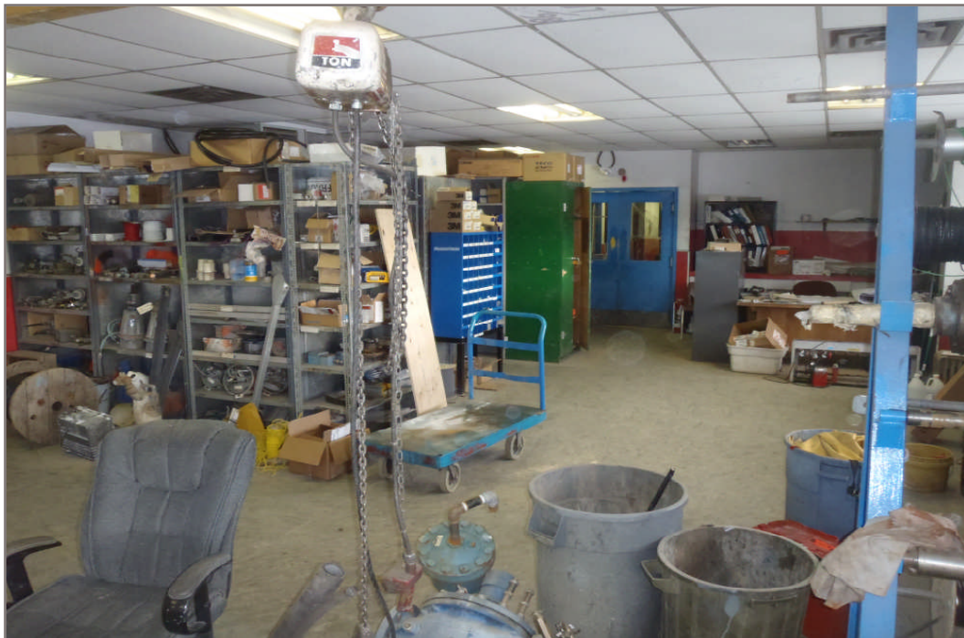
Photo 22: Blue lead based paint requiring regulated disposal applied to various surfaces within the storage area of the mill.
