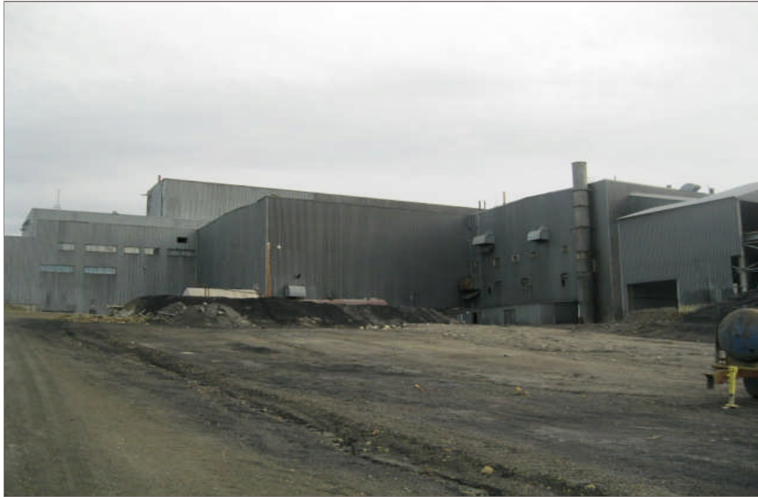
Photo 3: Mill Building looking north
