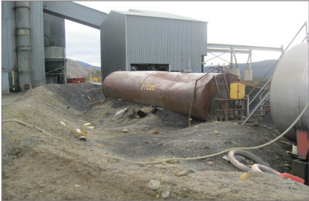
Photo 29: Hydrocarbon tanks located at the south end of the Mill
