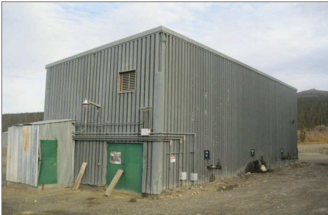
Photo 2: Fluid storage building containing three large AST's looking north
