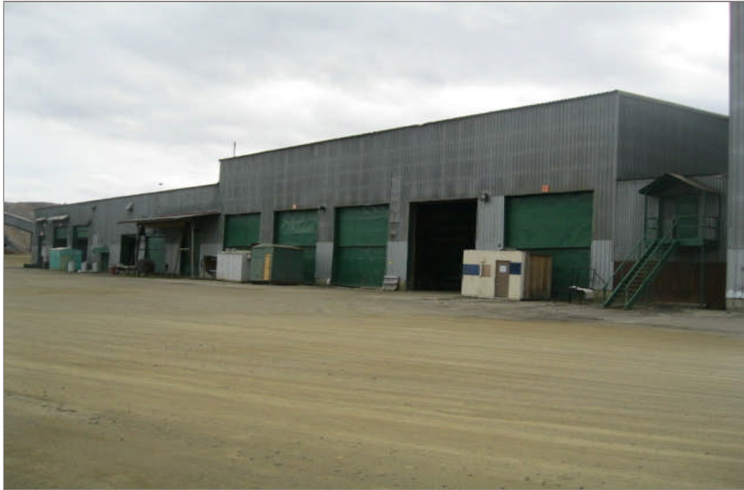
Photo 1: Main Warehouse Building looking east
