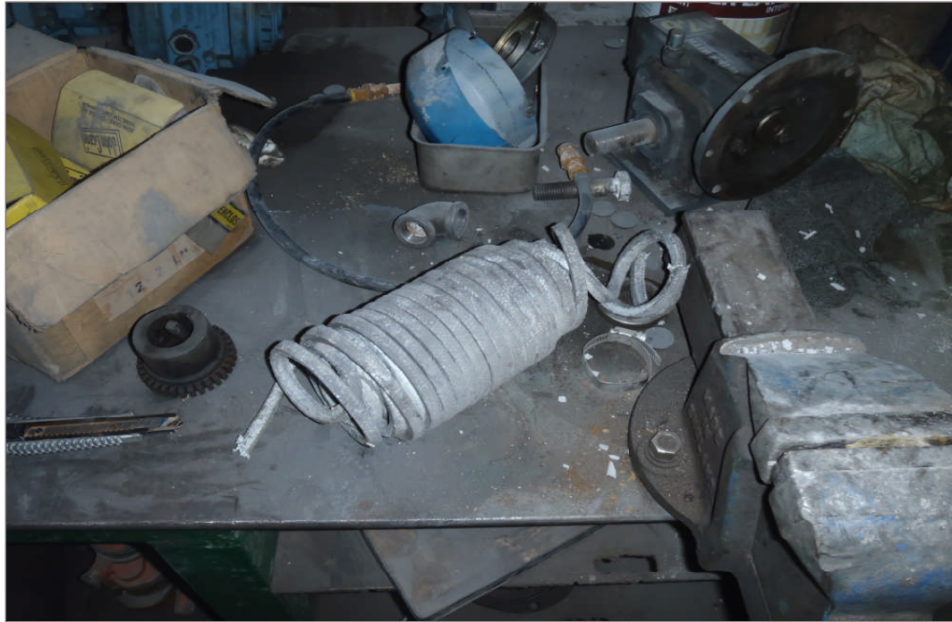
Photo 17: Asbestos containing pump packaging located in the Machine Shop of the Mill . The packaging is believed to be used on numerous machines within the Mill requiring gaskets.
