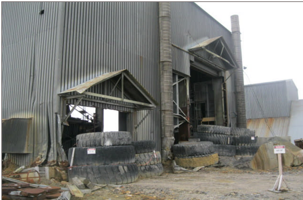
Photo 6: Crusher building looking south
