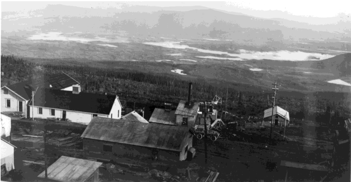
Photo shows Northwest Wernecke (right to left) B7 Stable, B8 Boiler house and part of the east wall and the roof of outhouse B10
