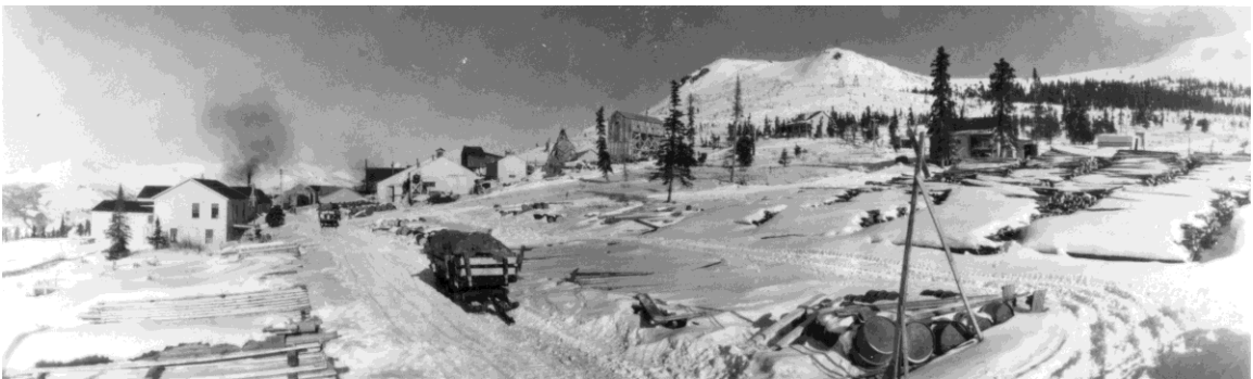
Wernecke Camp, facing north, Scene of buildings and underground lagging and or firewood off to each side of the photo.
