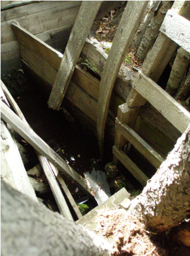
The cribbing of the shaft is rotten and collapsing with only a small opening remaining.
