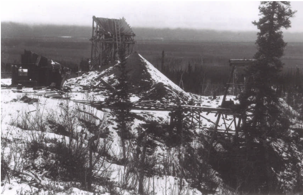
6695 - 22 October 1923 Silver King Mine. A view of the shaft and ore dump of the earliest workings on the Silver King mine site, a few miles west of Elsa on Galena Creek
