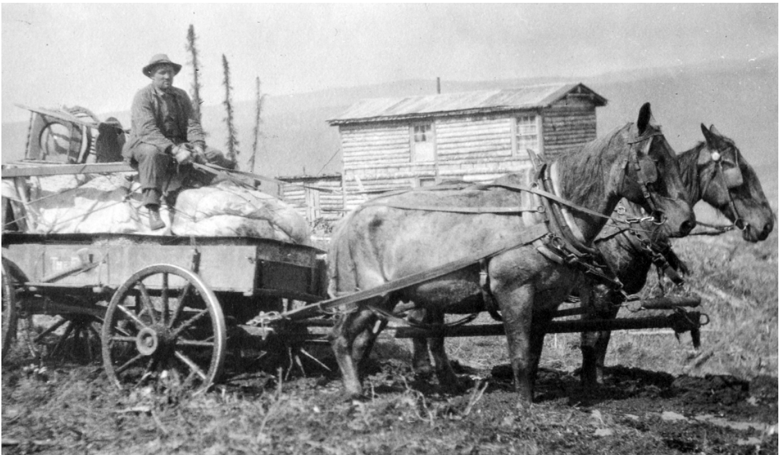
83_5_2 Eugene and Gertrude Fournier fonds Road House at Silver King Courtesy Yukon Archives
