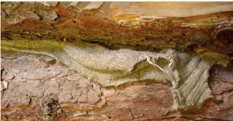
The log walls were chinked with moss, mud and strips of long johns and burlap.
