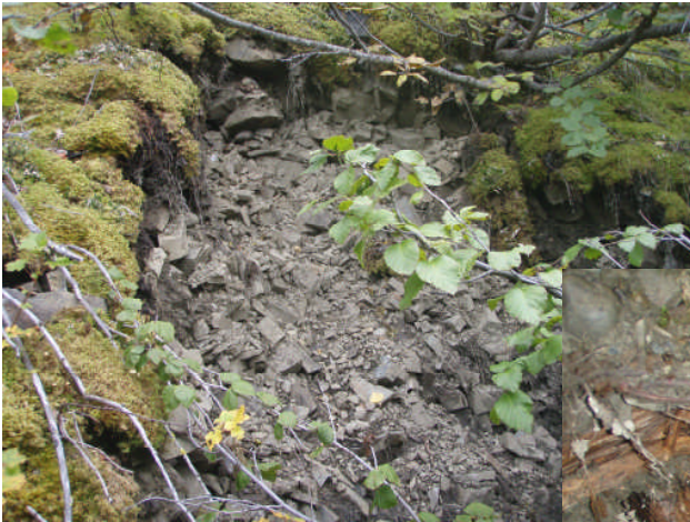
The adit has collapsed directly above the entrance.
