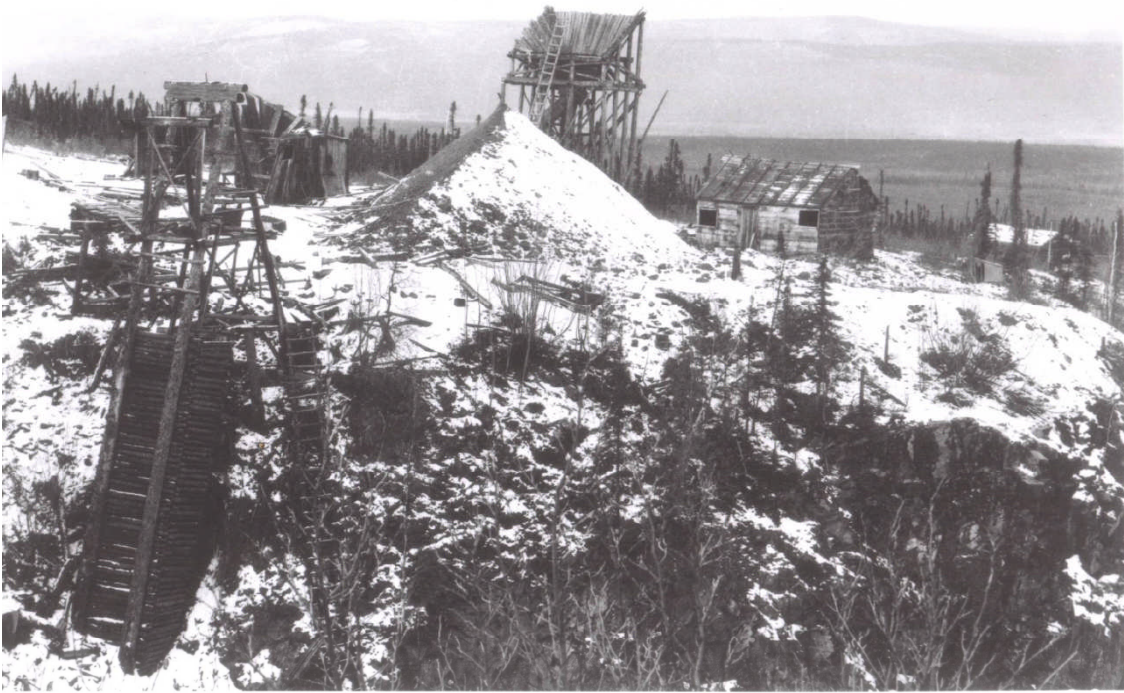
6696 - 23 October 1923 Silver King Mine – a view of the earliest workings of the old Silver King Mine taken from the opposite side of Galena Creek
