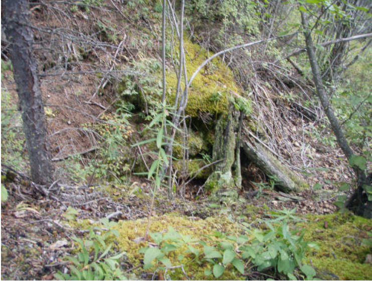
The Gravel Adit has collapsed with only rotten timbers, rail and metal remaining.
