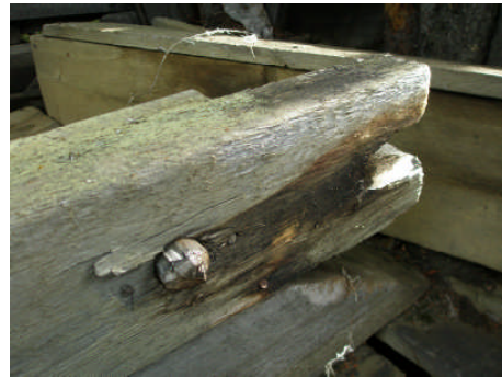
The cribbing of the shaft is rotten and collapsing with only a small opening remaining.
