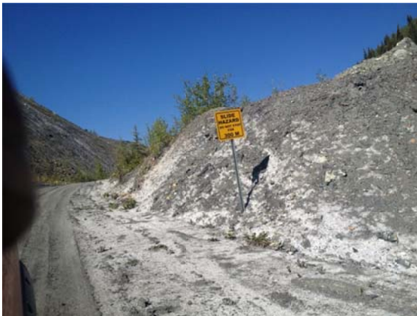
Photo 40 - Sign on waste rock pile near Clinton Creek
