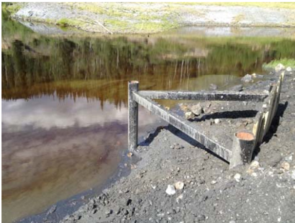
Photo 19 – Installed south abutment
