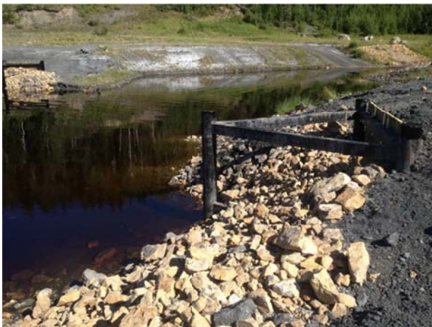
Photo 29 - Installed south abutment
