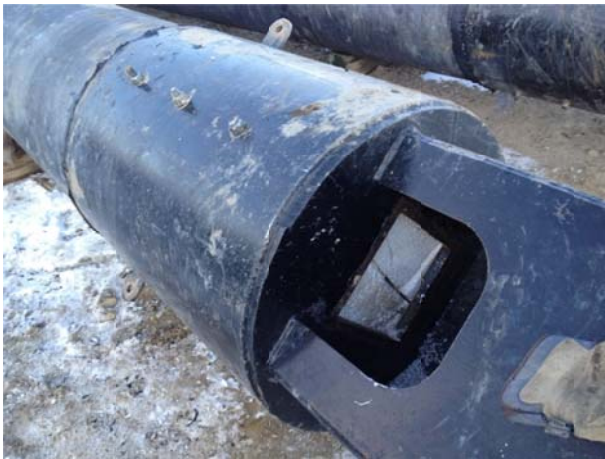
Photo 49 - Foam installed in pipe and end cap installed
