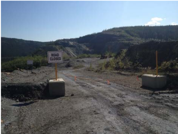
Photo 33 - Gate and sign at access road to abandoned shovel and drill
