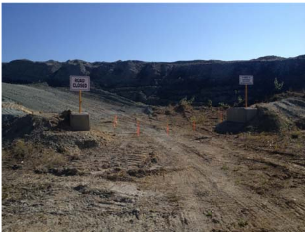
Photo 23 - Signage and gate at top of tailings pile
