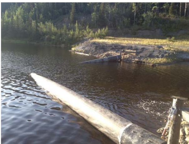
Photo 44 - Log-booms in place showing settlement in the water
