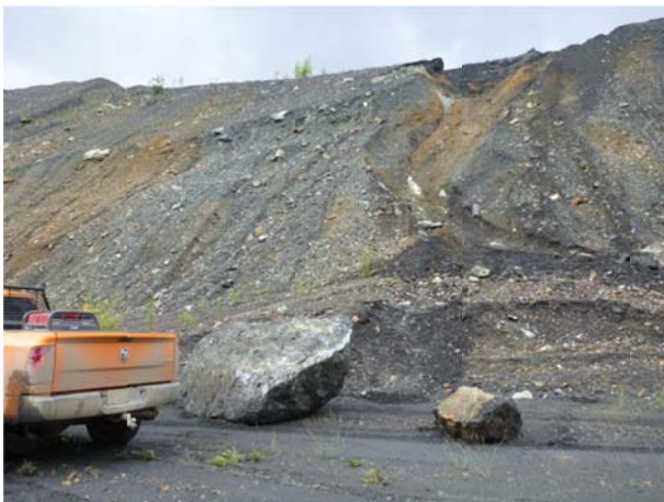
Photo 8 – Rock removed from slope and area it came from
