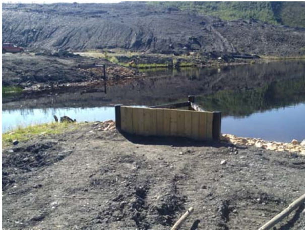
Photo 28 - Installed north abutment
