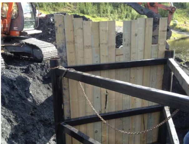
Photo 20 - Installing north abutment
