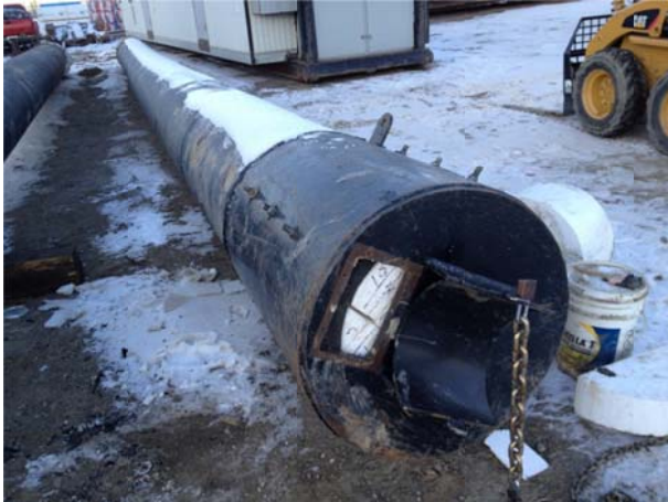
Photo 46 – Flotation foam installed in pipes
