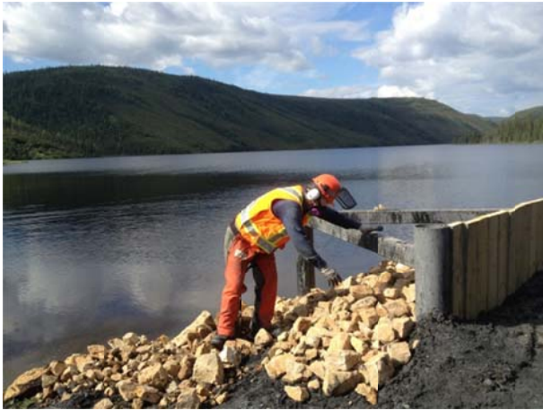
Photo 21 Placing rip rap around north abutment
