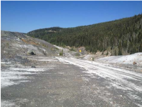
Photo 36 - Soft Shoulder sign on road along waste rock pile
