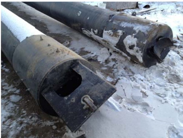
Photo 50 - Foam installation complete with inspection covers installed
