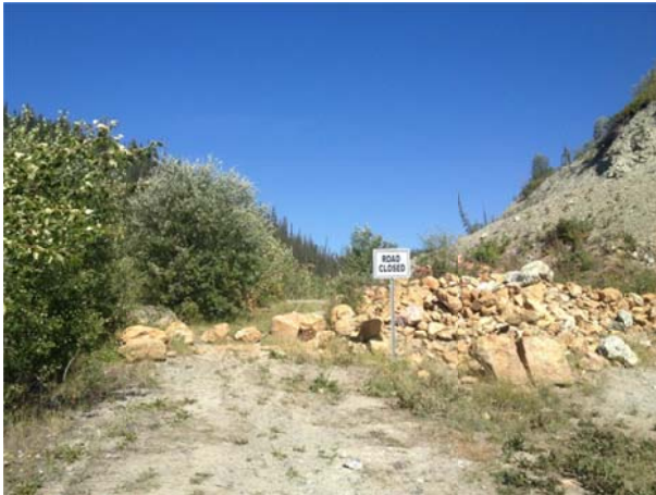
Photo 42 - Sign and rock blockage at Wolverine Creek access
