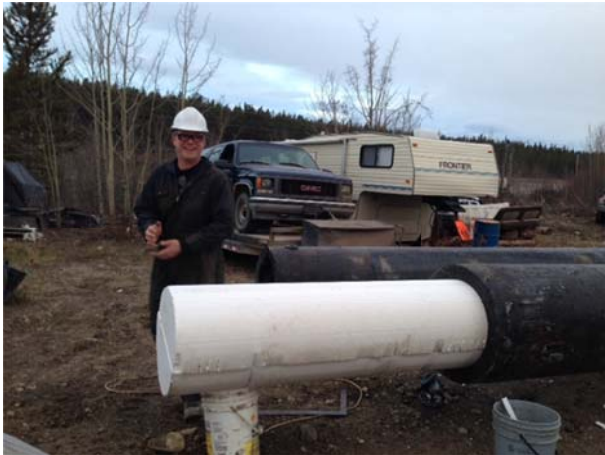
Photo 48 - Foam being placed in pipe
