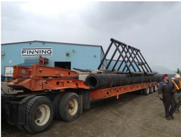
Photo 16 - Delivery of pipes and abutment structures to site
