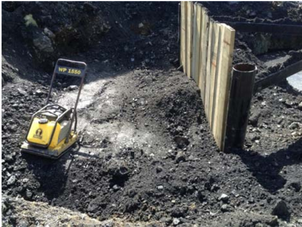
Photo 18 - Installing abutment structure and compacting backfill
