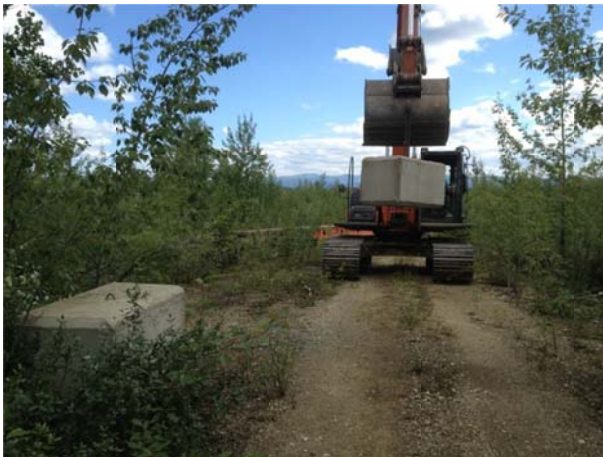
Photo 4 – Placing lock blocks at the airport road
