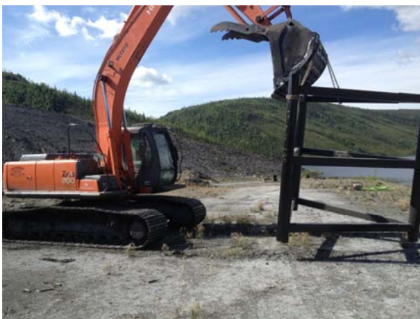
Photo 17 - Unload abutment structure from truck
