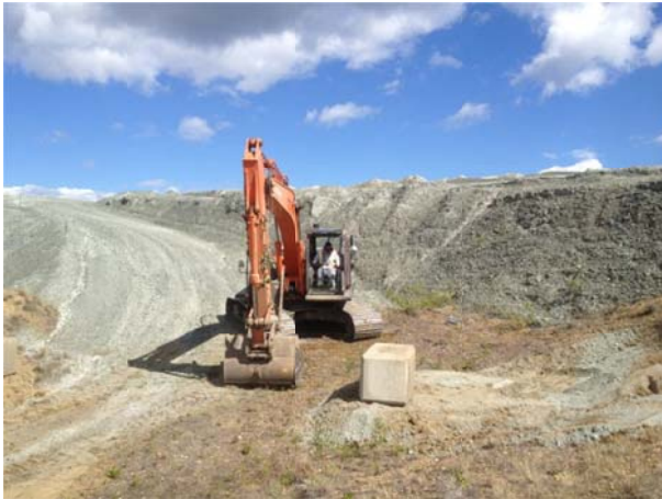
Photo 3 – Hitachi ZX 200 unloading lock blocks at gate locations
