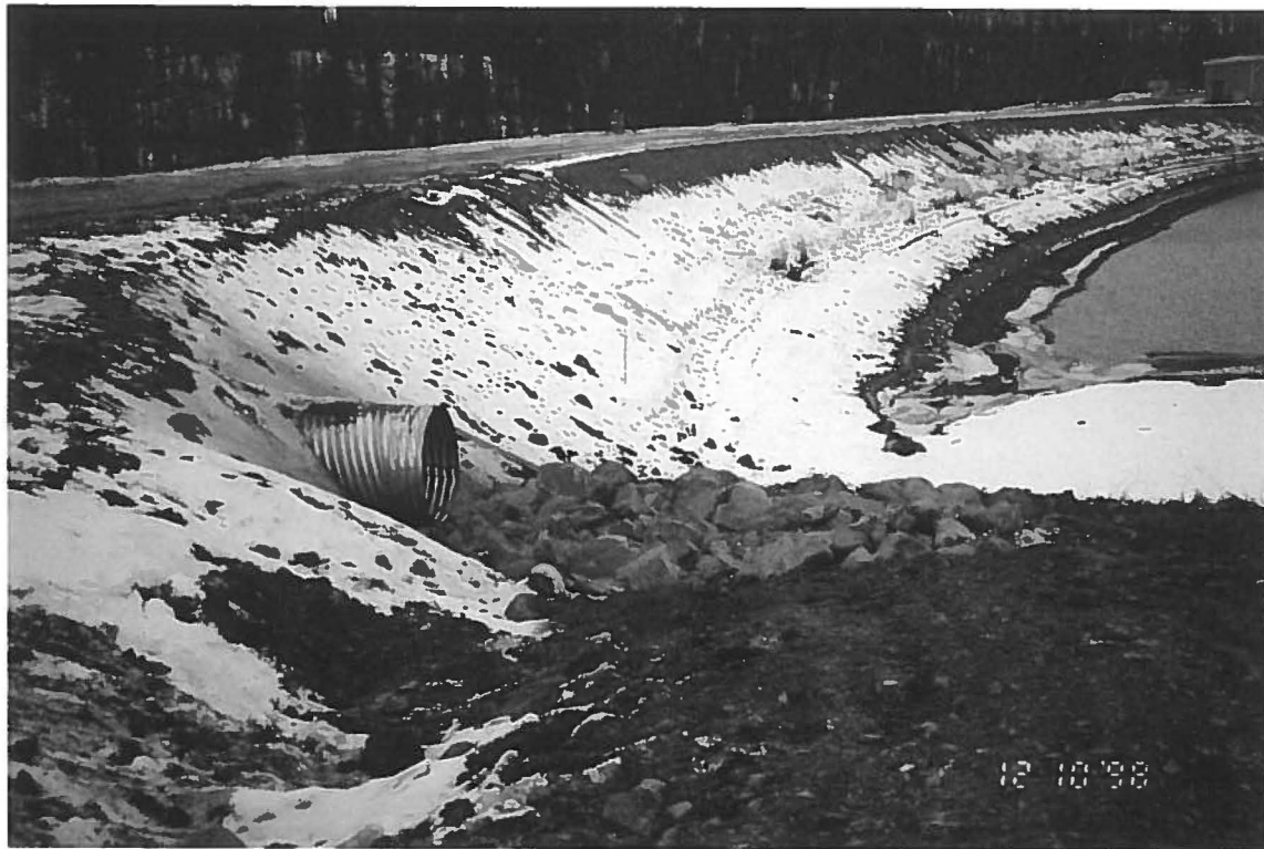
Photo 8 - Inlet of culvert spillway.
