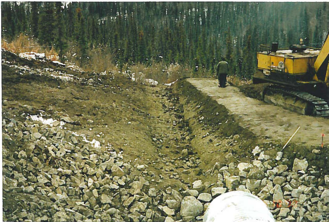
Photo 2 - Compaction of earth filled dyke.
