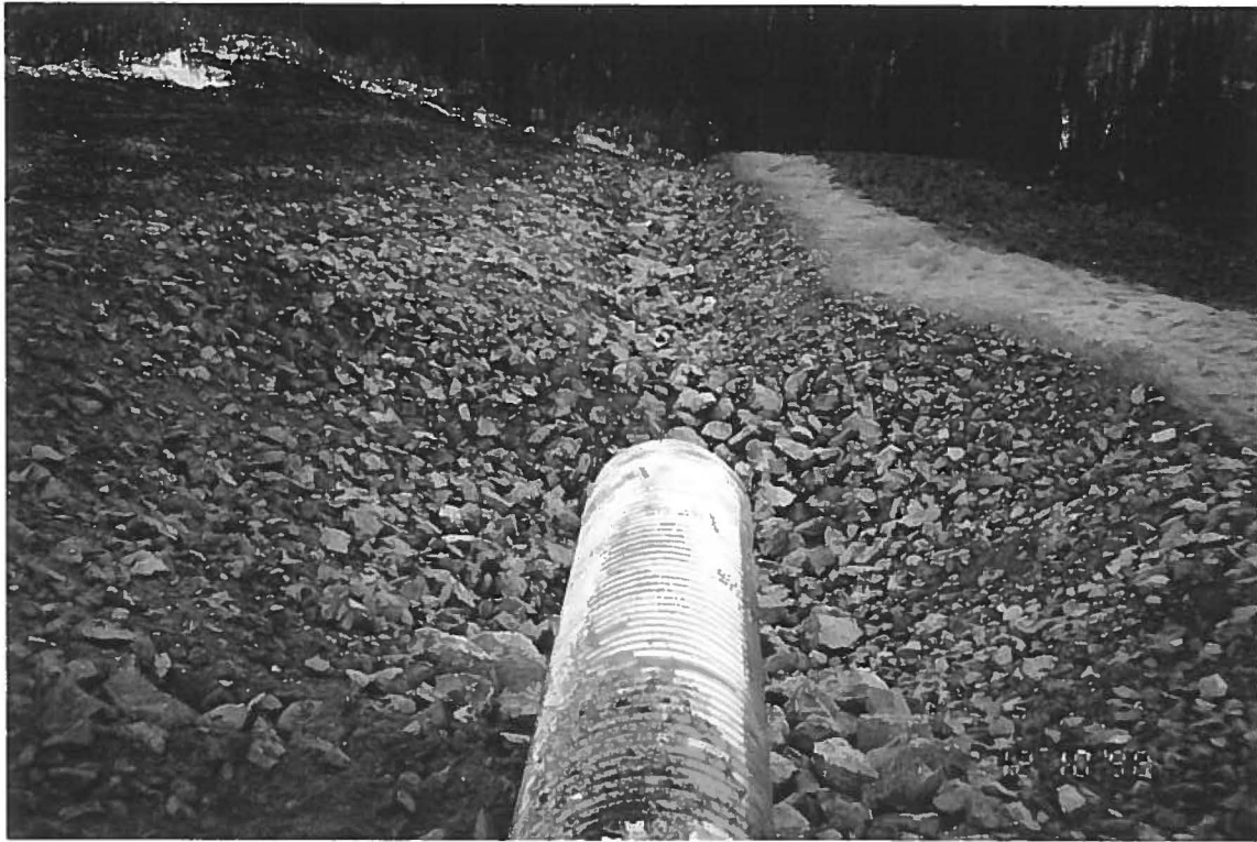
Photo 7 - View from dam over culvert outlet and plunge pool.
