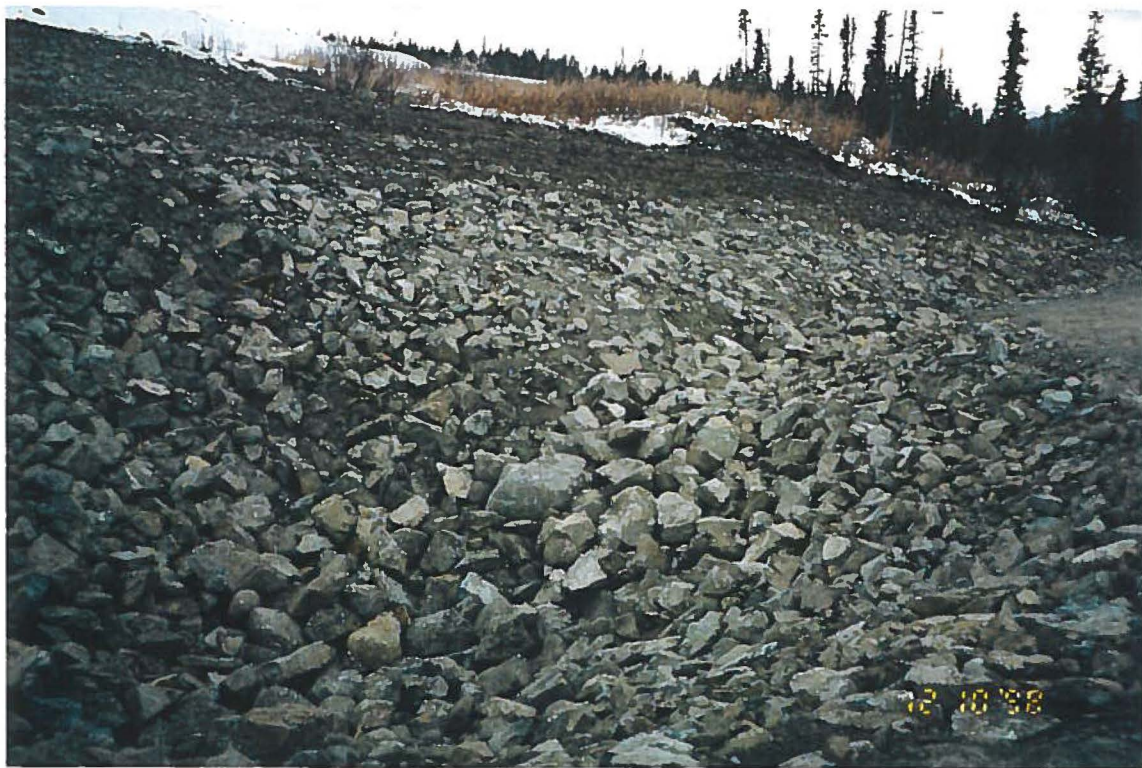
Photo 4 - Outlet of plunge pool.
