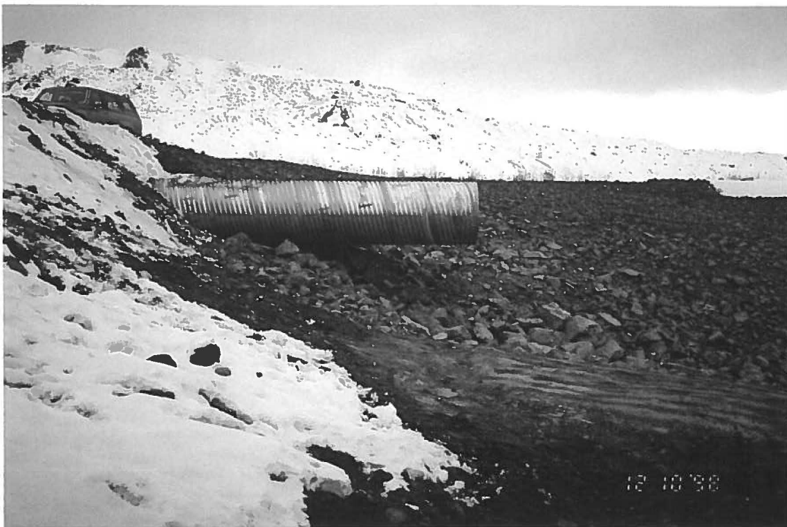
Photo 6 - Elevation view of culvert outlet.
