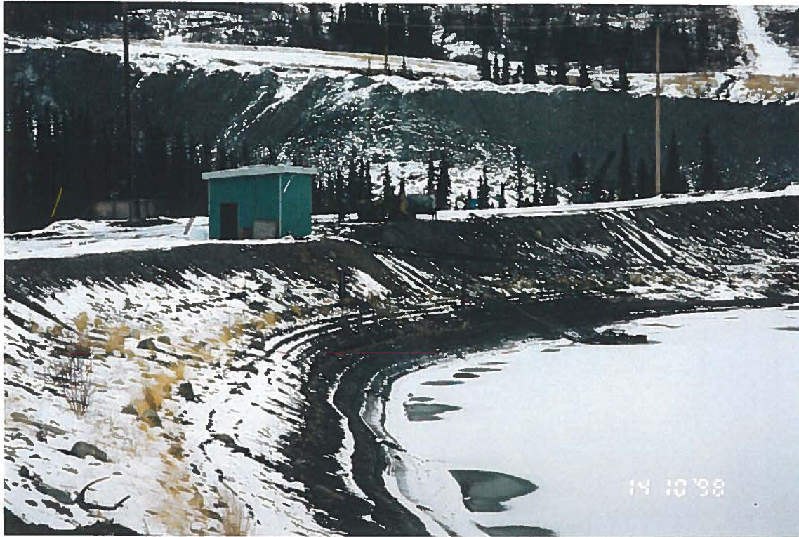
Photo 11 - View of pumphouse on Little Creek Dam
