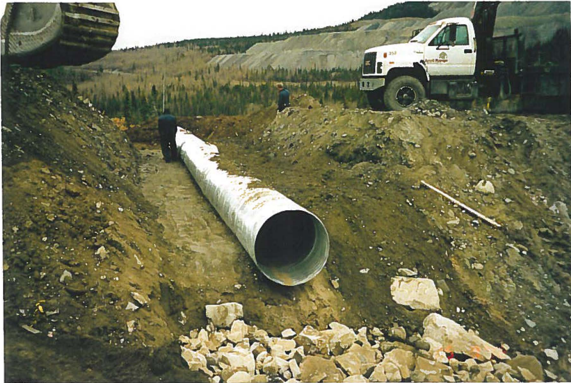
Photo 1 - Compaction of backfill around haunching of 900mm CNP culverts.
