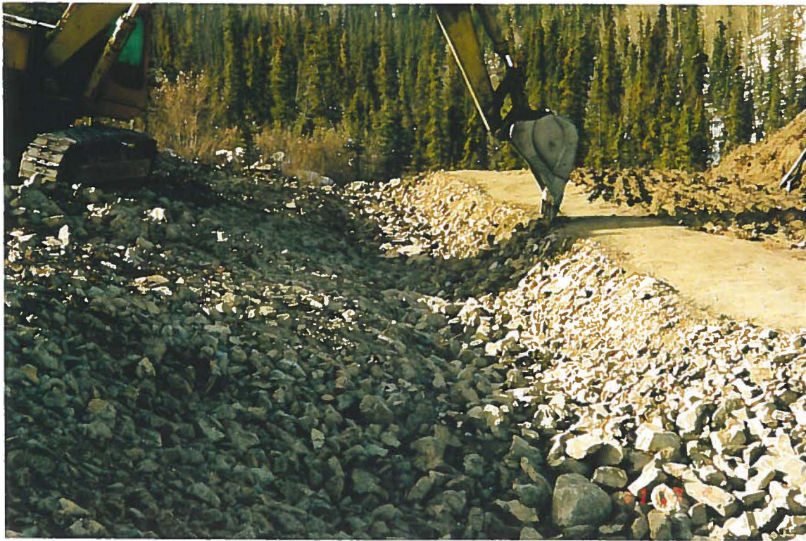
Photo 3 - Placement of riprap in exit channel from plunge pool.
