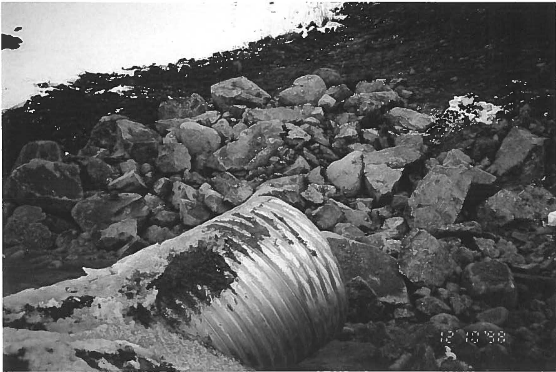
Photo 9 - Inlet to spillway
