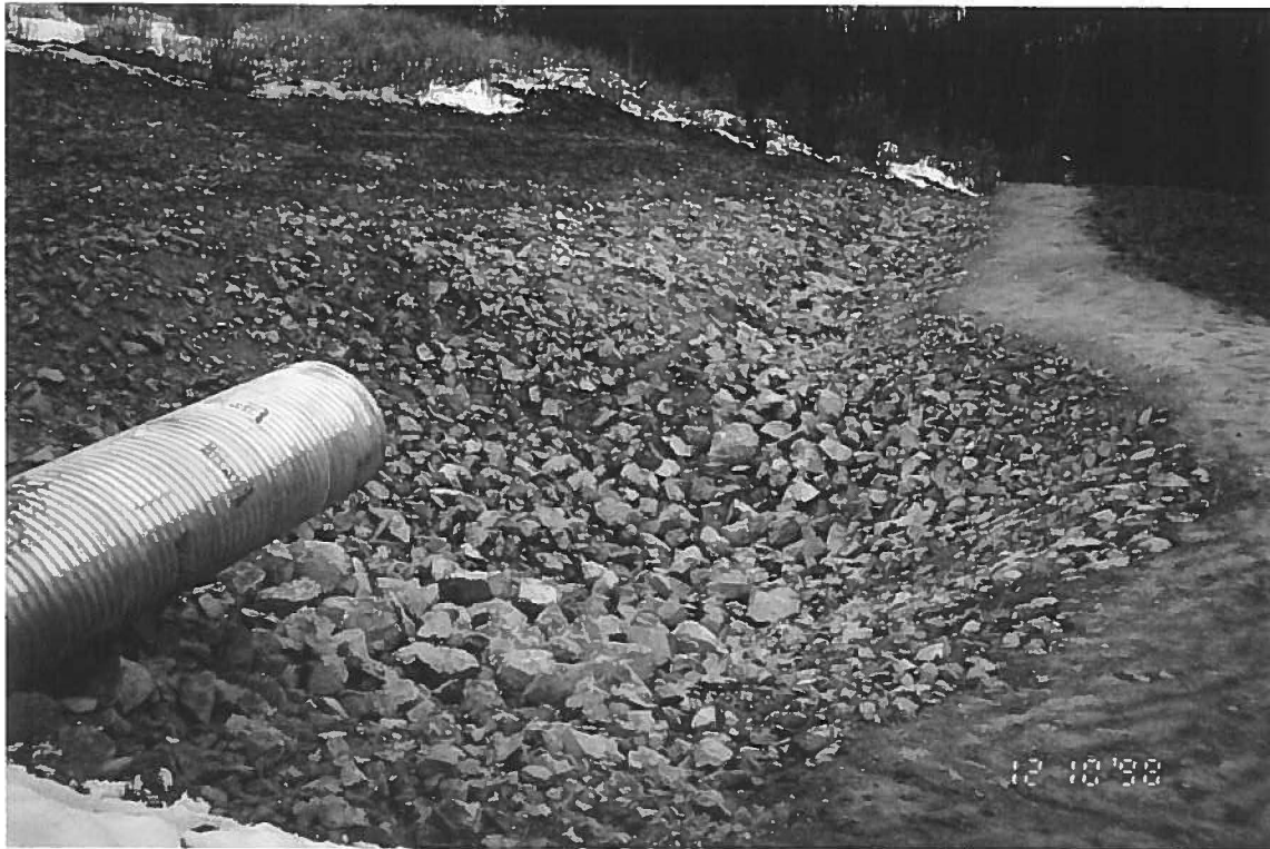
Photo 5 - View from Little Creek Dam looking out over culvert outlet and the plunge pool.
