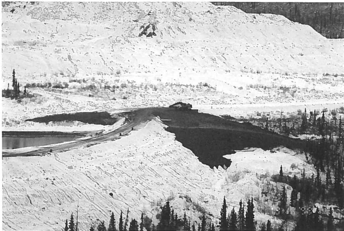
Photo 10 - View looking across at spillway with Little Creek pond to the left.
