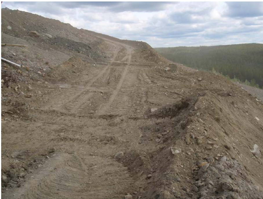
Photo 2: Access road from the east side, below CT#1
