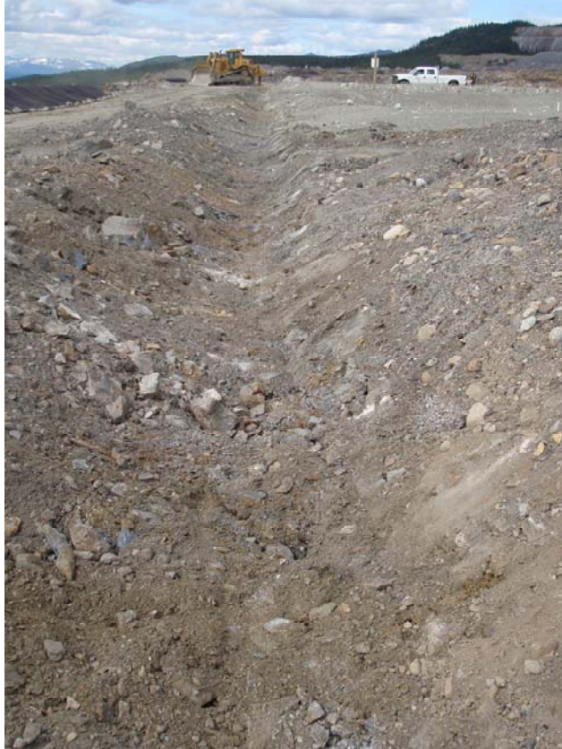
Photo 7: Drainage ditch, looking west
