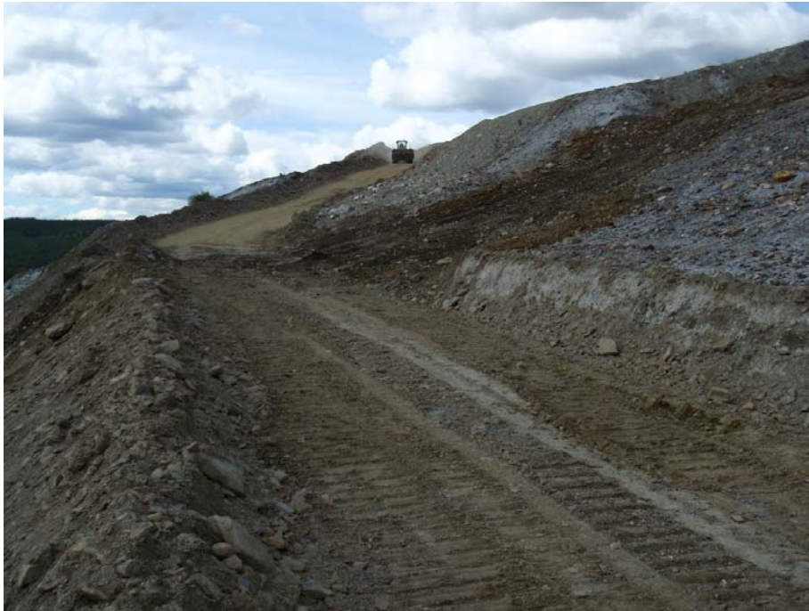
Photo 1: Access road from west side, below CT#4
