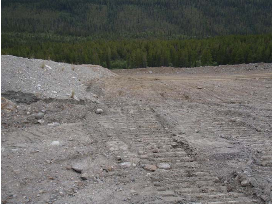
Photo 9: West side of CT#4, erosion has been repaired and compacted
