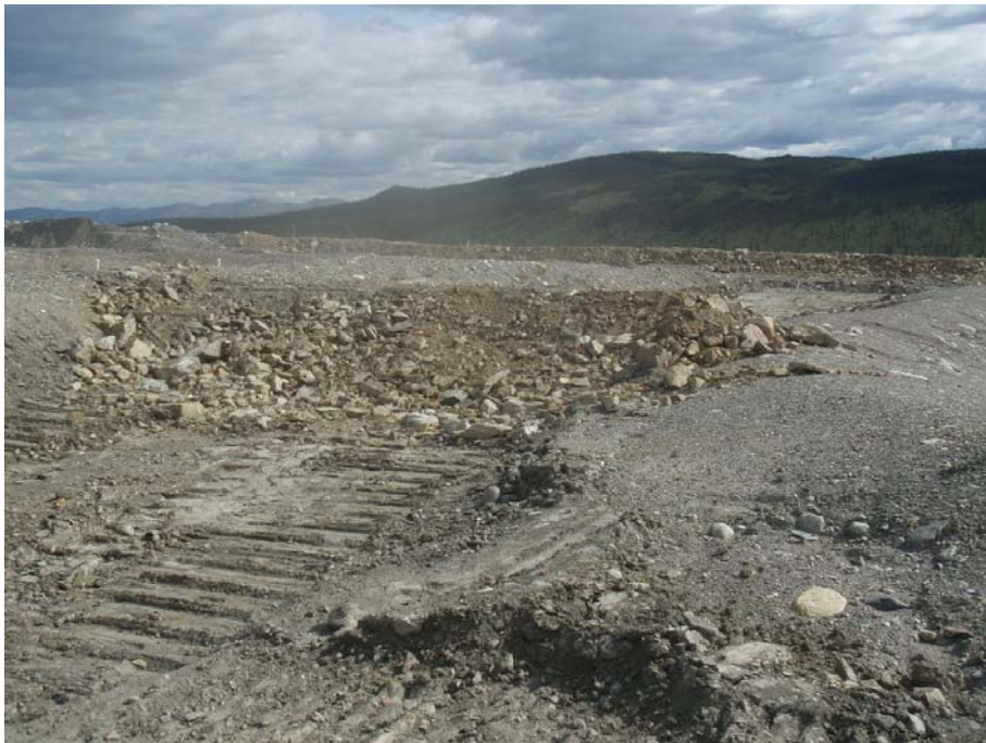
Photo 4: Berm 2 in foreground, Berm 3 in background
