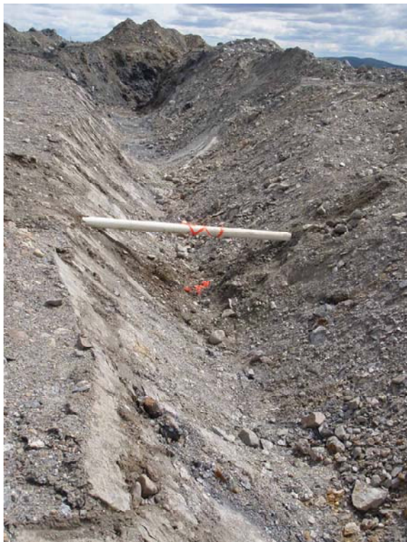
Photo 6: Drainage ditch, looking east. New pipe to protect wires
