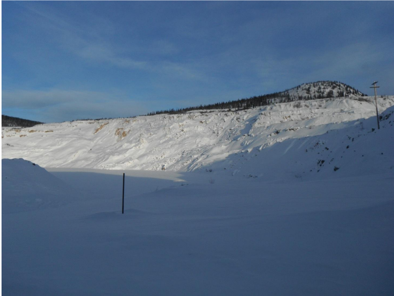
Photo 1: Faro Pit – January 18, 2012, Southeast Wall
