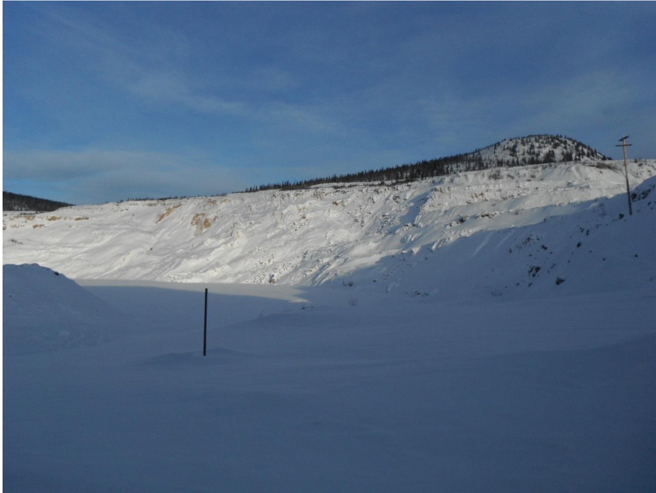
Photo 1: Faro Pit – January 18, 2012, Southeast Wall
