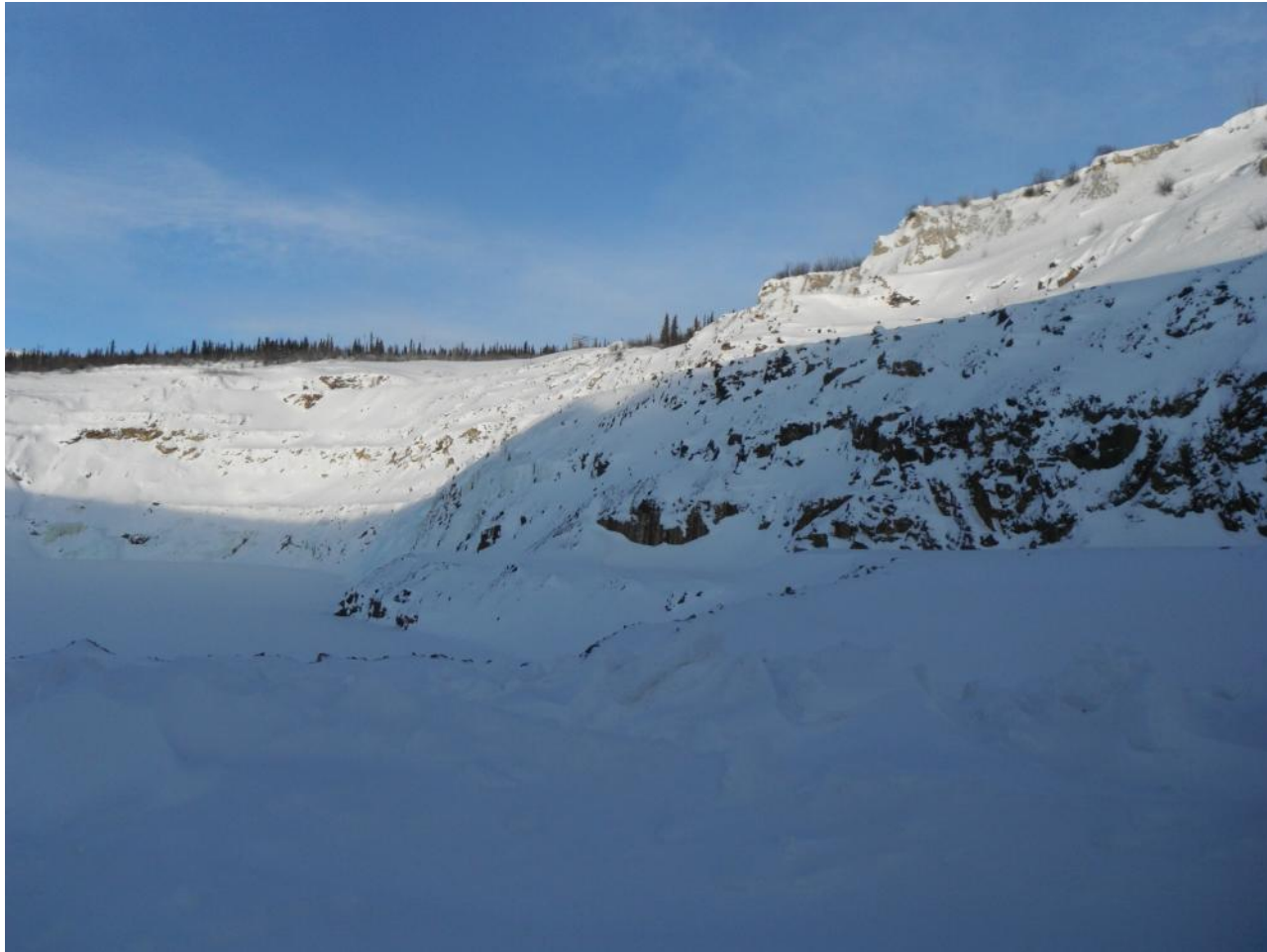
Photo 2: Vangorda Pit – January 18, 2012, Northwest/Northeast Walls
