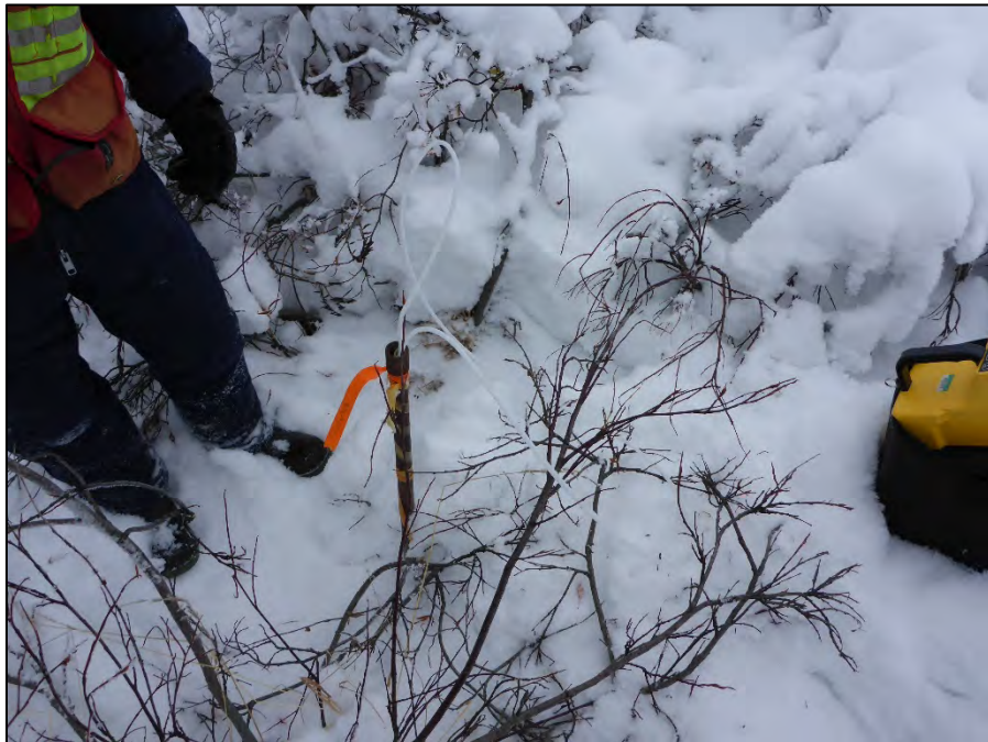
Photo 30: View of drive point well MP09-08. Photo taken on February 3, 2016.
