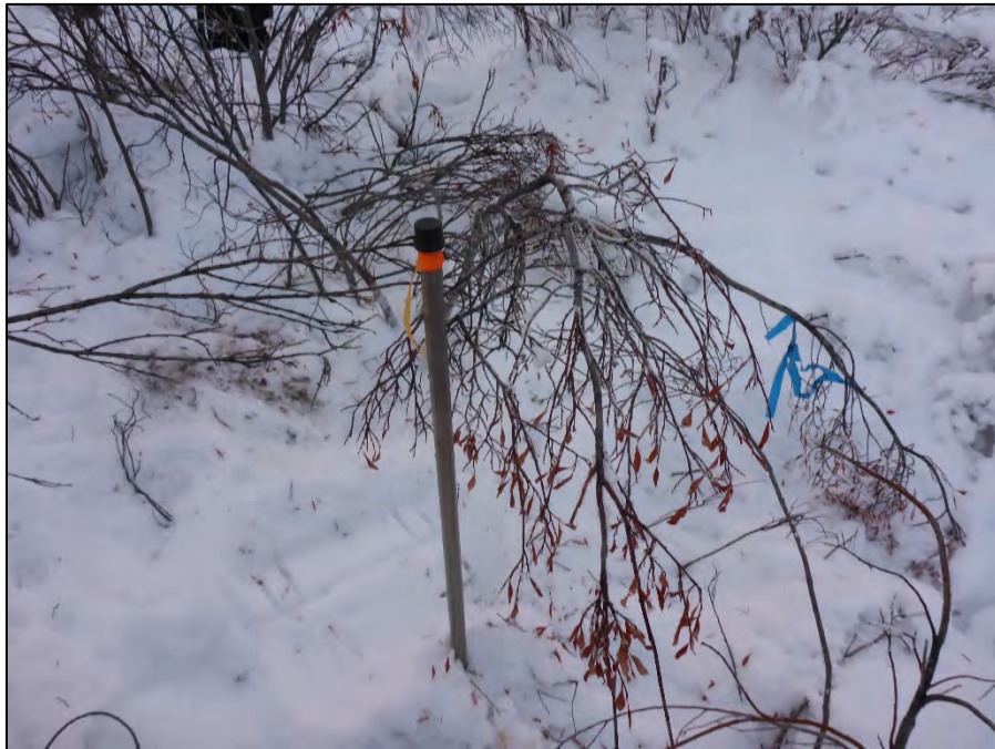
Photo 10: View of drive point well GSI-HA-01A. Photo taken on February 1, 2016.
