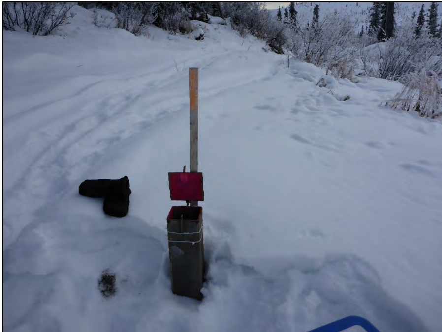
Photo 20: View of well CH-P-13-01/10. Photo taken on February 2, 2016.
