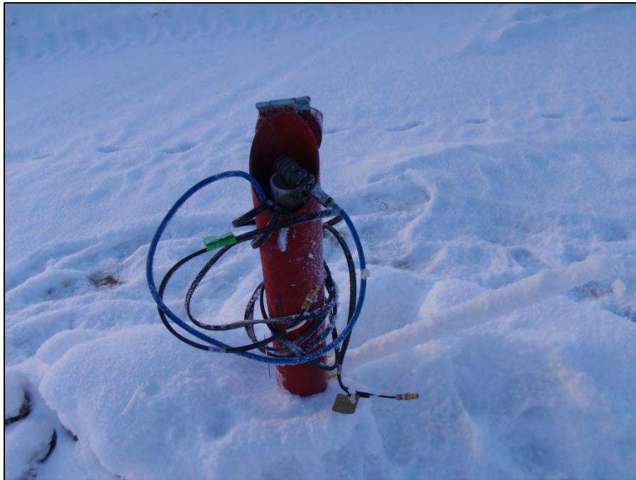
Photo 33: View of well W14103083BH04. Photo taken on February 2, 2016.
