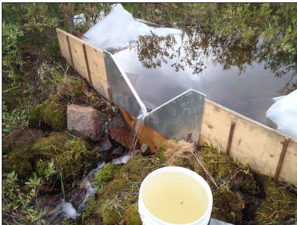
Photo 1. Upper Pony Creek (H-PC-U) v-notch weir; re-installed July 24, 2012.
