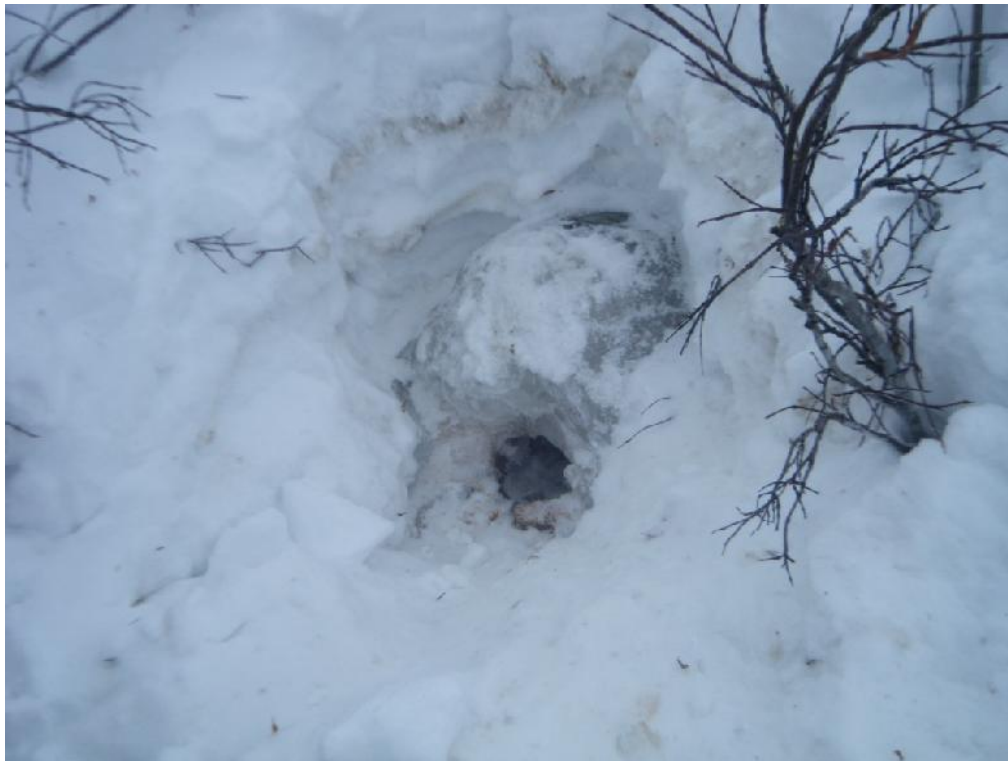
Photo 4. Pony Creek downstream of Pit (H-PC-DSP) – Frozen to substrate at culvert – February 1, 2012.
