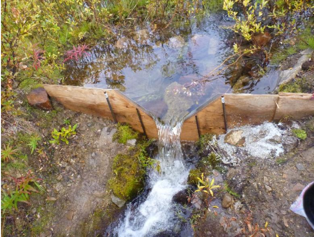
Figure 3. V-notch weir installation in the upper Pony Creek watershed (H-PC-U).
