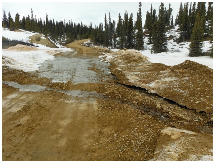
Photo 4. H-DC-R station showing flow of Dome Creek over the road crossing.
