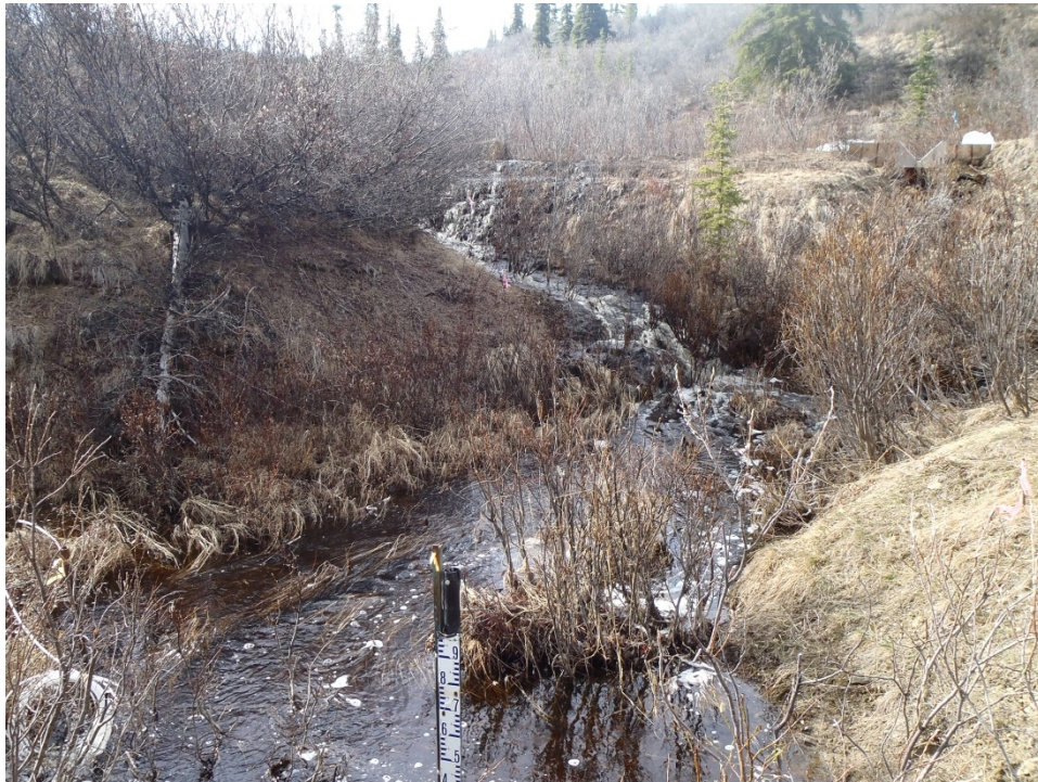
Photo 9. H-PC-U station looking upstream. Note the additional channels diverting around the weir installation.
