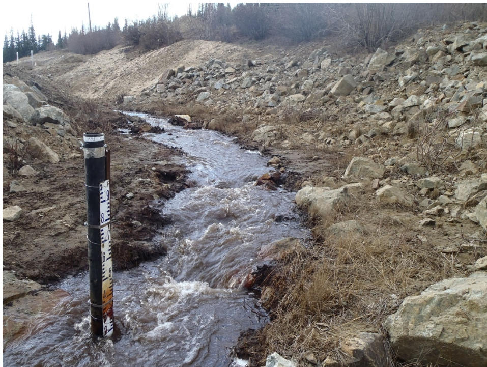
Photo 12. H-DCB station installation looking upstream.
