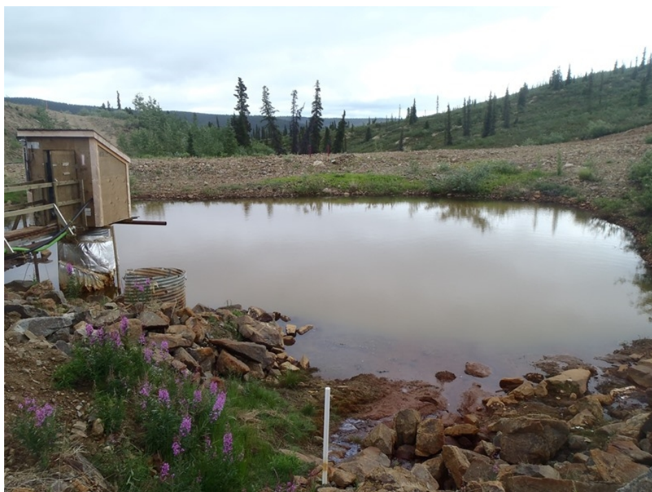
Photo 5. The WQ-SP sampling location showing conditions on seepage pond.
