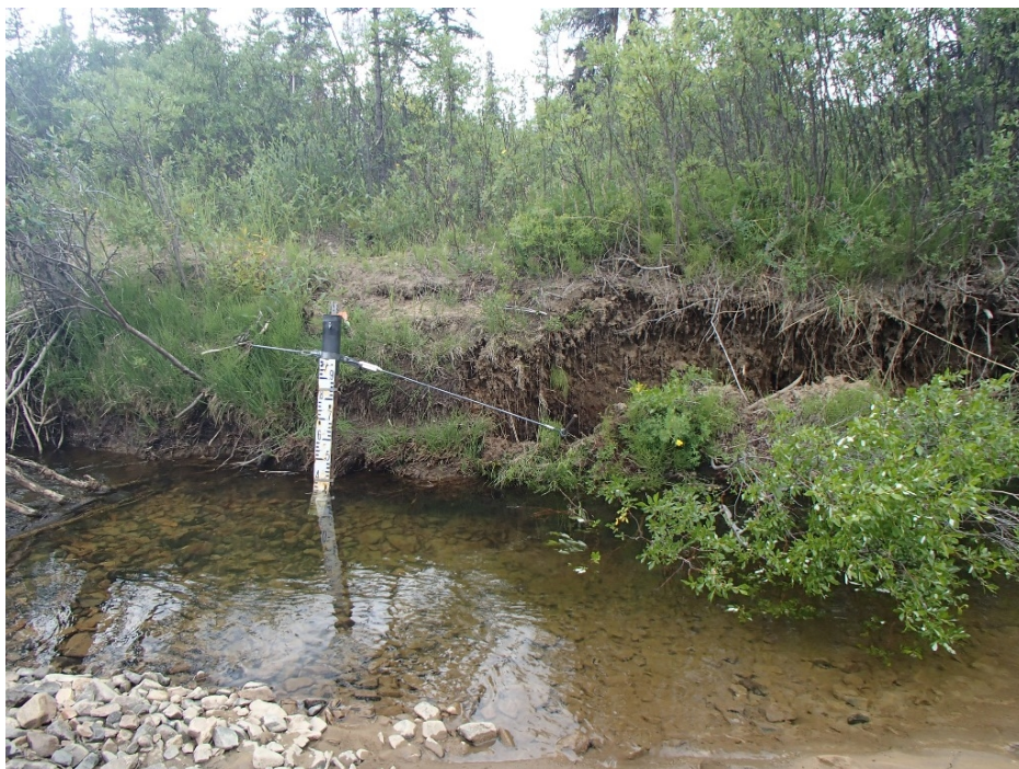
Photo 2. The H-VC-REF station, showing eroding bank and compromised well brace.
