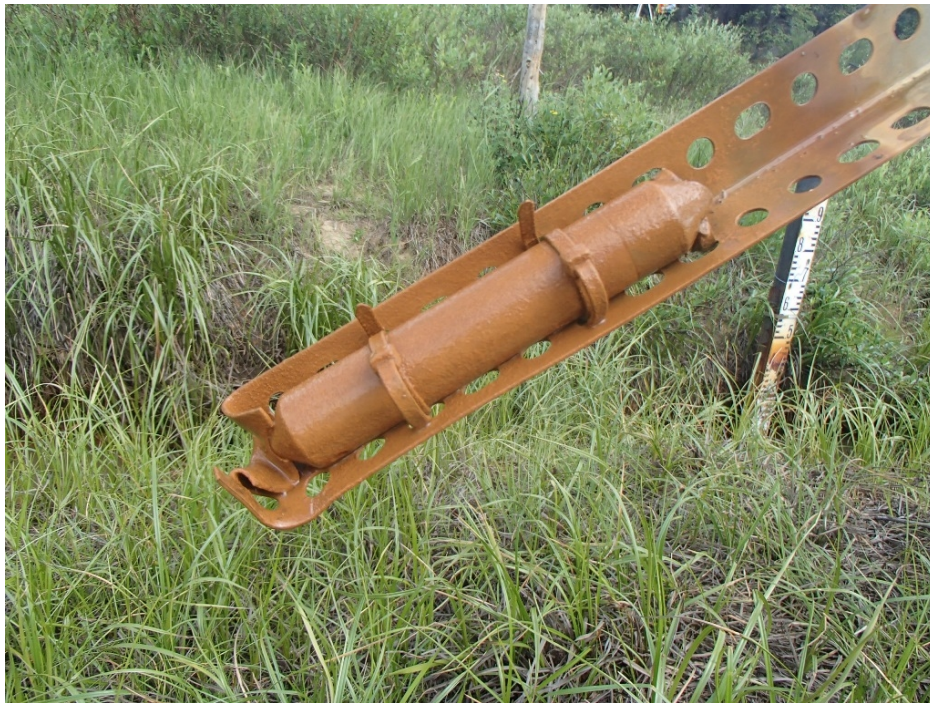
Photo 1. H-DC-R logger submerged in silt, well sedimentation detected.
