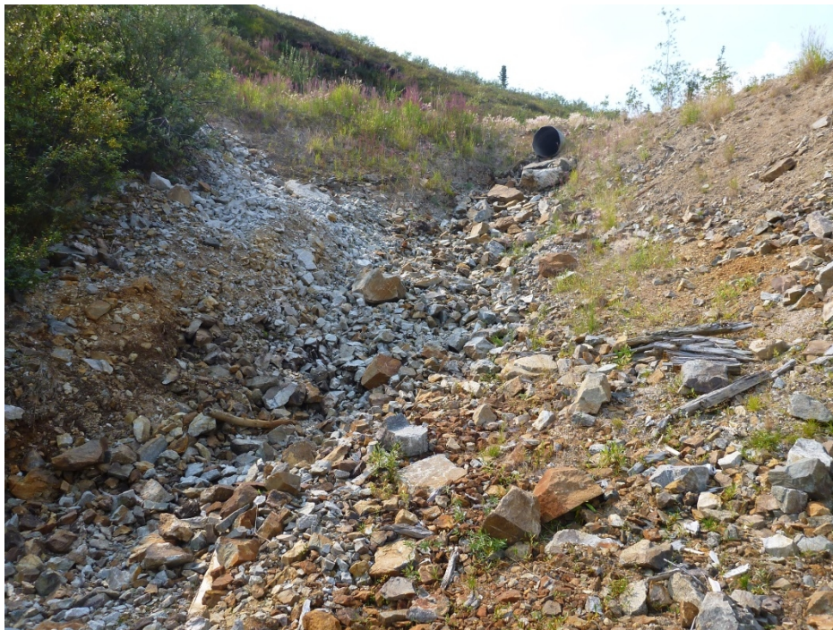
Photo 7. WQ-Adit Seep site showing no surface flow.
