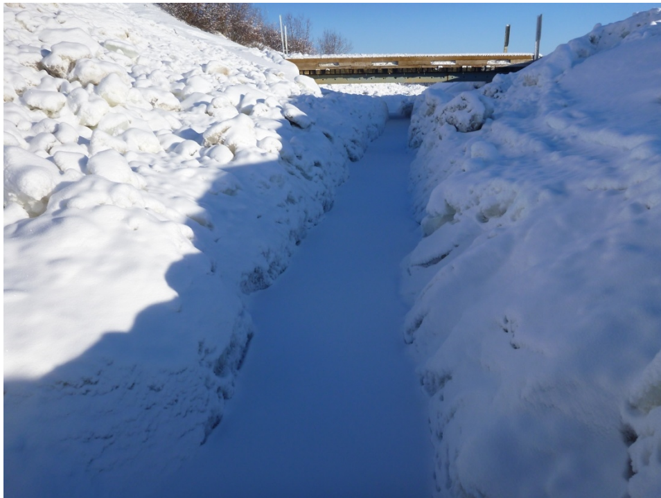
Photo 1. H-DC-B channel. Flow observed beneath and between layers of ice preventing discharge measurement or water quality sample.
