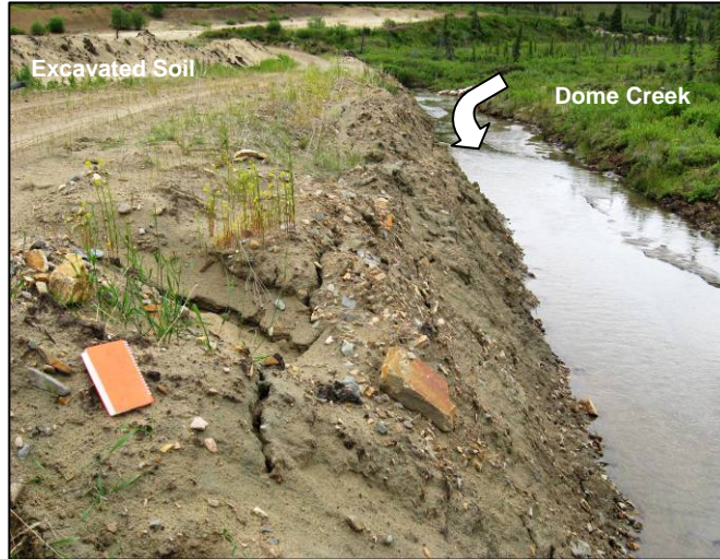
Figure 34 View U/S at Confluence With Dome Cr
