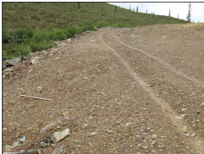
Figure 13 View S at Stabilizing berm from WP 22
