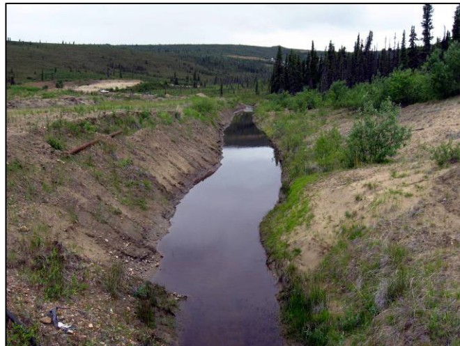
Figure 36 View U/S From Sta 0+620 (WP 67)
