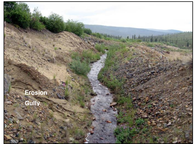
Figure 39 View D/S from Bridge
