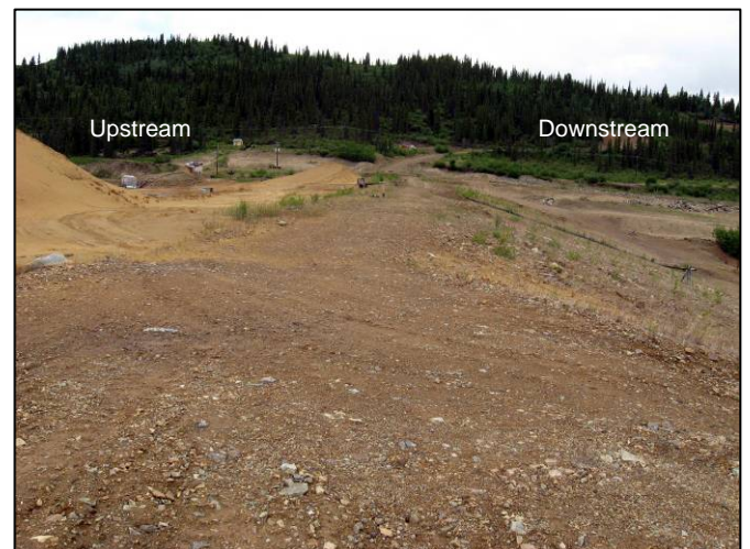
Figure 10 View N at Main Dam From S Abutment
