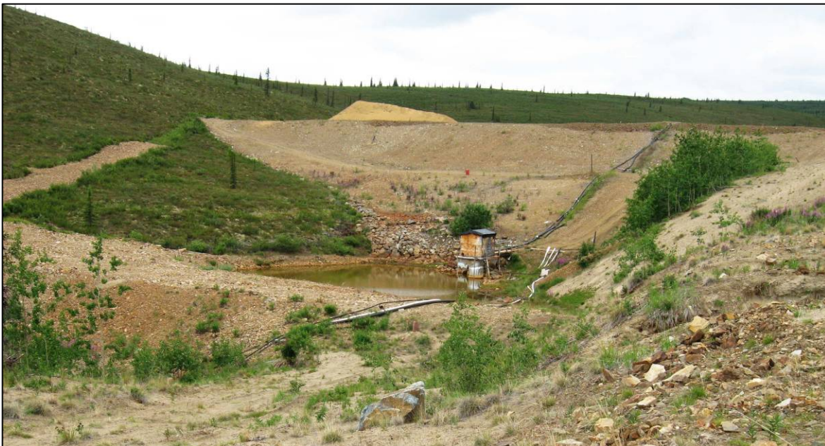
Figure 24 View W at Seepage Pond and Tailings Dam
