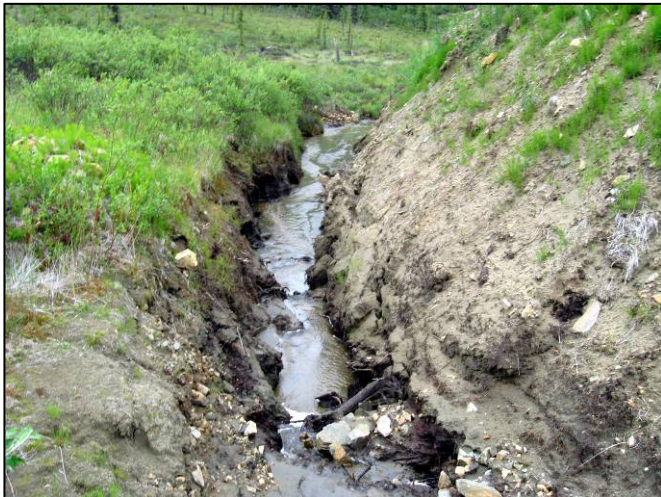
Figure 32 View D/S Along Ditch From Sta 0+285
