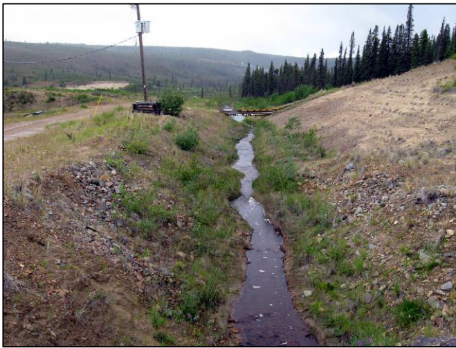
Figure 38 View U/S from Bridge
