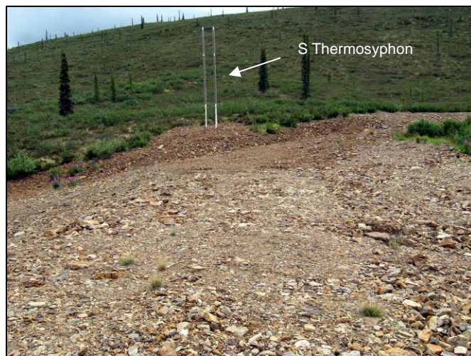
Figure 20 View S Along Seepage Dyke Crest
