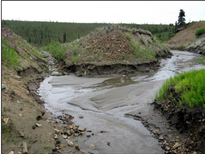
Figure 30 View U/S at Secondary Ditch at Sta 0+280
