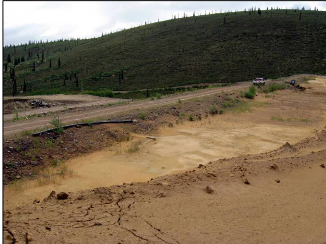
Figure 11 View SE at Main Dam Upstream Slope
