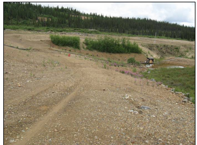
Figure 14 View N at Stabilizing berm from WP 22
