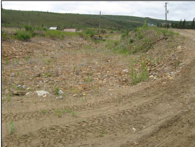
Figure 50 Channel U/S of Road Crossing
