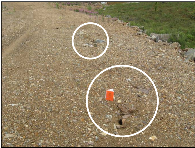
Figure 16 Spreading of Fill at WP 22 (View N)
