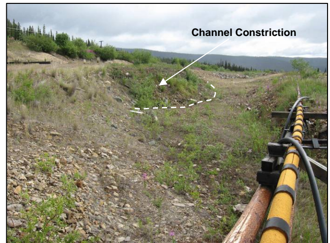
Figure 49 Spillway at Discharge Line Crossing
