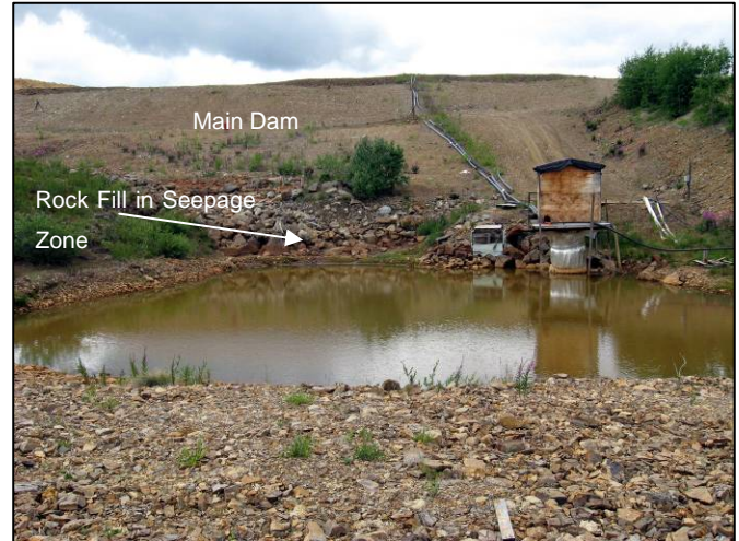
Figure 19 View W over Seepage Pond From Dyke
