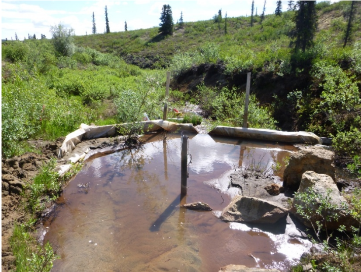
Photo 9. H-DC-M WP, looking downstream showing sediment excavated from weir pond (June 16, 2015).
