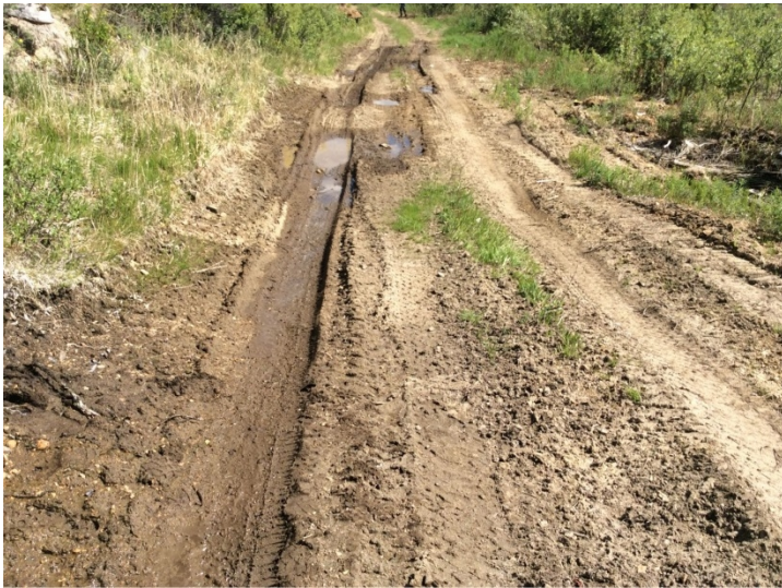
Photo 15. WQ-DESS-02, dry conditions (June 16, 2015).
