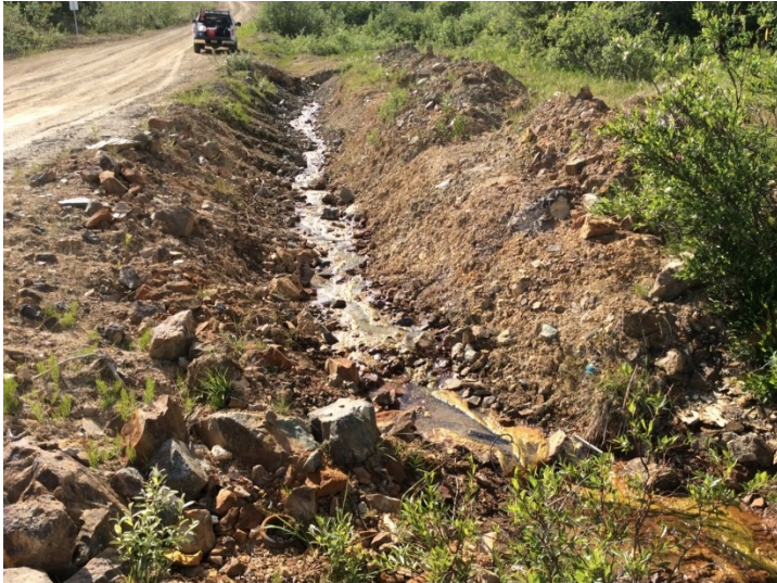
Photo 5. WQ-MS-S-03, looking upstream (June 16, 2015).
