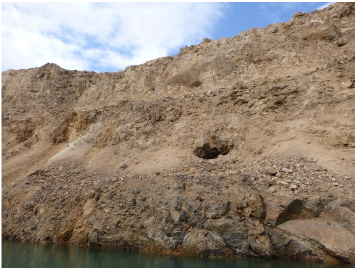
Photo 33. Pit Lake, west pit wall showing potentially unstable rocks above normal sampling location (June 17, 2015).
