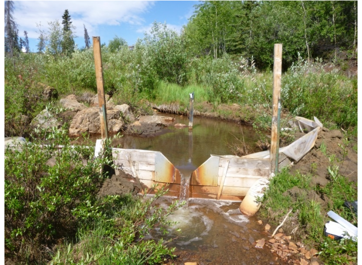
Photo 10. H-DC-M WP, looking upstream (June 16, 2015).
