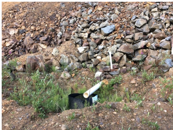
Photo 21. WQ-NW-SEEP-02 – overview of site. Pipe outlet dry.
