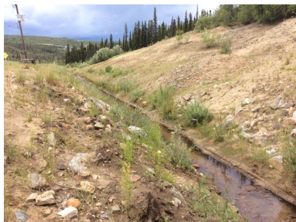
Photo 6. WQ-DC-B – looking upstream.
