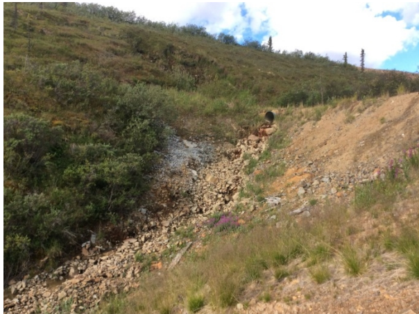
Photo 18. WQ-ADIT-SEEP – looking upstream.
