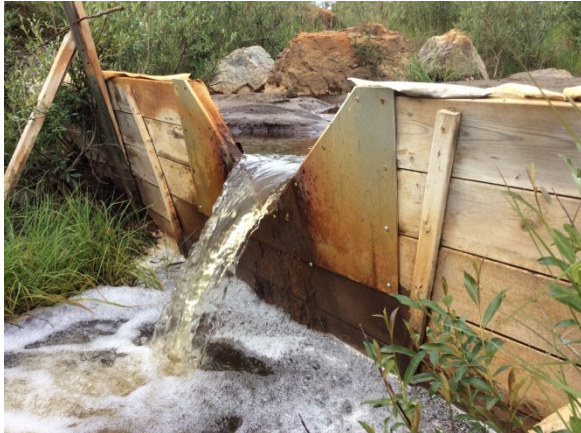
Photo 13. H-DC-M WP – overview of V-notch weir plate.
