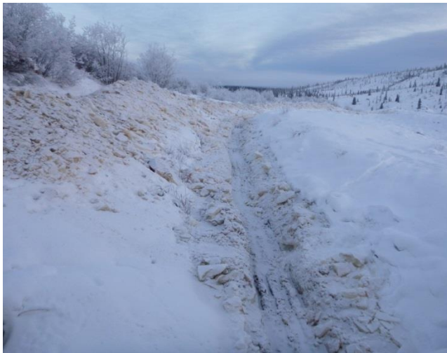
Photo 3. Recently dredged diversion channel downstream of H-DC-B (January 1, 2015).
