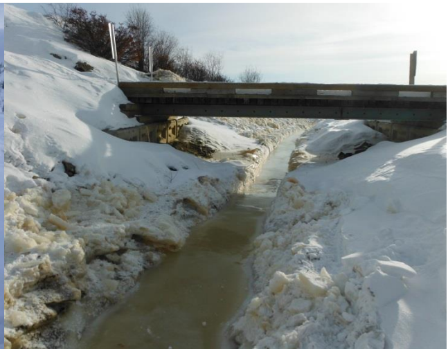
Photo 4. WQ-DC-B, looking downstream (March 17, 2015).
