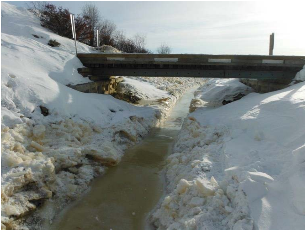
Figure 3-40: DC-B, looking downstream (March 17, 2015). Source: EDI 2015a.
