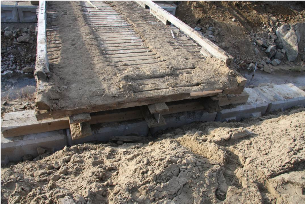
Photo 6 (opposite side of the diversion channel)
