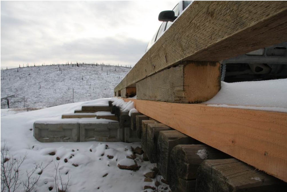
5.) Rails were replaced with new 6 x 6's. (Next 2 pics)
