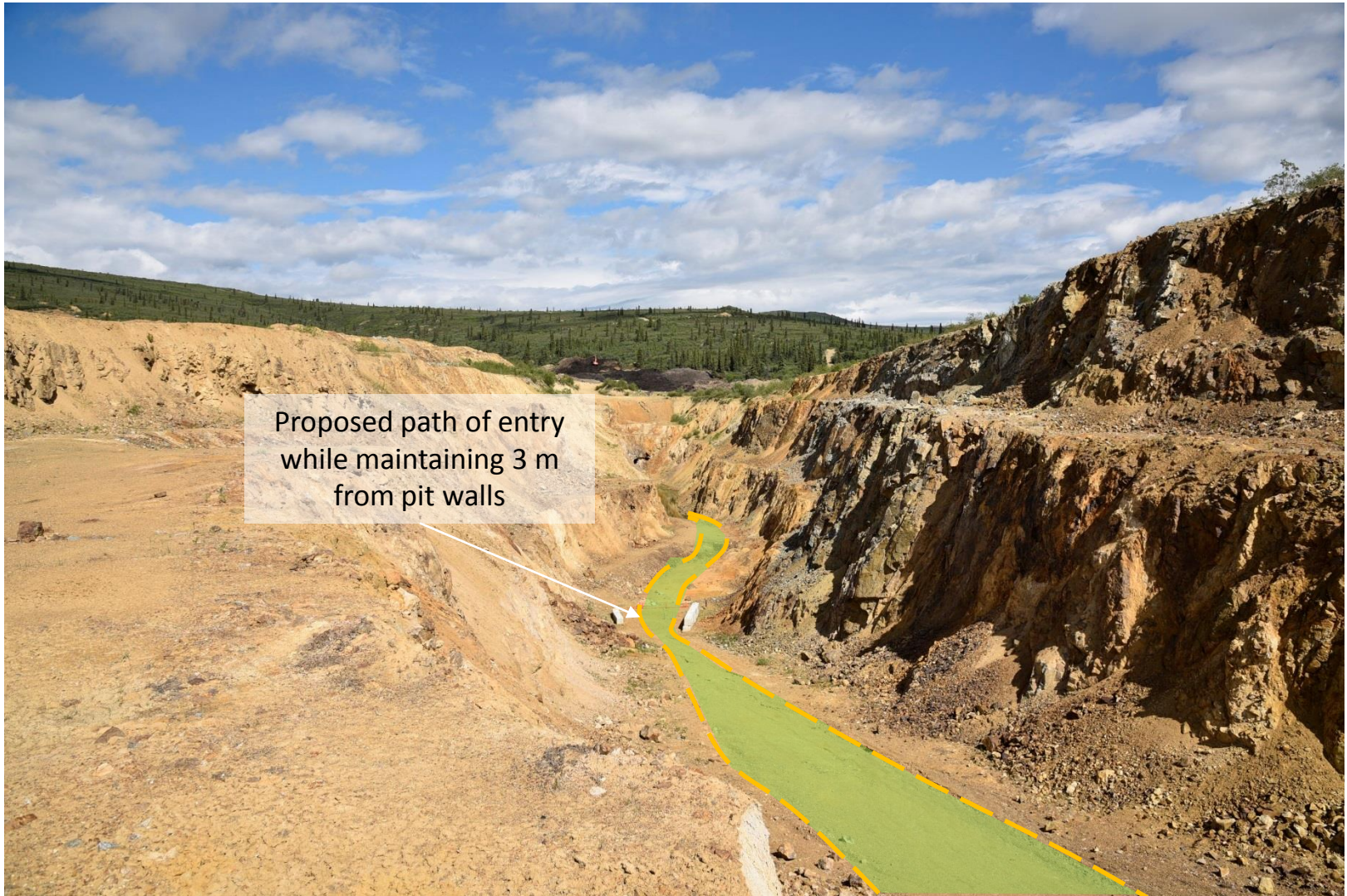
Photo 9: Overview of entry path that should be taken into the pit. Personnel should not come within 3 m of pit walls. Photo taken June 23, 2016
