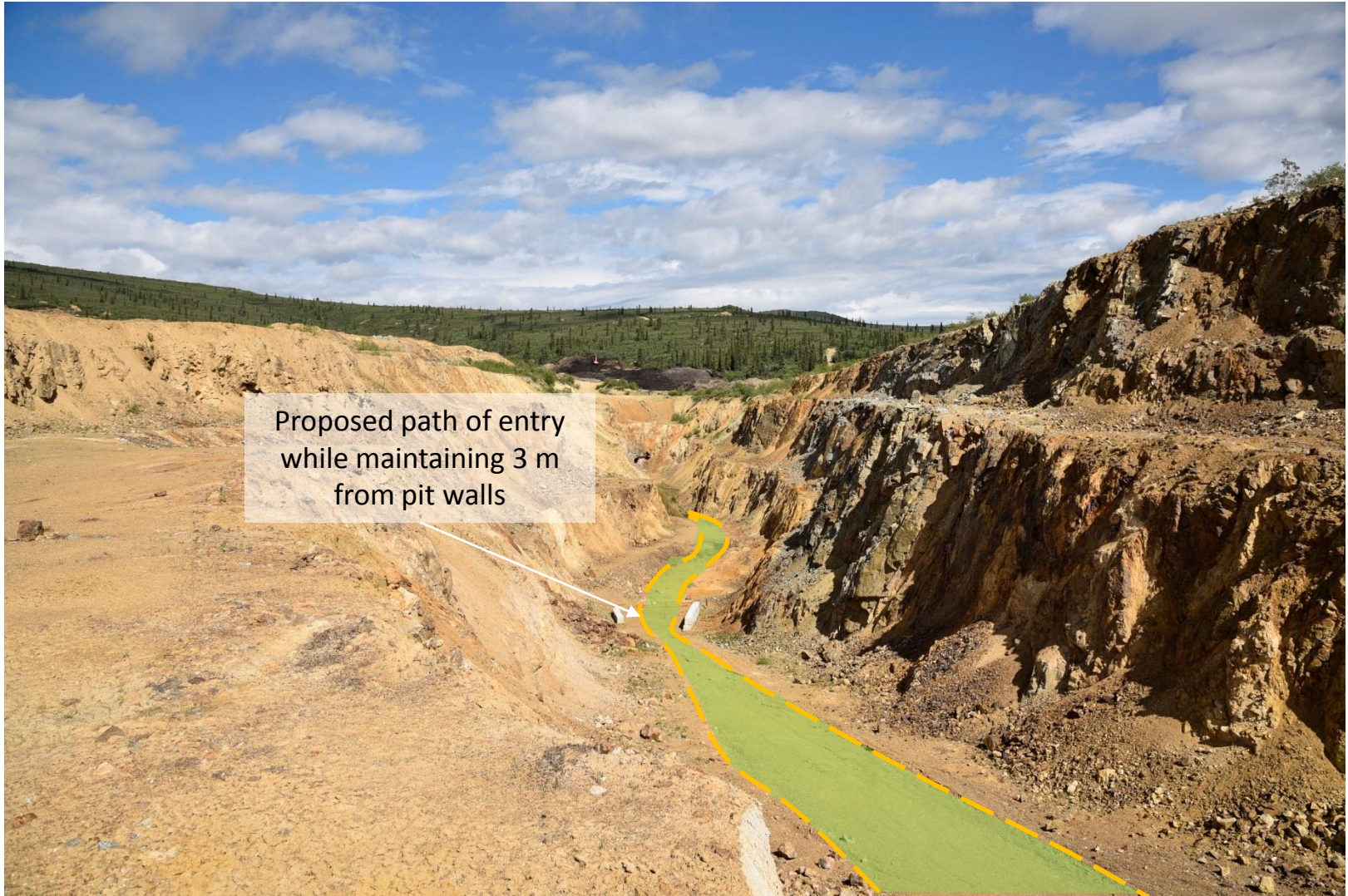
Photo 1: Overview of entry path that should be taken into the pit. Personnel should not come within 3 m of pit walls. Photo taken June 23, 2016
