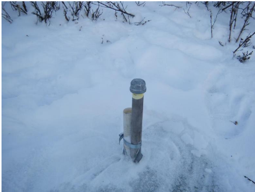
Photo 14. Second piezometer at site CH13-107-PZ011, November 13, 2013.
