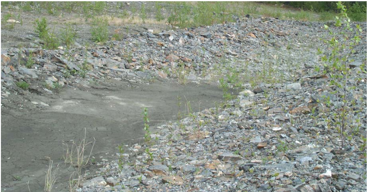
Photo 4: View of the collection drain at the toe of the till cover. Note the accumulated fines that have been washed off the slope
