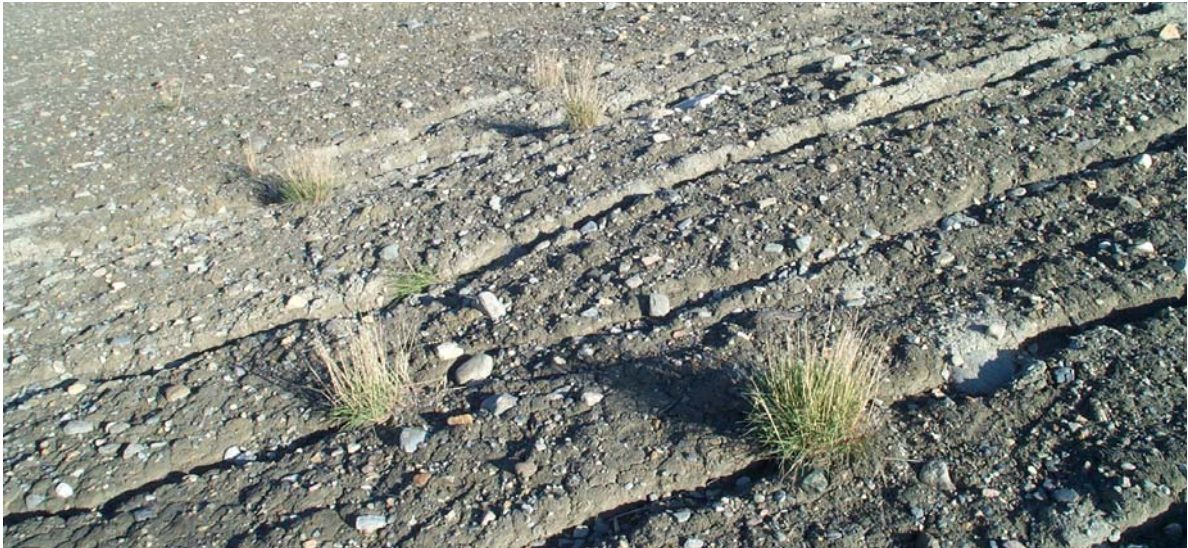
Photo 5: Sparse natural vegetation starting to establish in the erosion gullies on the 10 year old Vangorda waste rock pile till cover.
