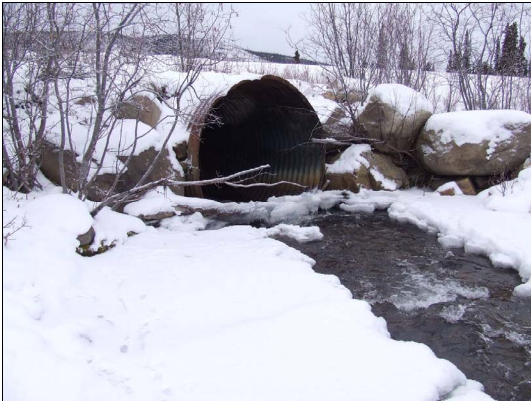
GCULV looking downstream to the culvert on the Mine Access Road, October 27, 2011.
