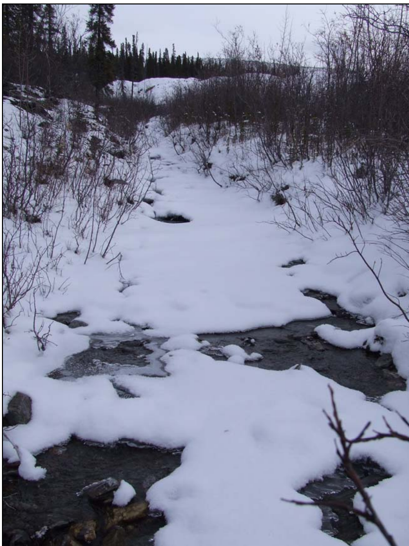
NWID, Northwest Inceptor Ditch looking upstream.
