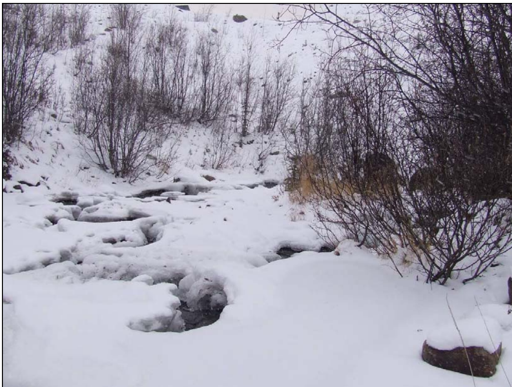
USFR looking downstream to the culverts through the Haul Road, October 26 th , 2011.
