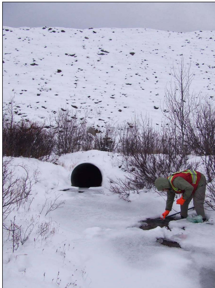
VR looking downstream towards Haul Road, Oct 25 th , 2011.
