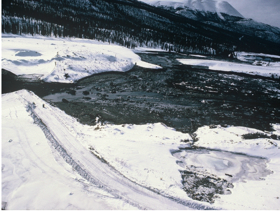
Plate 3. Breach in tailings dam (1975).
