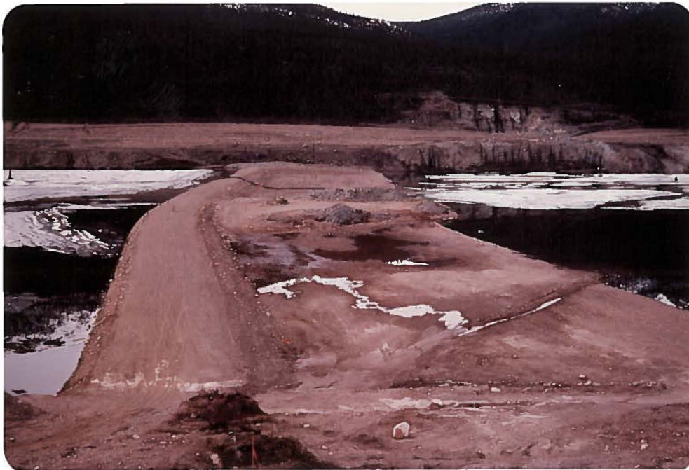
View SSW of Intermediate Dam at full impoundment. Note surface of seepage at downstream toe of embankment from approx. Sta 0+220 to Sta 0+350 (c. 1 June 1982)
