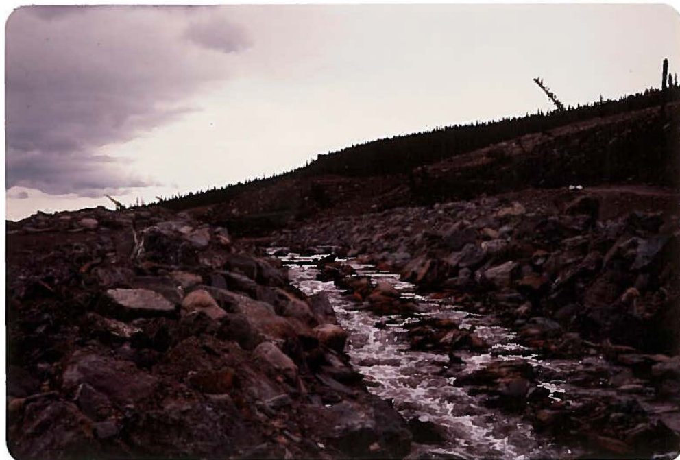
View SE of Intermediate Dam decant functioning at full impoundment.
