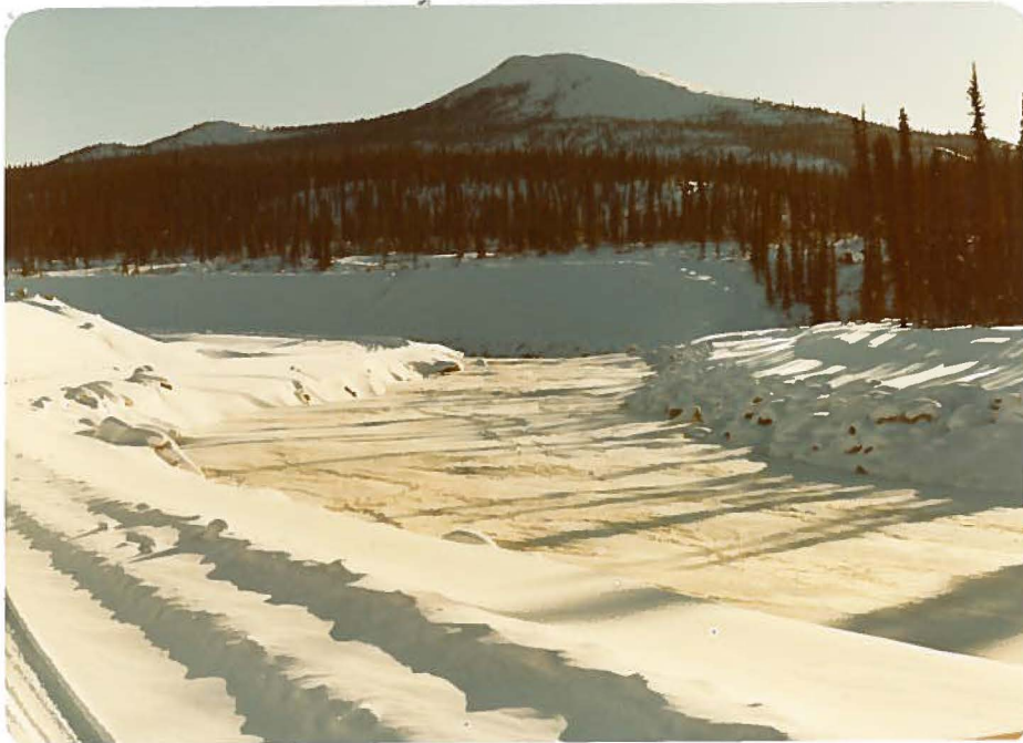
View S From about Sta 3 + 400
