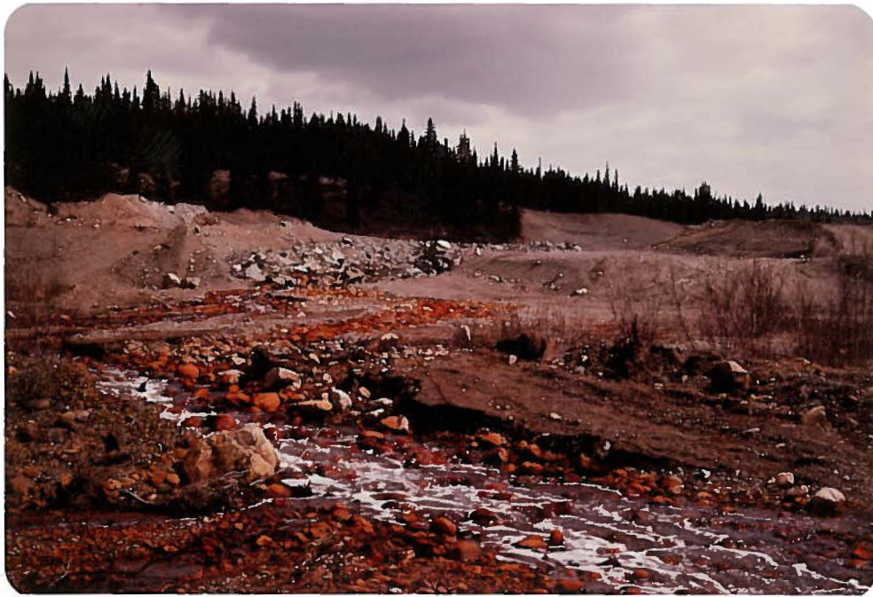
View east from end of decant/spillway (c. 1 June 1982). Note that decant flow over natural materials is not resulting in unacceptable erosion.
