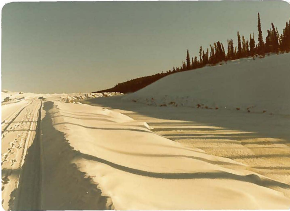
View S.E. from about Sta 3 + 200.
