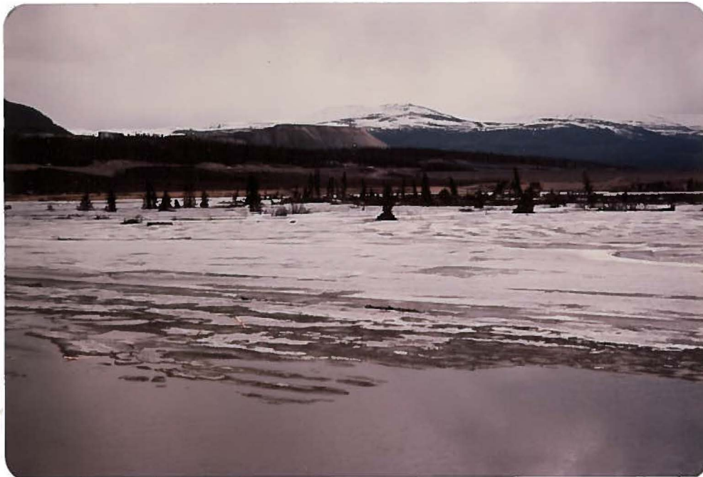
View NE from south abutment Int. Dam showing I.D. reservoir at full impoundment. Note that construction stakes in left foreground and trees have been jacked from the valley bottom by the reservoir ice surface due to winter impoundment.
