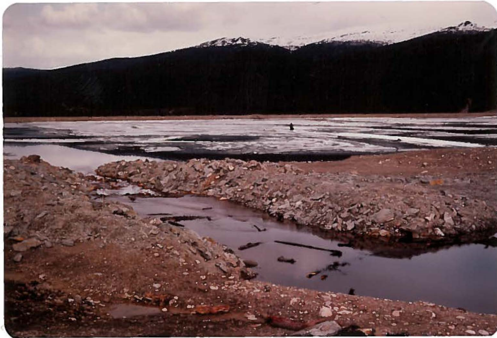
View NW showing Intermediate Dam decant/spillway function at full impoundment. CVD reservoir in the background (c. 1 June 1982)
