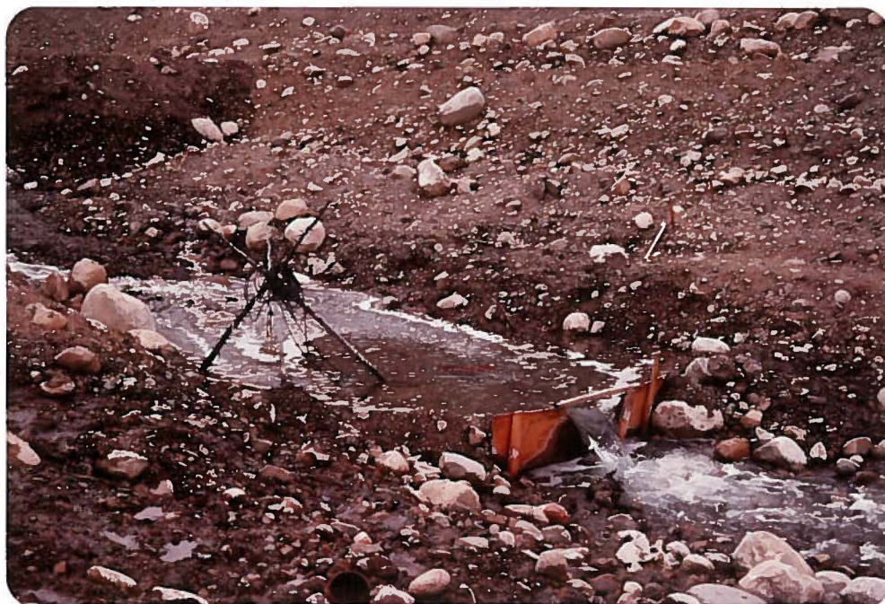
Closeup view of weir No. 1 (1000 i.g.p.m. approx.) showing also observation point for pneumatic piezometers at Sta 0+210.
