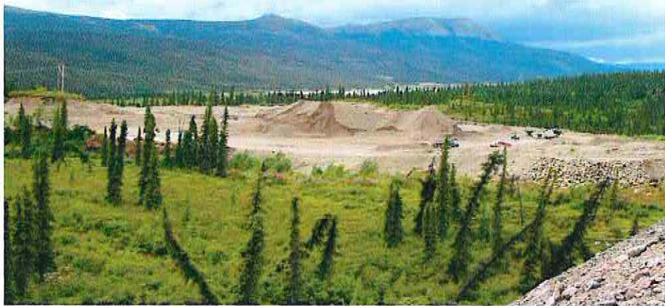
Photo 1: Haul Road Borrow Site
