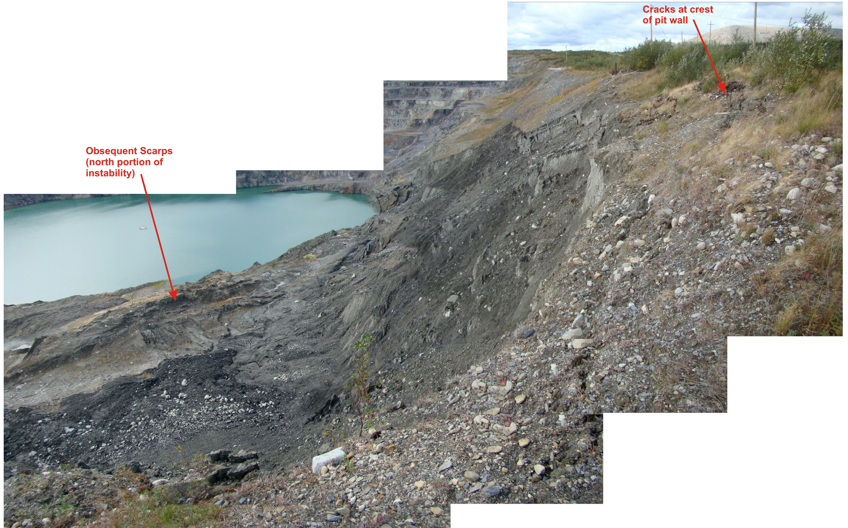
Photograph 7 : Crest of east wall looking north (August, 2009).
