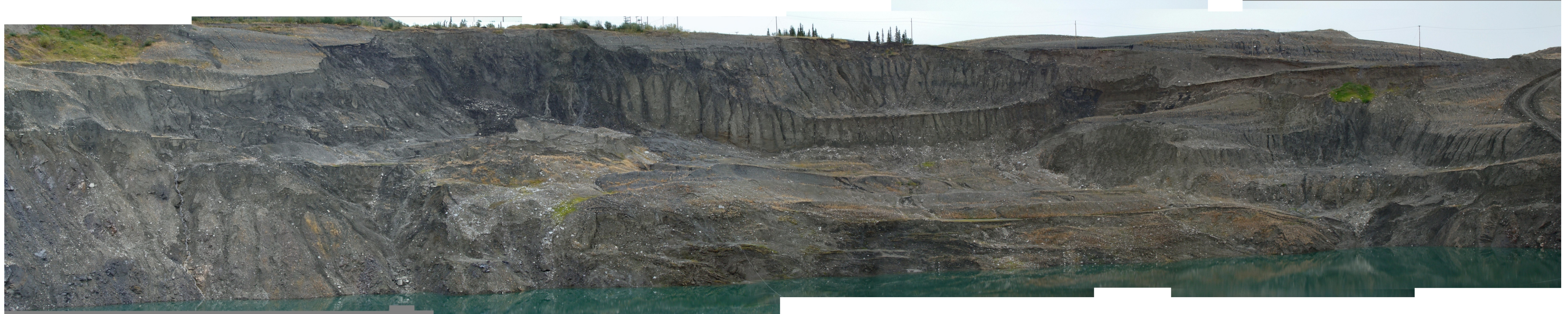
Photograph 3 : East Wall Instability.
