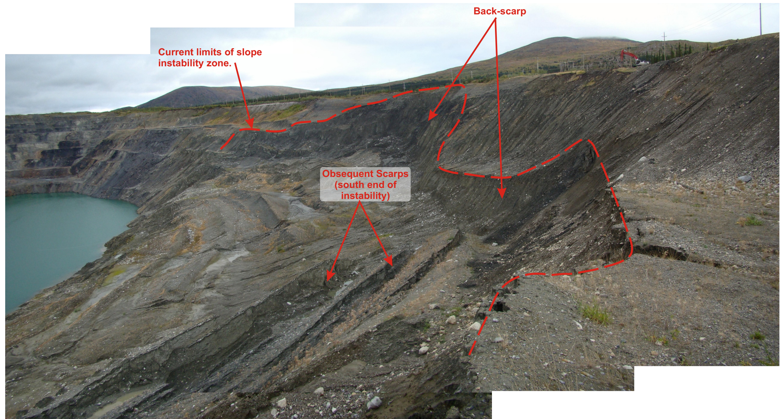
Photograph 5 : East wall instability looking north (August, 2009).
