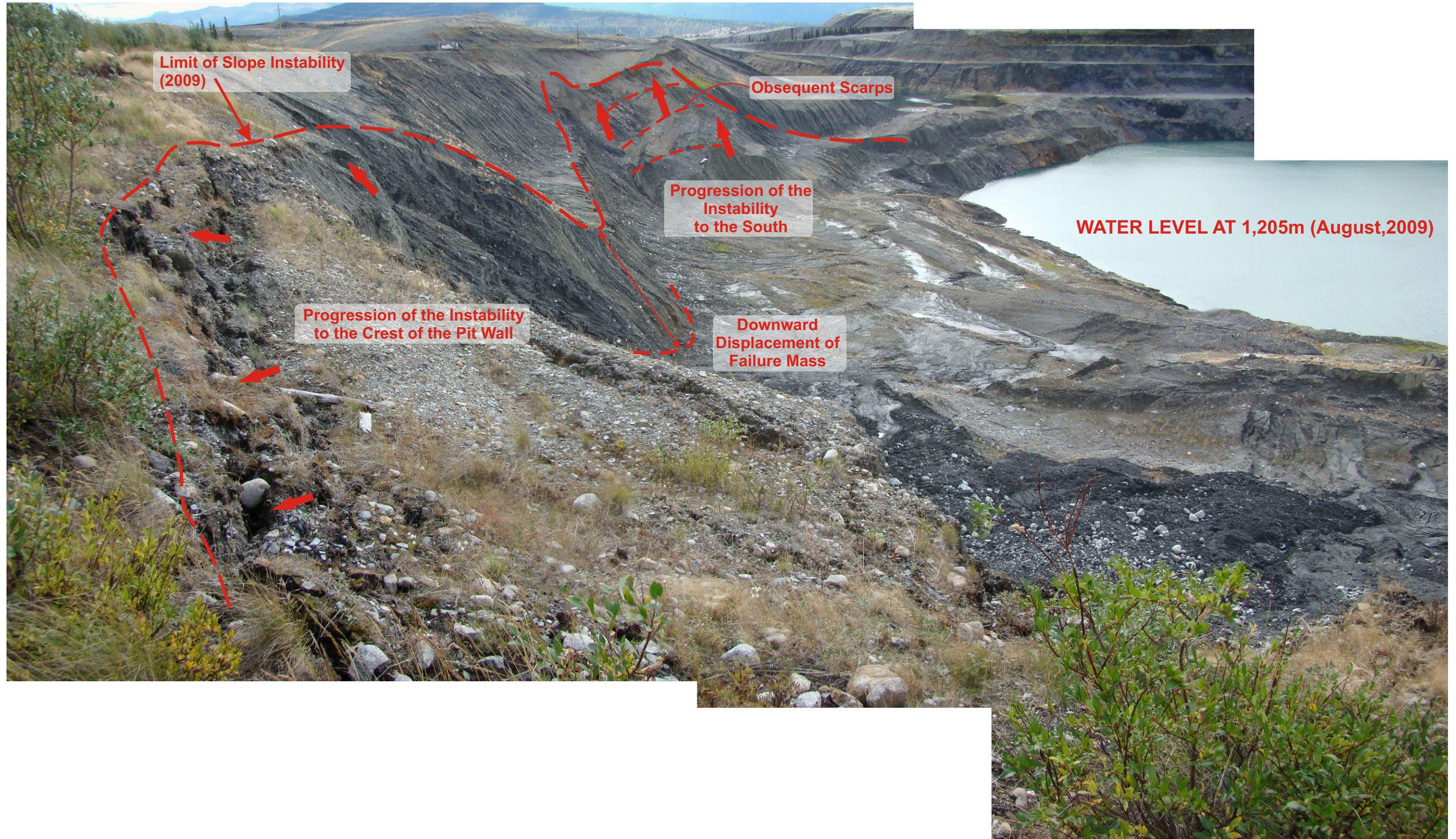
Photograph 8 : East wall instability. Crest of the pit wall looking south (2009).
