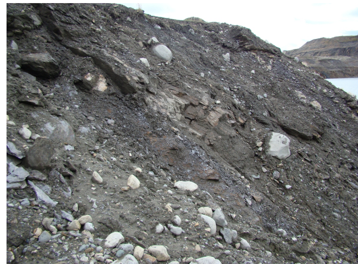
Photograph 16 : Rock exposed on the lower wall at the north limit of instability.
