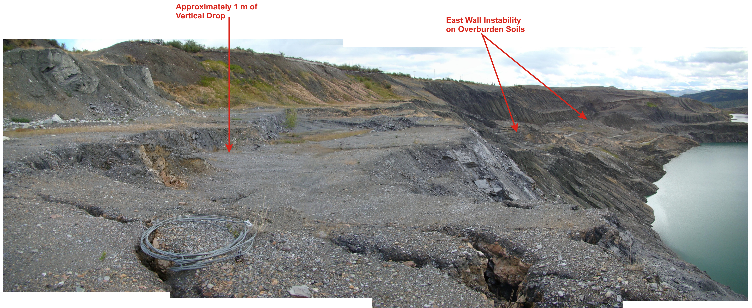
Photograph 12 : Instability on rock slopes in the north portion of the east wall (August, 2009).
