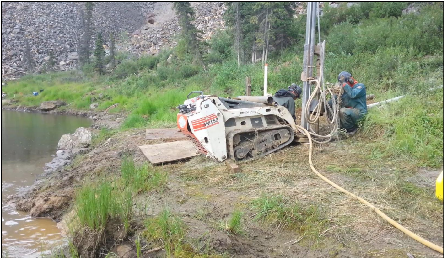
Photo A4: Drilling with ODEX at MW14-12D. Compressed air is fed from an air compressor upslope of the pond area.
