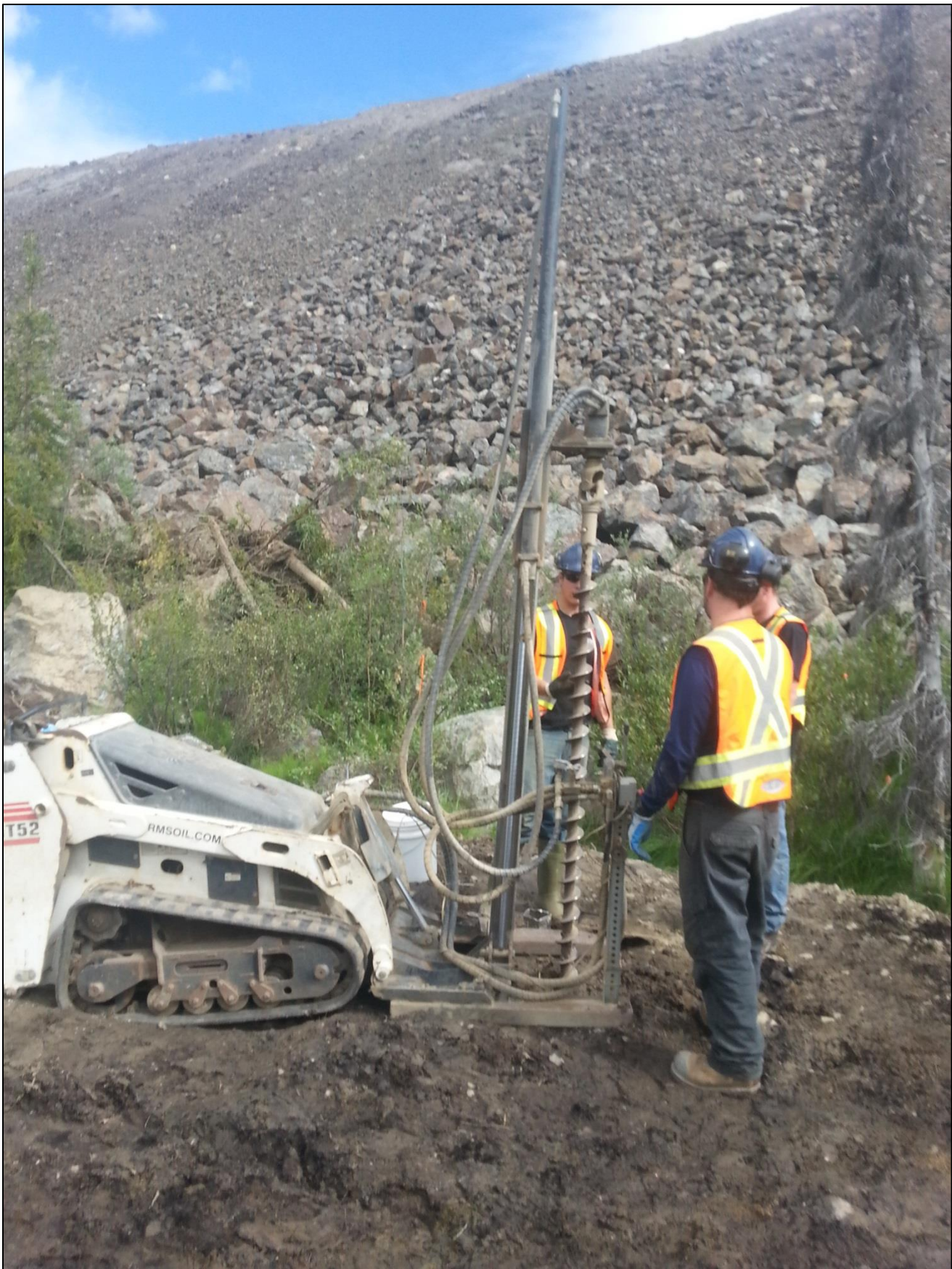
Photo A2: The drill at MW14-08, set up to drill with solid stem auger and preparing to insert the first auger flyte into the ground. The drill is powered with hydraulics from the modified Bobcat.
